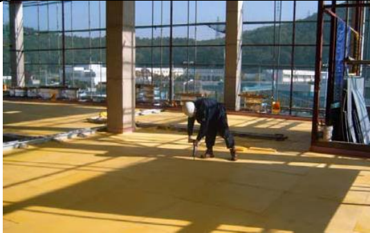
Spread PO-MAT on floor after cleaning
