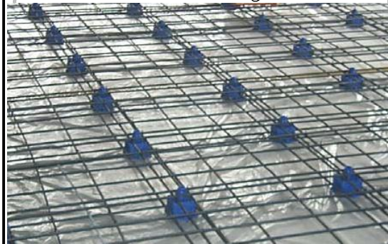
Reinforcing on the Jack-up mount
