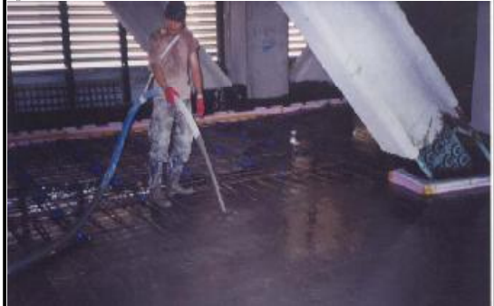
Drying concrete & Lifting floor
