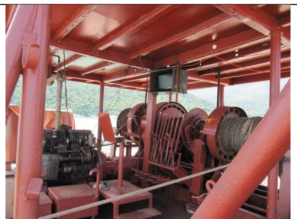
Winch system on vessel board
