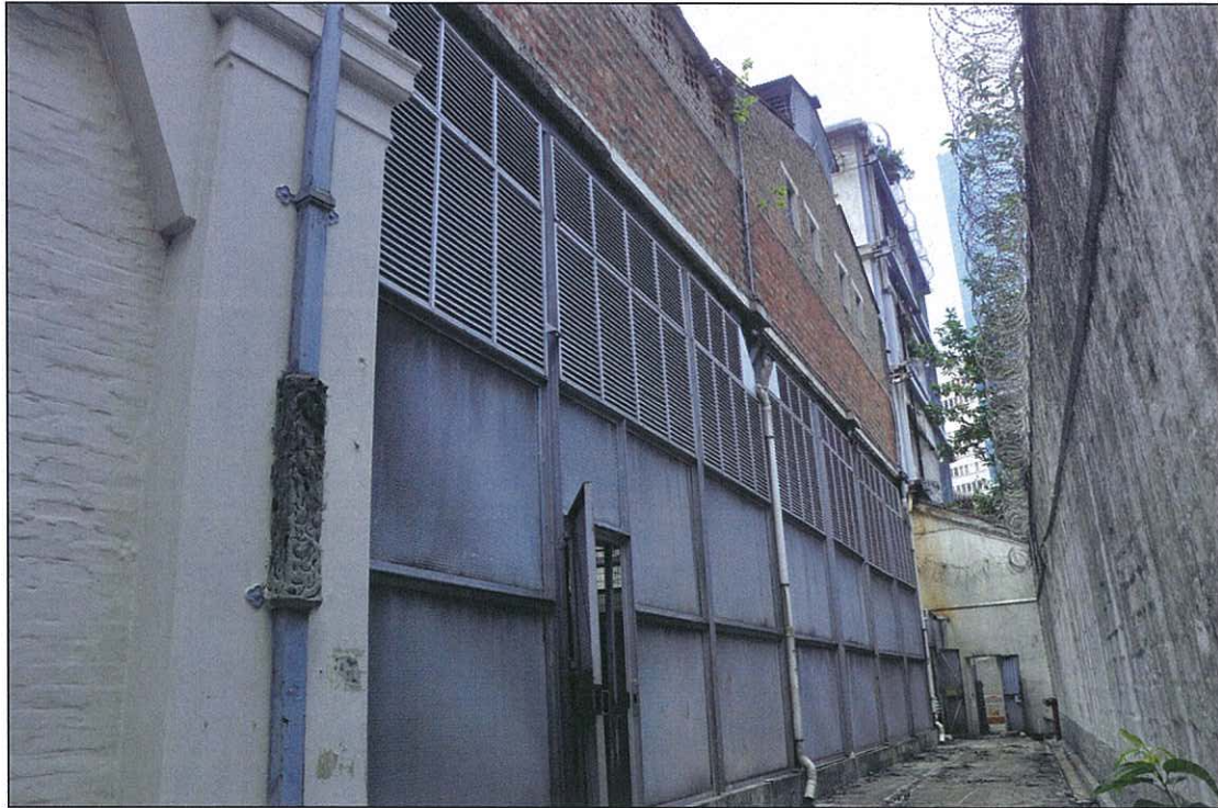
Photo 16.07 – East elevation, lower part (2011/09/07)
