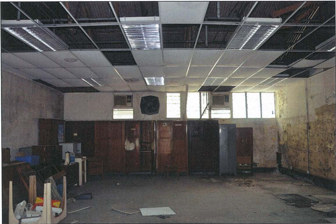
Photo 16.32 – Room G3, interior view (2011/09/07)
