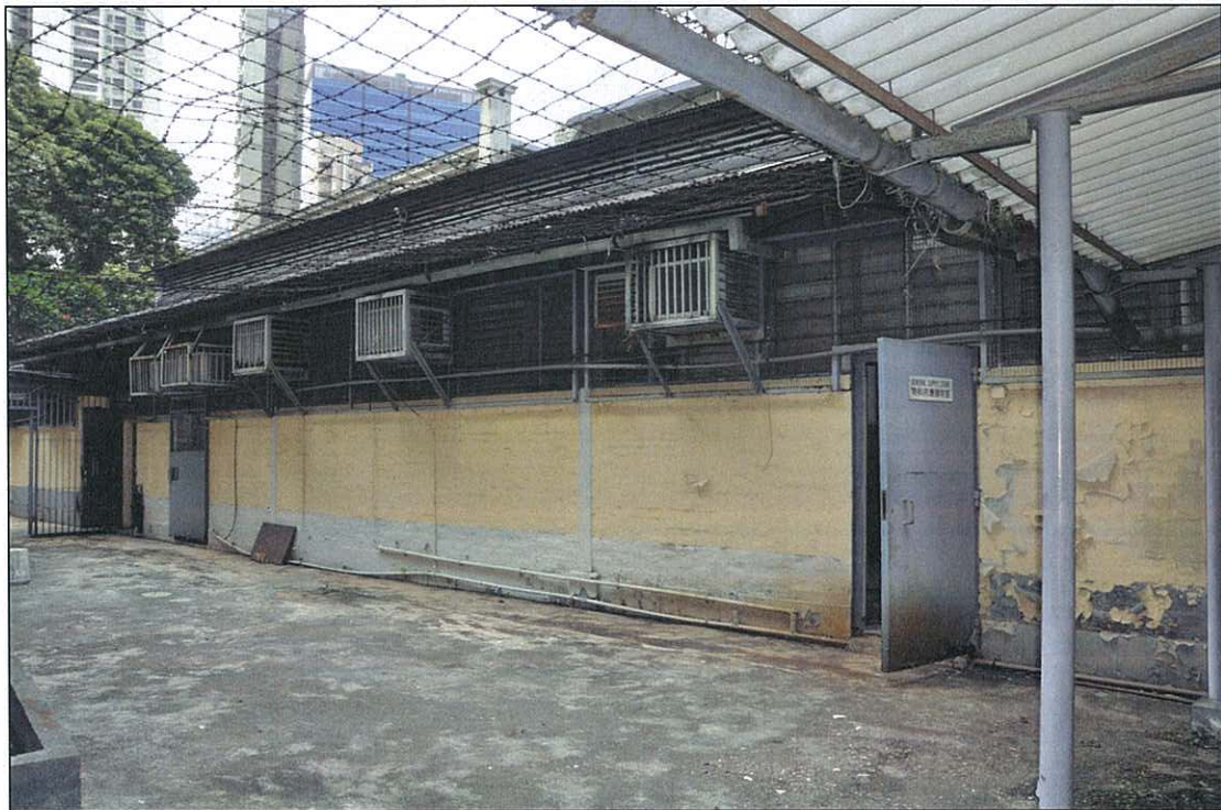
Photo 16.19 – External wall at yard (2011/09/07)
