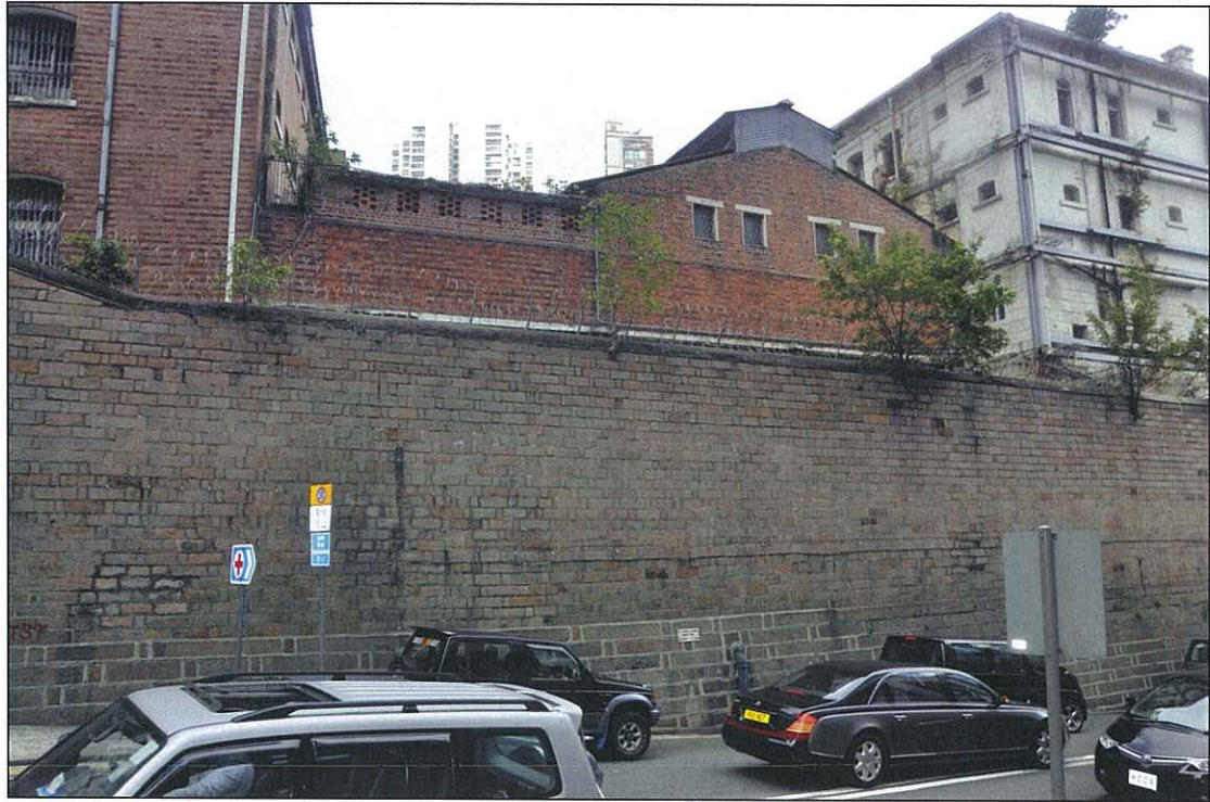
Photo 16.01 – External view from Arbutnot Road (2011/10/06)
