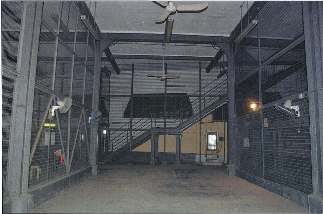
Photo 16.43 – Room LG2, interior view (2011/09/21)
