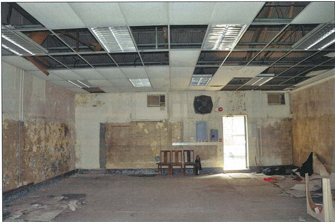
Photo 16.33 – Room G3, interior view (2011/09/07)
