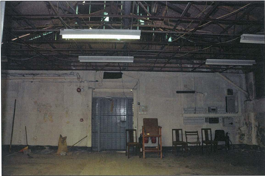
Photo 16.24 – Room G1, interior view (2011/09/07)
