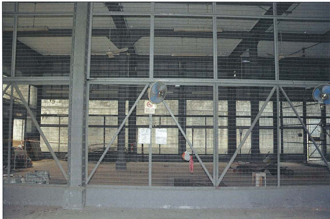
Photo 16.44 – Room LG2, interior view (2011/09/21)
