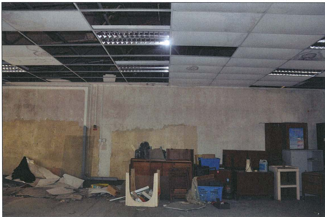
Photo 16.34 – Room G3, interior view (2011/09/07)
