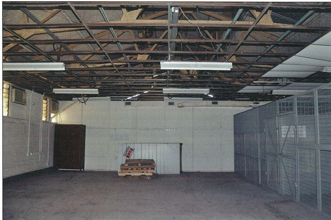
Photo 16.27 – Room G2, interior view (2011/09/07)
