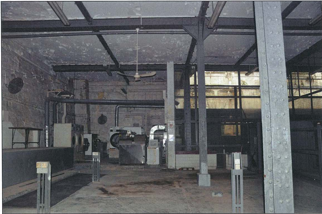
Photo 16.45 – Room LG3, interior view (2011/09/21)
