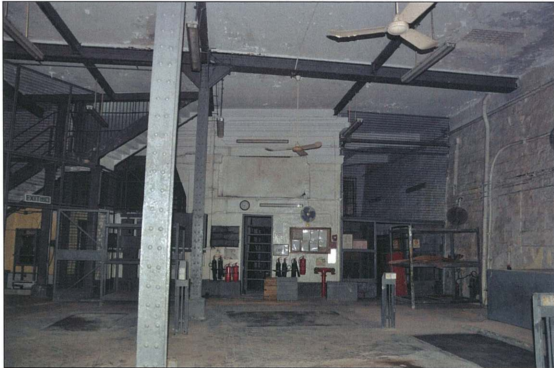
Photo 16.47 – Room LG3, interior view (2011/09/21)
