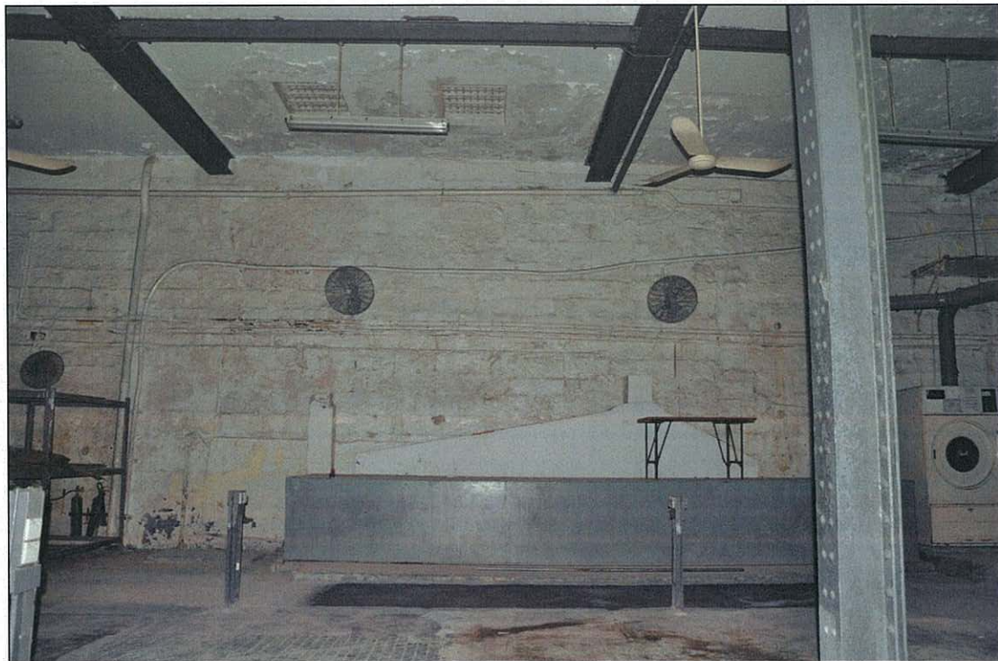
Photo 16.46 – Room LG3, interior view (2011/09/21)
