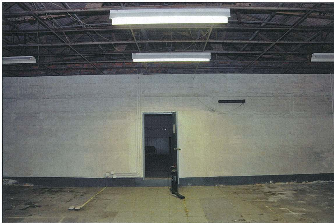
Photo 16.22 – Room G1, interior view (2011/09/07)
