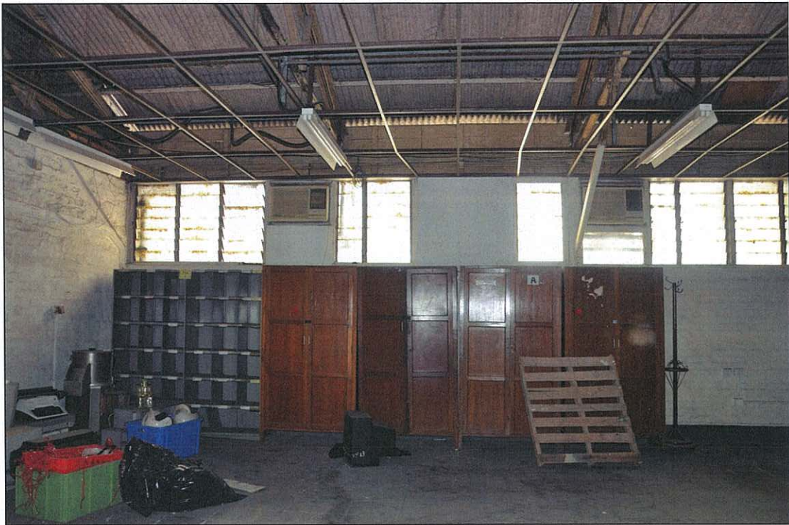
Photo 16.28 – Room G2, interior view (2011/09/07)
