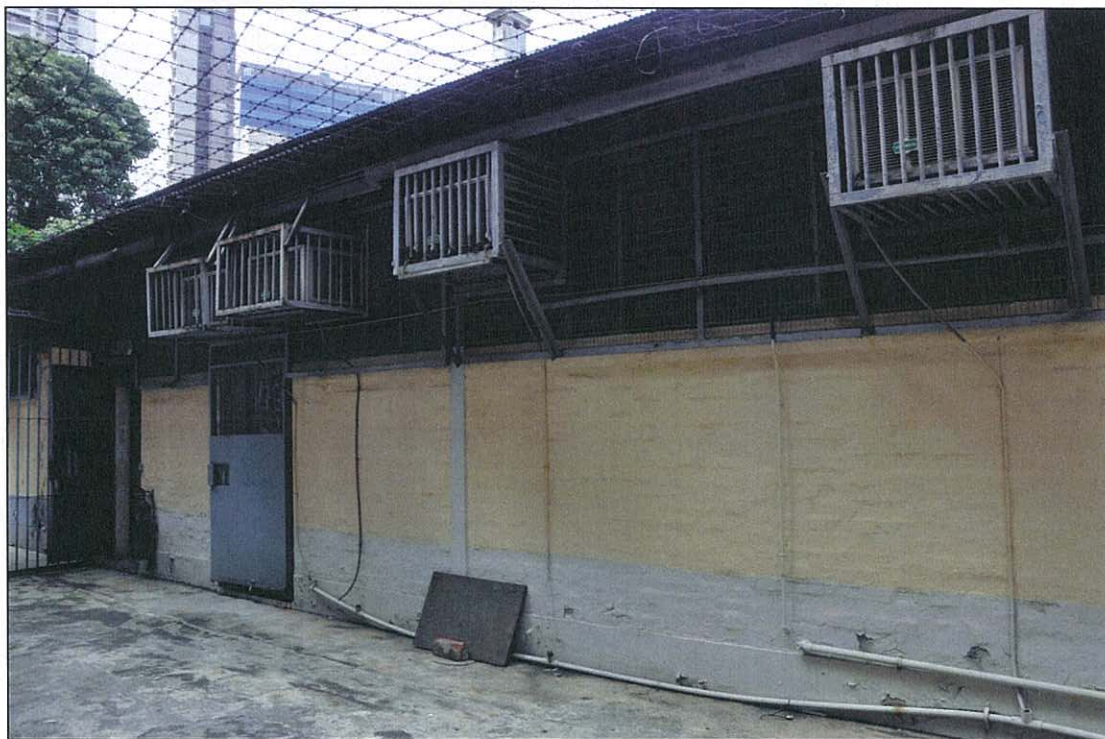
Photo 16.16 – External wall at yard (2011/09/07)
