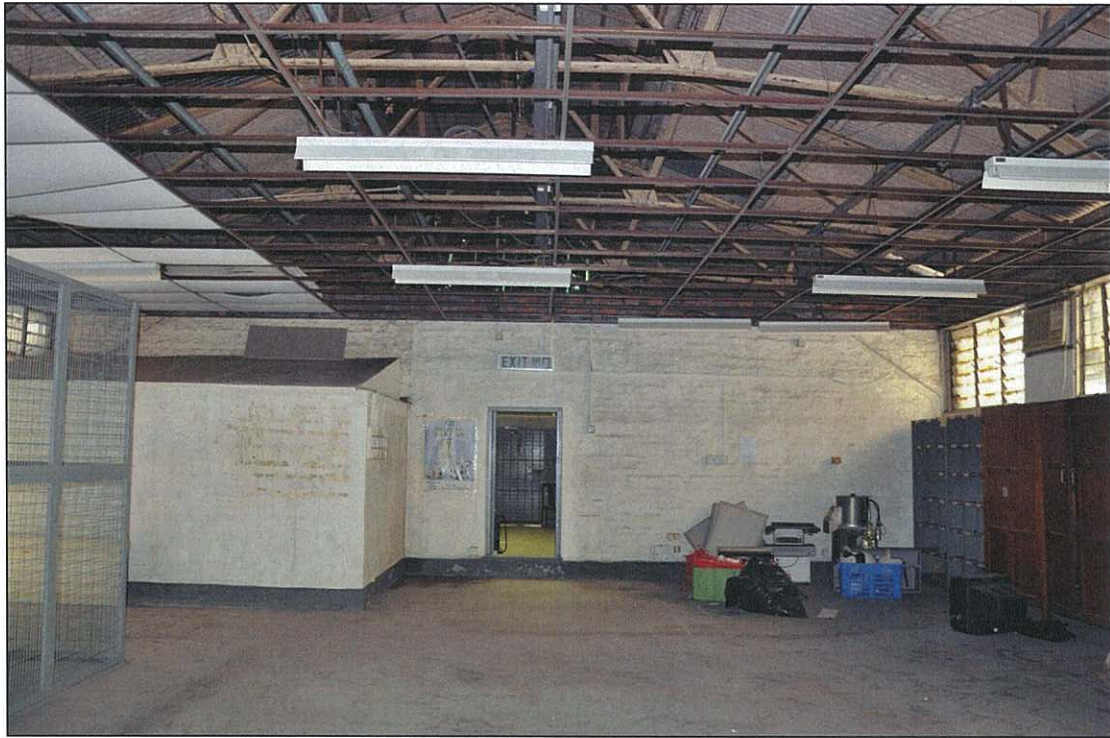
Photo 16.30 – Room G2, interior view (2011/09/07)
