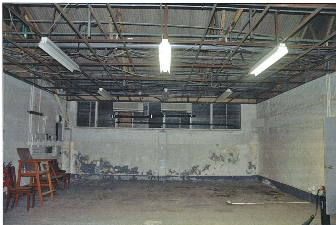
Photo 16.23 – Room G1, interior view (2011/09/07)
