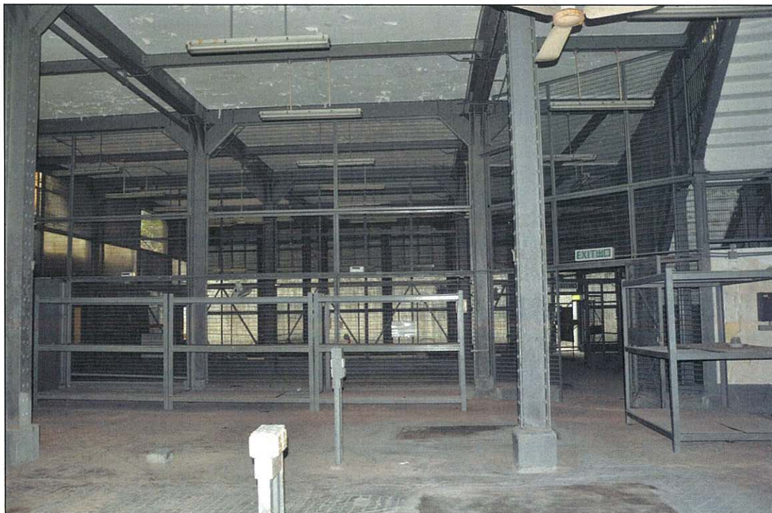
Photo 16.48 – Room LG3, interior view (2011/09/21)
