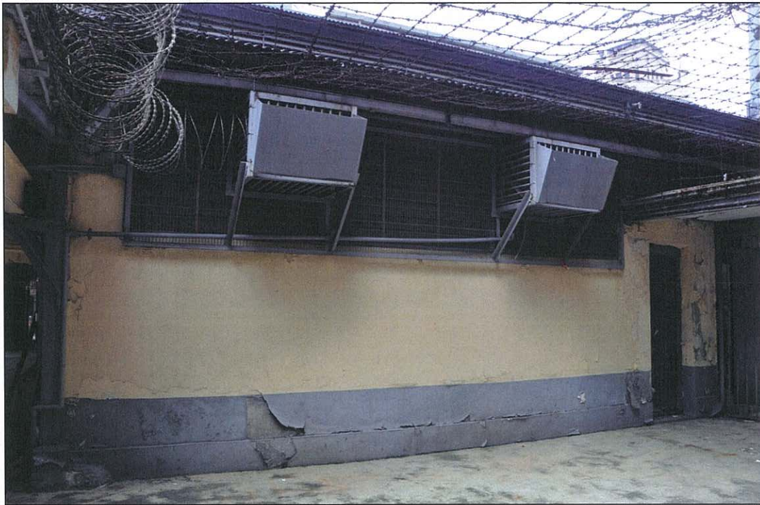
Photo 16.10 – Ground floor, view from yard (2011/09/07)
