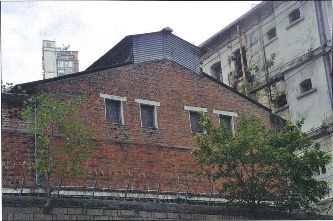
Photo 16.03 – External view from Arbuthnot Road (2011/10/06)
