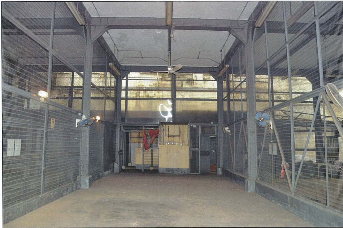
Photo 16.41 – Room LG2, interior view (2011/09/21)
