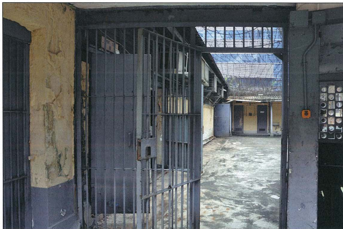
Photo 16.13 – Entrance to yard (2011/09/07)
