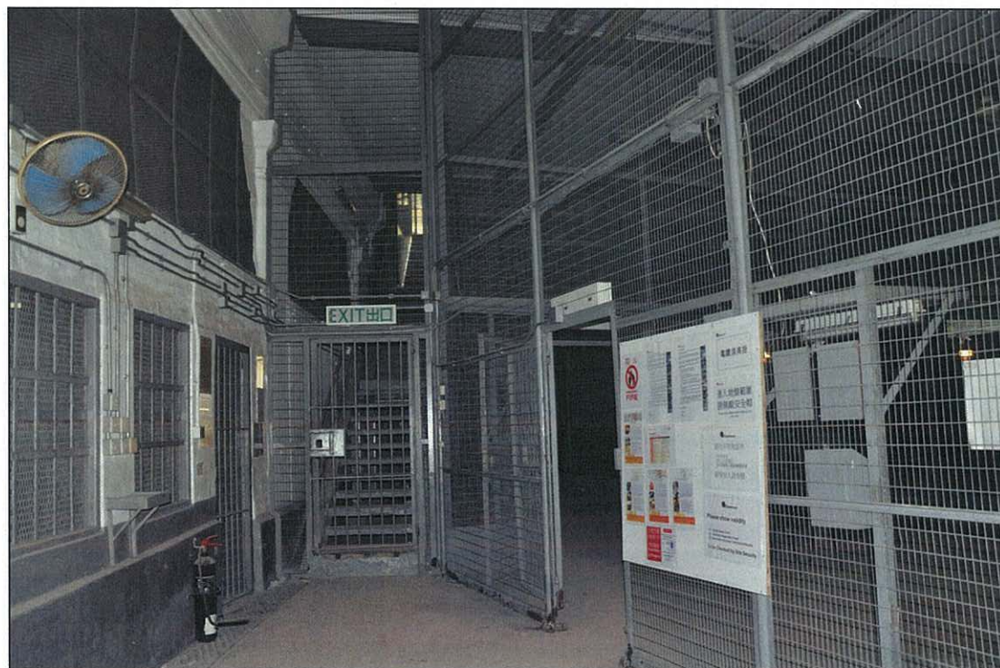
Photo 16.36 – Staircase entrance lobby, interior view (2011/09/21)
