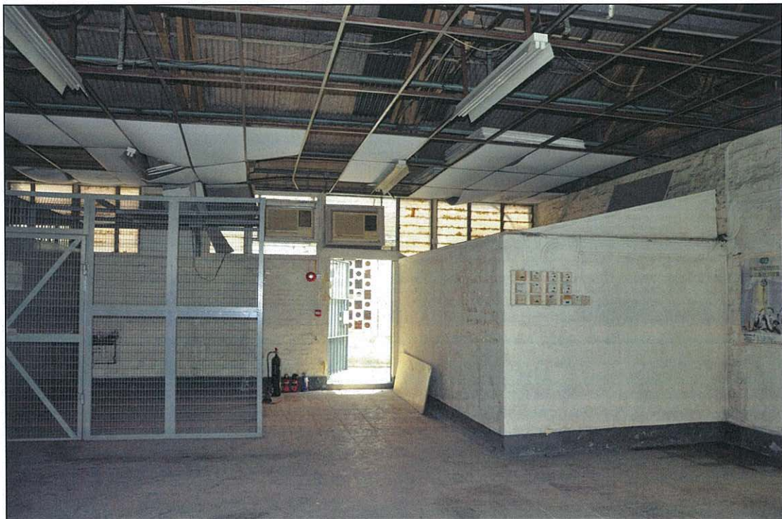
Photo 16.29 – Room G2, interior view (2011/09/07)
