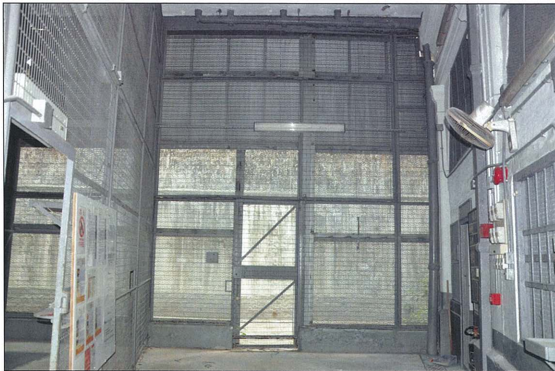
Photo 16.35 – Staircase entrance lobby, interior view (2011/09/21)
