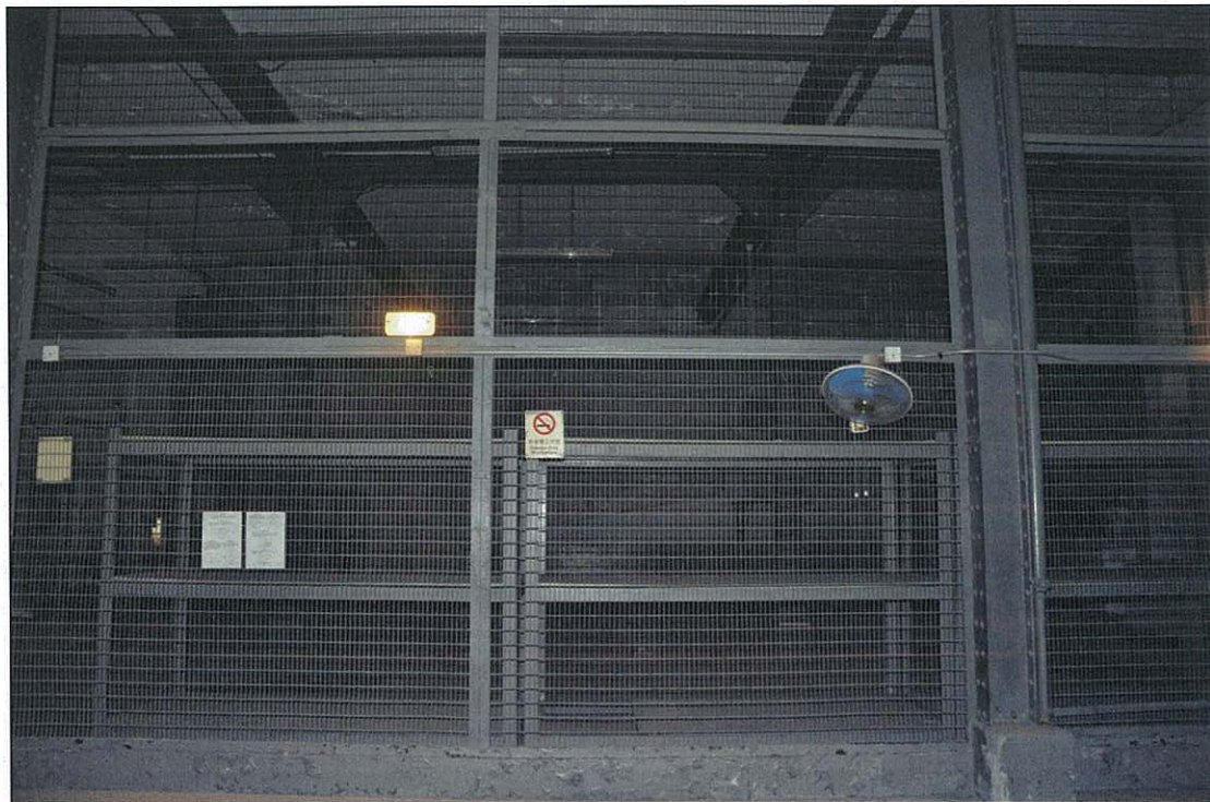
Photo 16.42 – Room LG2, interior view (2011/09/21)
