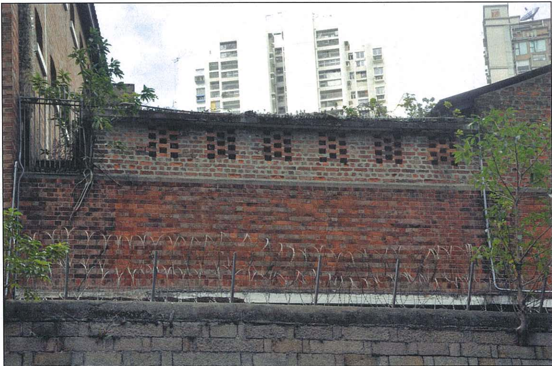
Photo 16.04 – External view from Arbuthnot Road (2011/10/06)
