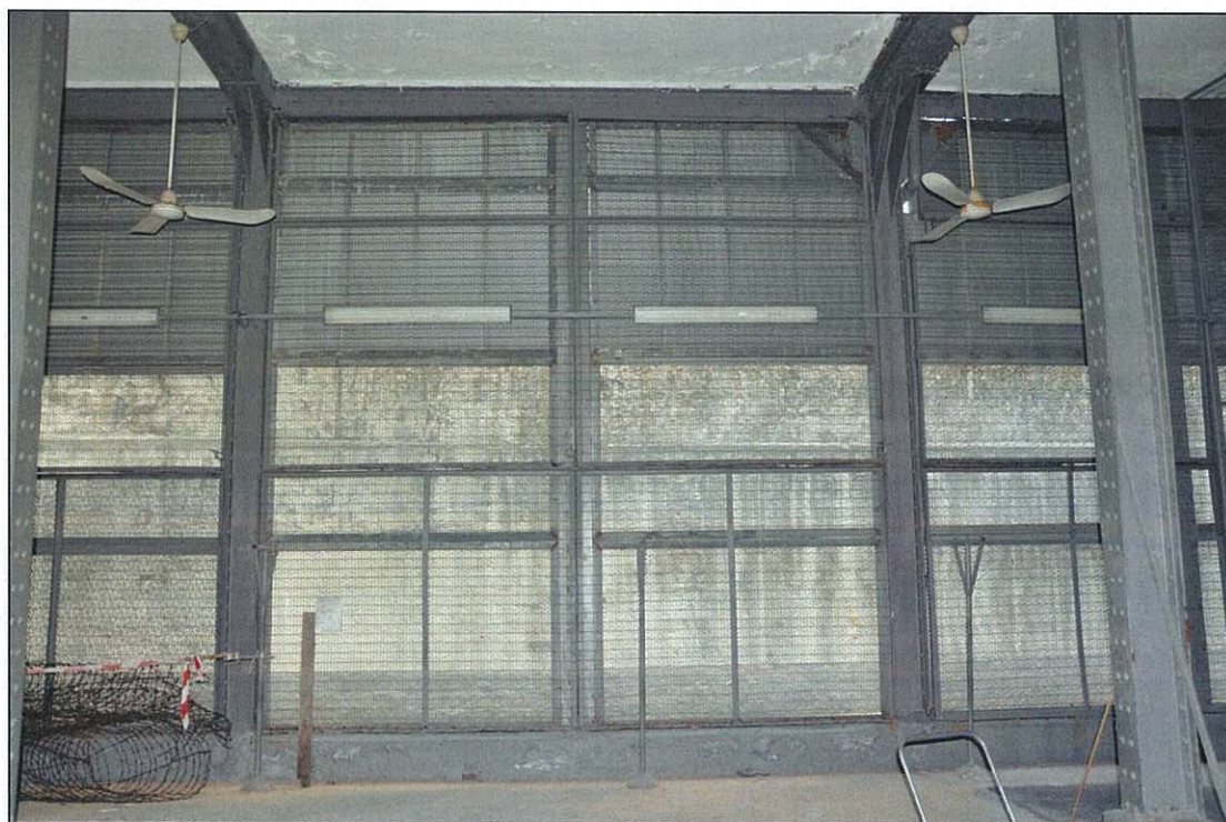
Photo 16.40 – Room LG1, interior view (2011/09/21)
