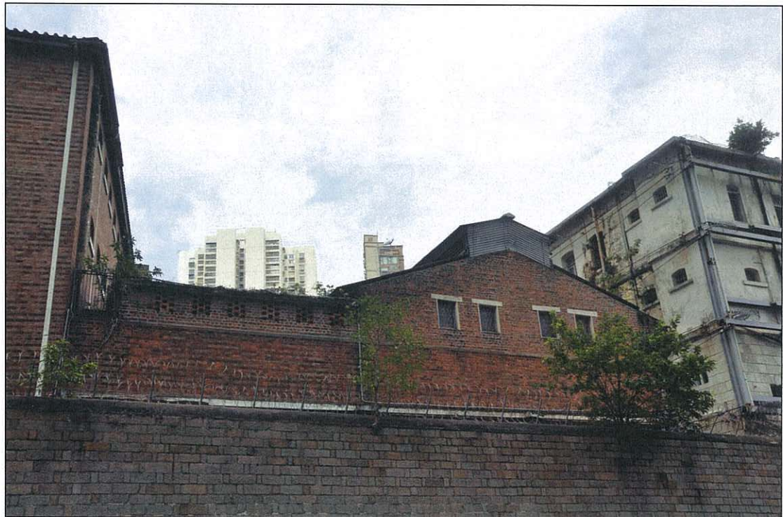
Photo 16.02 – External view from Arbutnot Road (2011/10/06)
