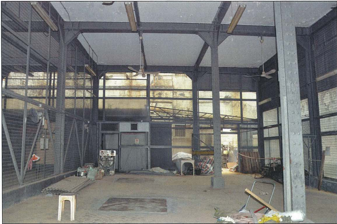
Photo 16.37 – Room LG1, interior view (2011/09/21)
