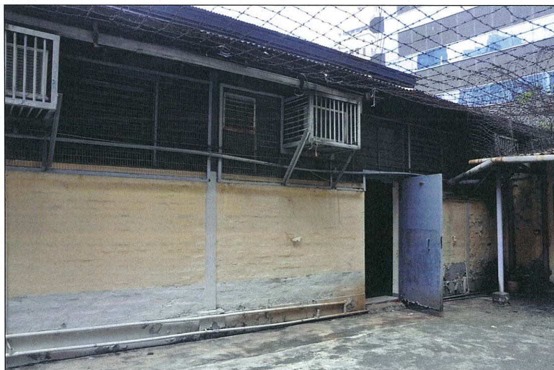
Photo 16.17 – External wall at yard (2011/09/07)
