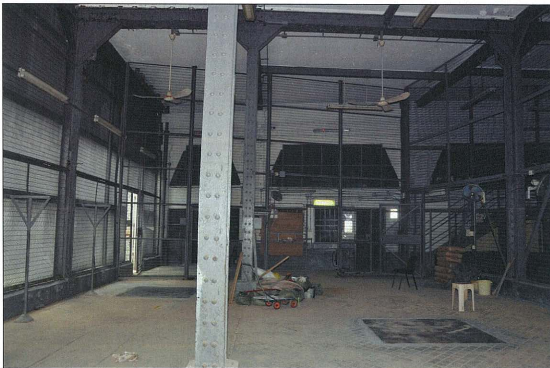
Photo 16.39 – Room LG1, interior view (2011/09/21)
