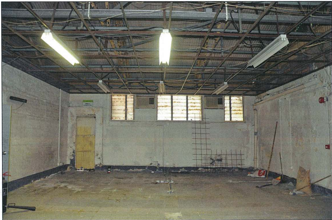
Photo 16.25 – Room G1, interior view (2011/09/07)
