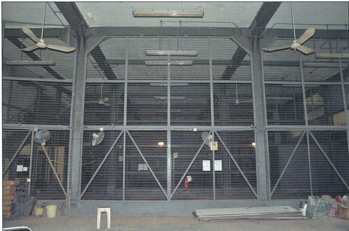
Photo 16.38 – Room LG1, interior view (2011/09/21)
