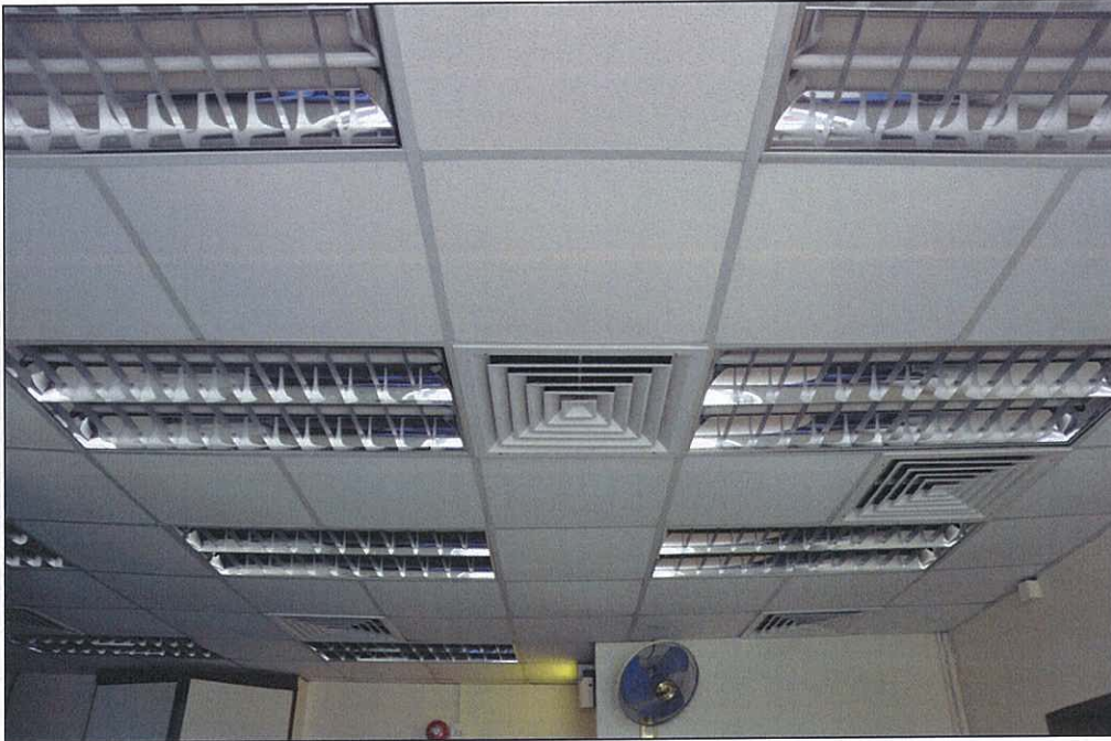
Photo 18.55 – Room 2, false ceiling (2011/10/03)
