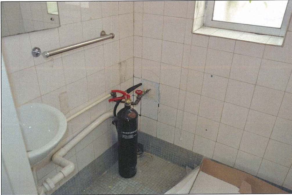
Photo 18.34 – Toilet (wash basin only) at Room 1, floor (2011/08/13)
