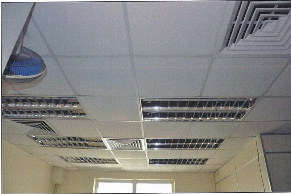
Photo 18.51 – Room 2, false ceiling (2011/10/03)
