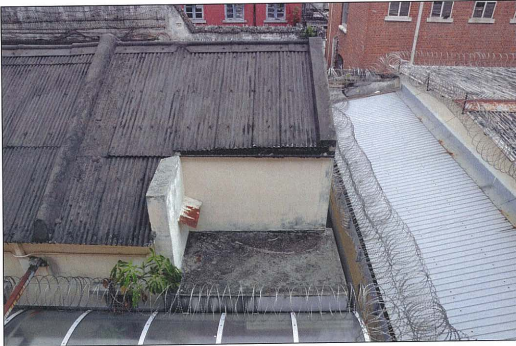
Photo 18.01 – Roof, photo taken on 1/f of Building 17 (2011/09/21)
