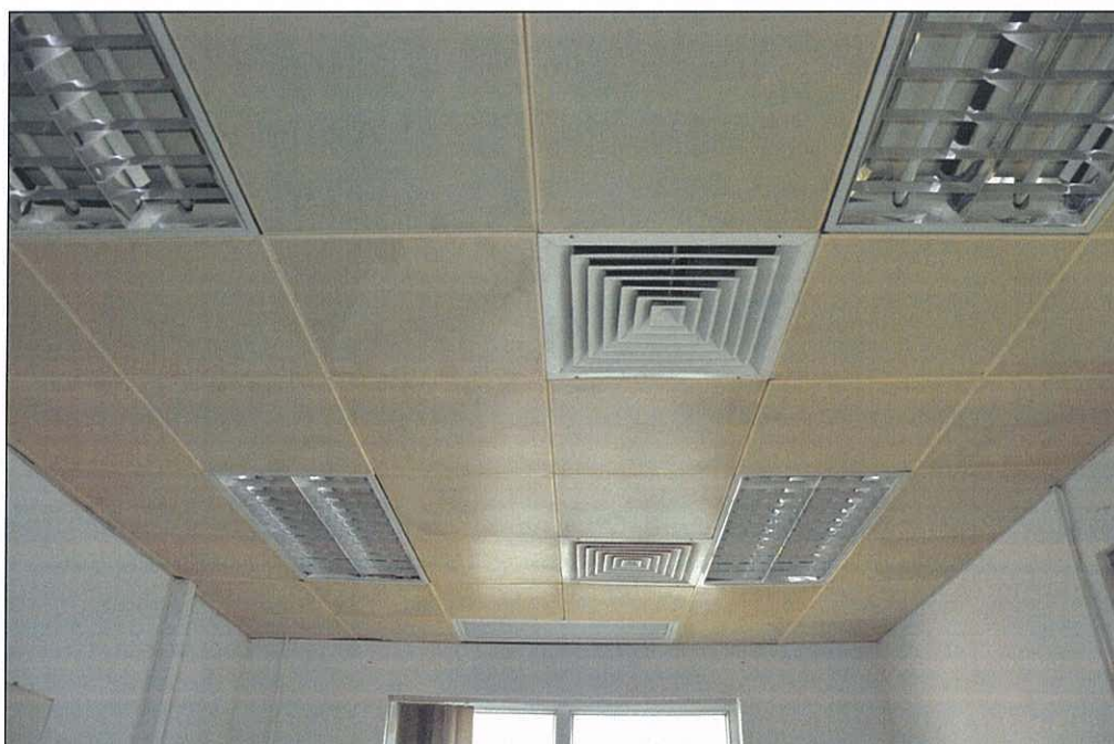
Photo 18.29 – Room 1, false ceiling (2011/10/03)
