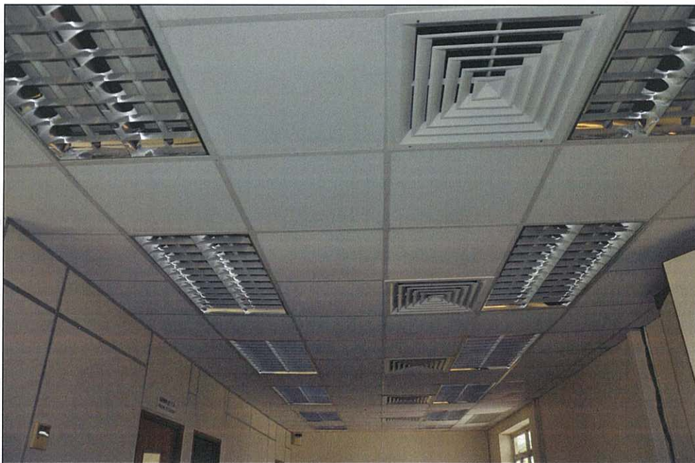
Photo 18.46 – Room 2, false ceiling (2011/10/03)
