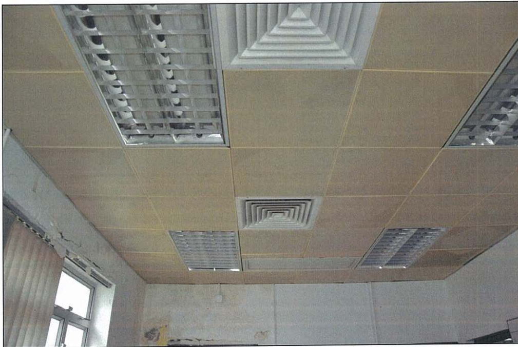
Photo 18.31 – Room 1, false ceiling (2011/10/03)
