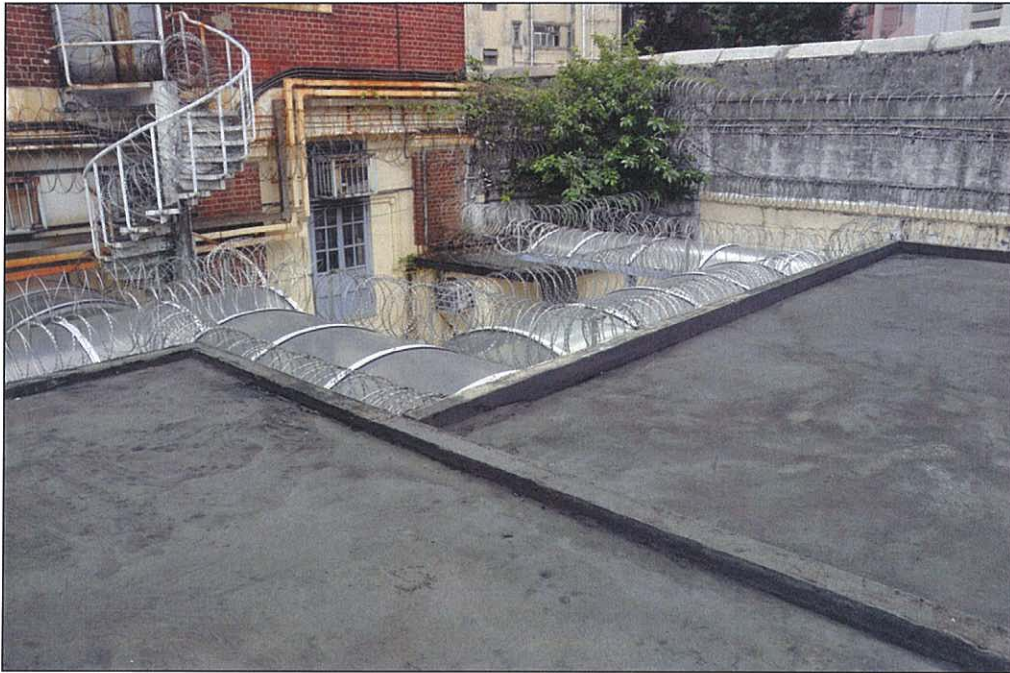
Photo 18.07 – Flat roof at west side (2011/09/02)
