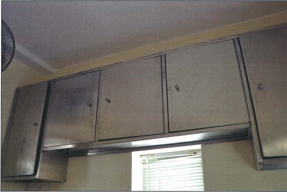
Photo 18.61 – Pantry at Room 2, stainless steel hanging cabinet (2011/08/13)
