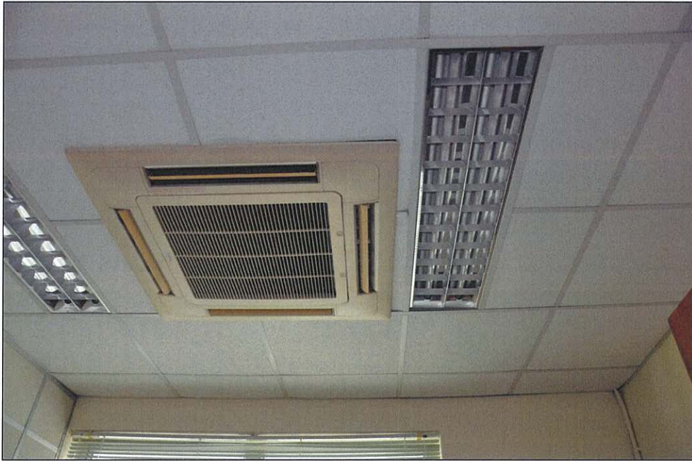
Photo 18.40 – Room 3, false ceiling (2011/10/03)
