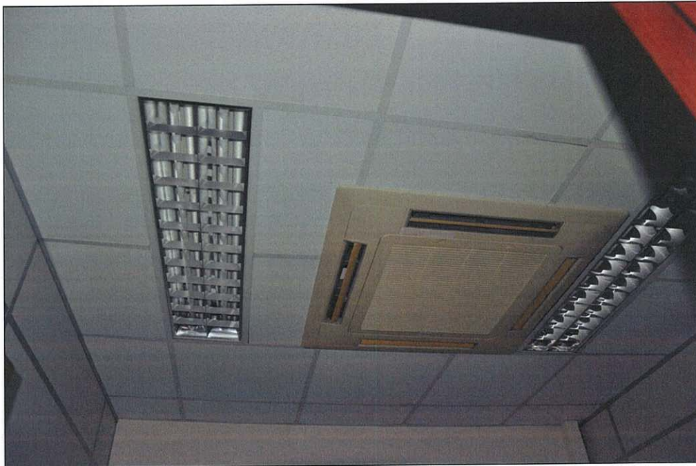
Photo 18.43 – Room 4, false ceiling (2011/10/03)
