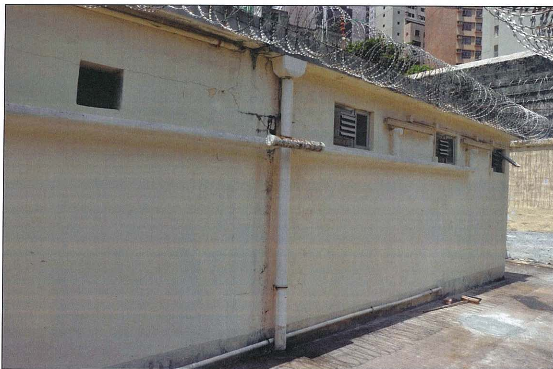
Photo 18.24 – North elevation, west part (2011/08/13)
