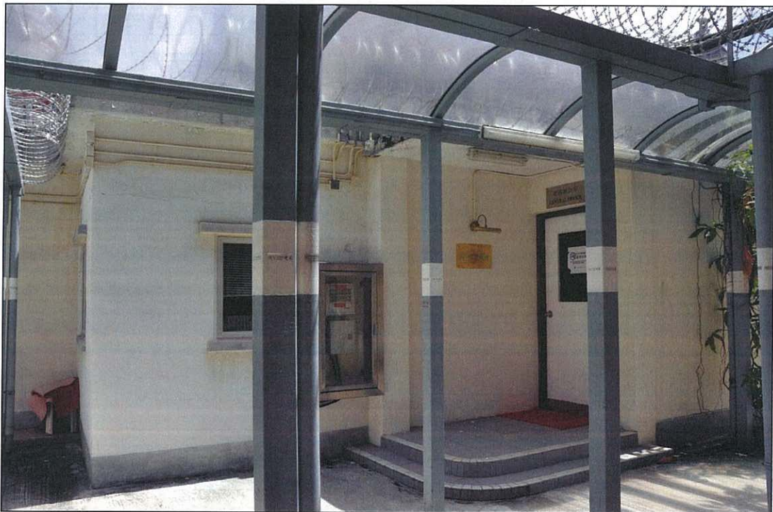
Photo 18.18 – Door at west side of south elevation (2011/08/13)
