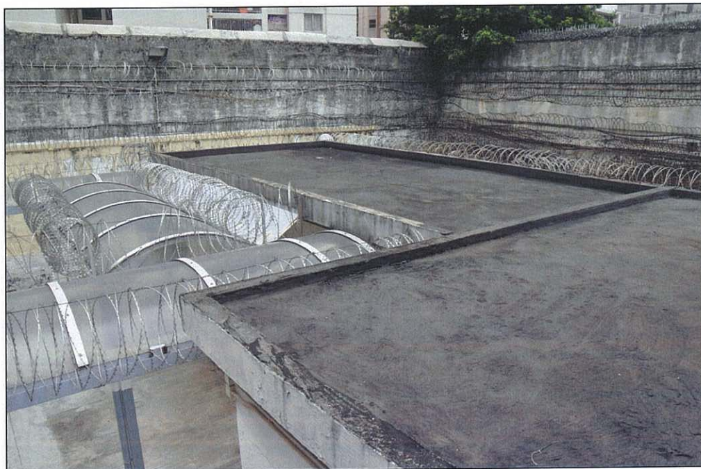
Photo 18.06 – Flat roof at west side (2011/09/02)
