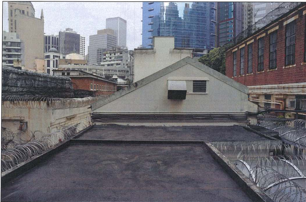
Photo 18.08 – Flat roof at west side (2011/09/02)
