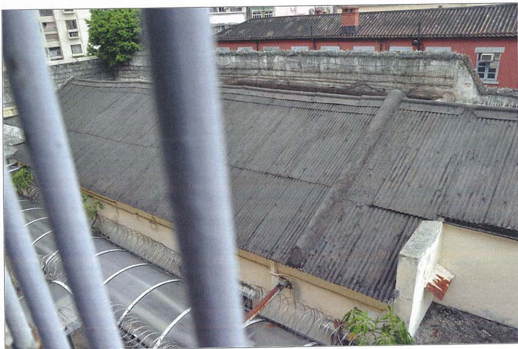
Photo 18.02 – Roof, photo taken on 1/f of Building 17 (2011/09/21)
