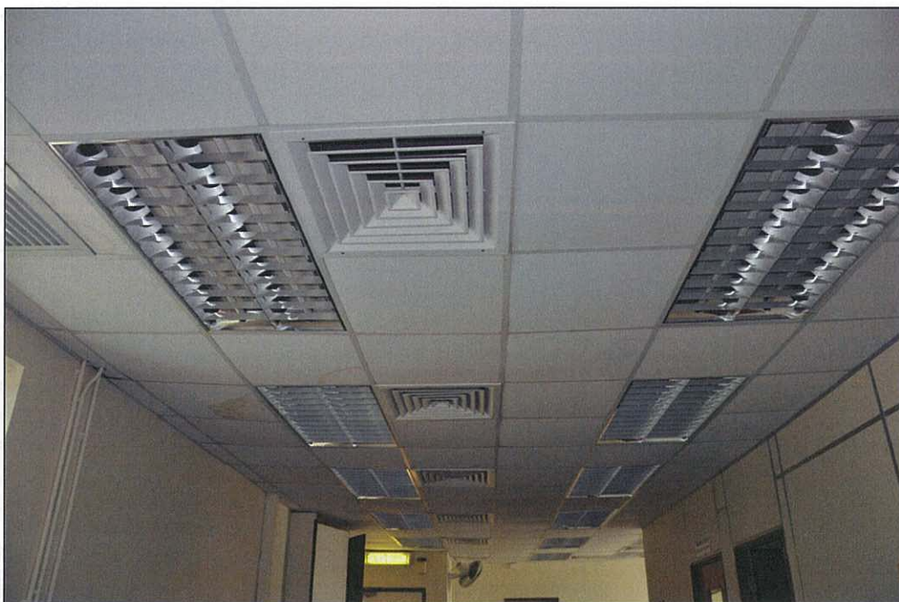
Photo 18.36 – Room 1, false ceiling (2011/10/03)
