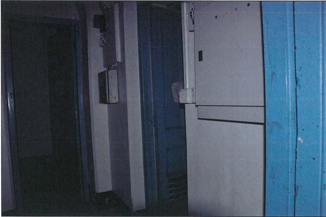
Photo 5.48 – Rear room 2, entrance from Building 4 (2011/08/15)
