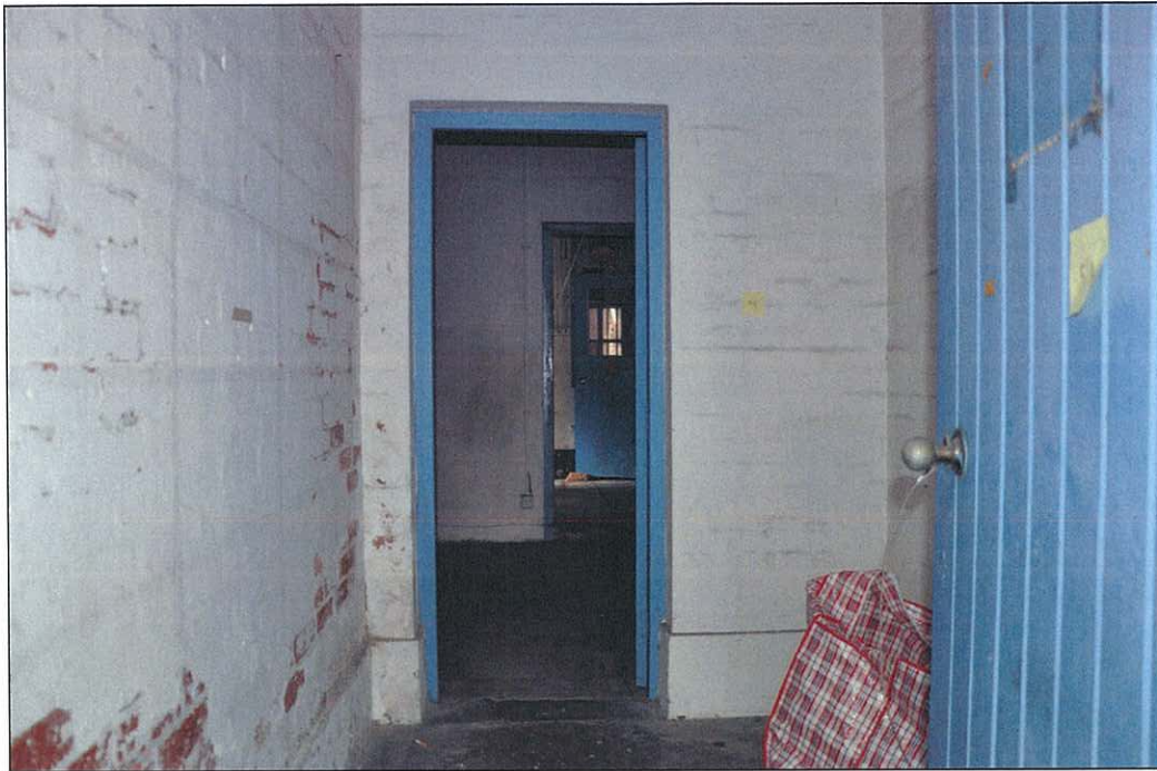
Photo 5.46 – Rear room 1, interior (2011/08/15)
