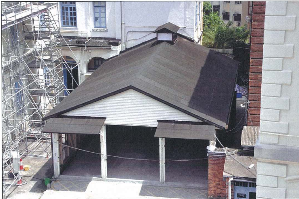
Photo 5.02 – Roof from high level (2011/08/29)
