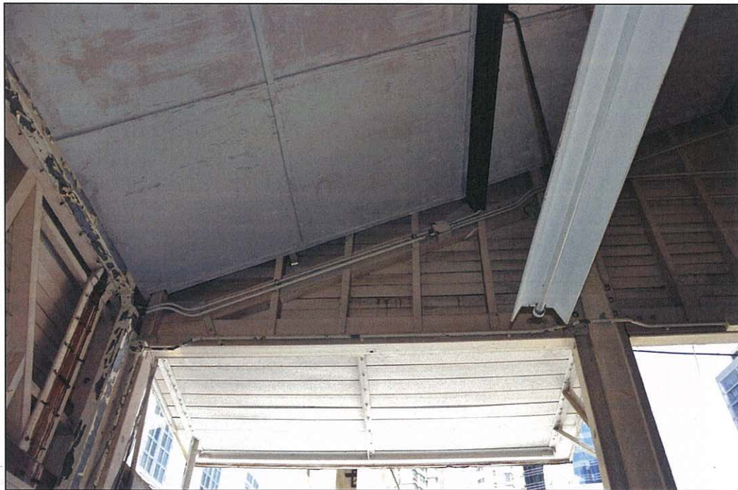
Photo 5.36 – View of timber cladding above north side entrance from internal (2011/08/13)
