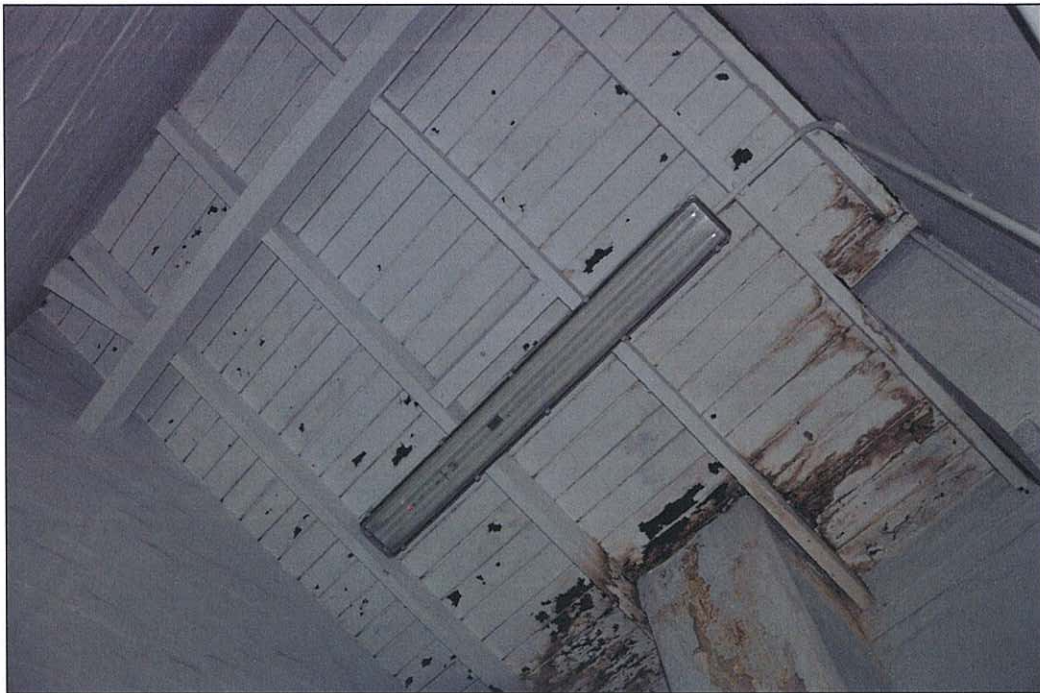
Photo 5.54 – Rear room 2, soffite of roof (2011/08/15)
