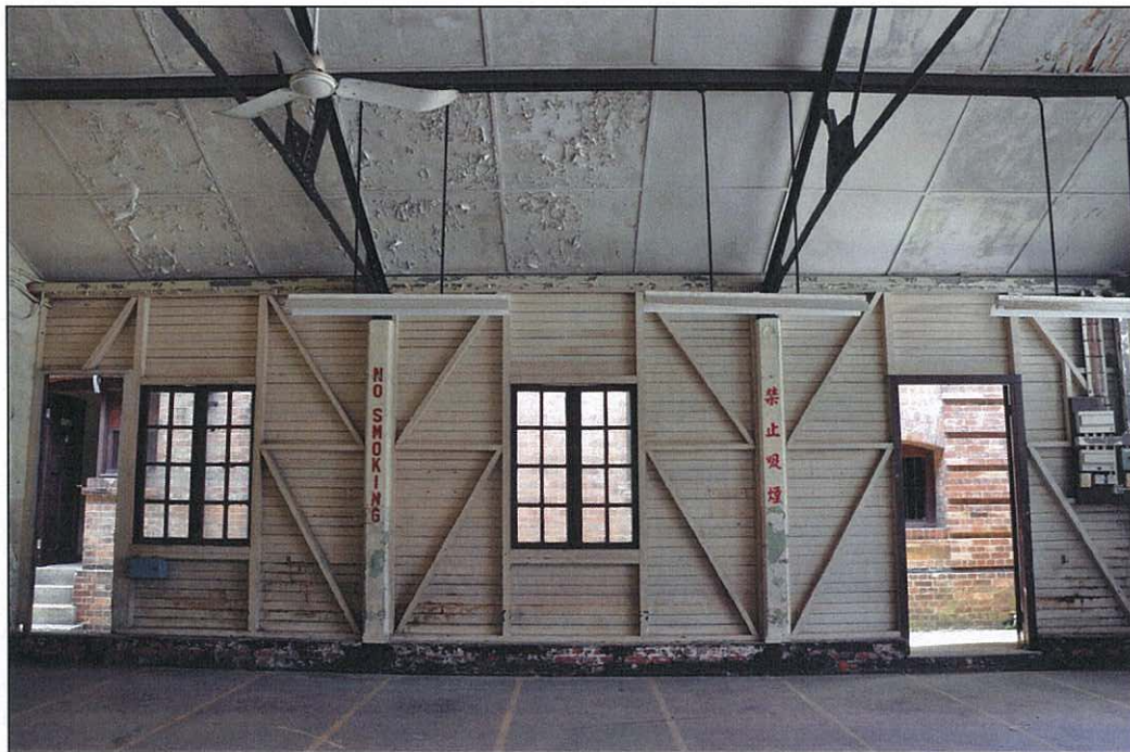
Photo 5.28 – Internal view of south external wall (2011/08/13)
