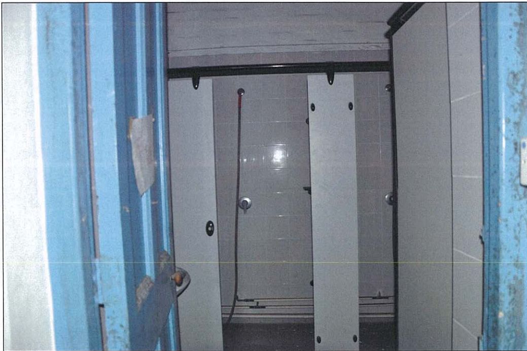
Photo 5.50 – Rear room 2, interior (2011/08/15)
