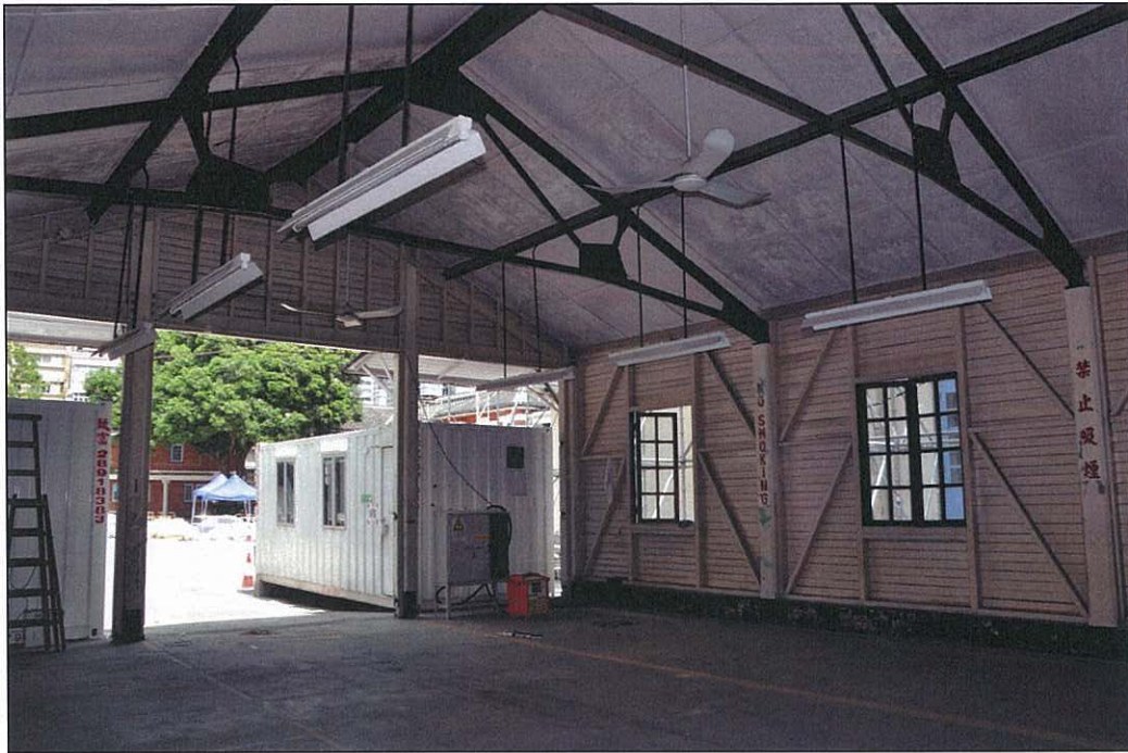
Photo 5.29 – View of entrance from internal end wall (2011/08/13)
