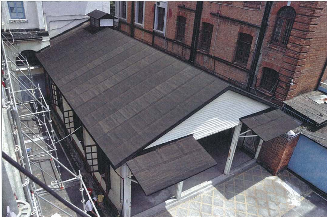
Photo 5.04 – Roof from high level (2011/08/29)
