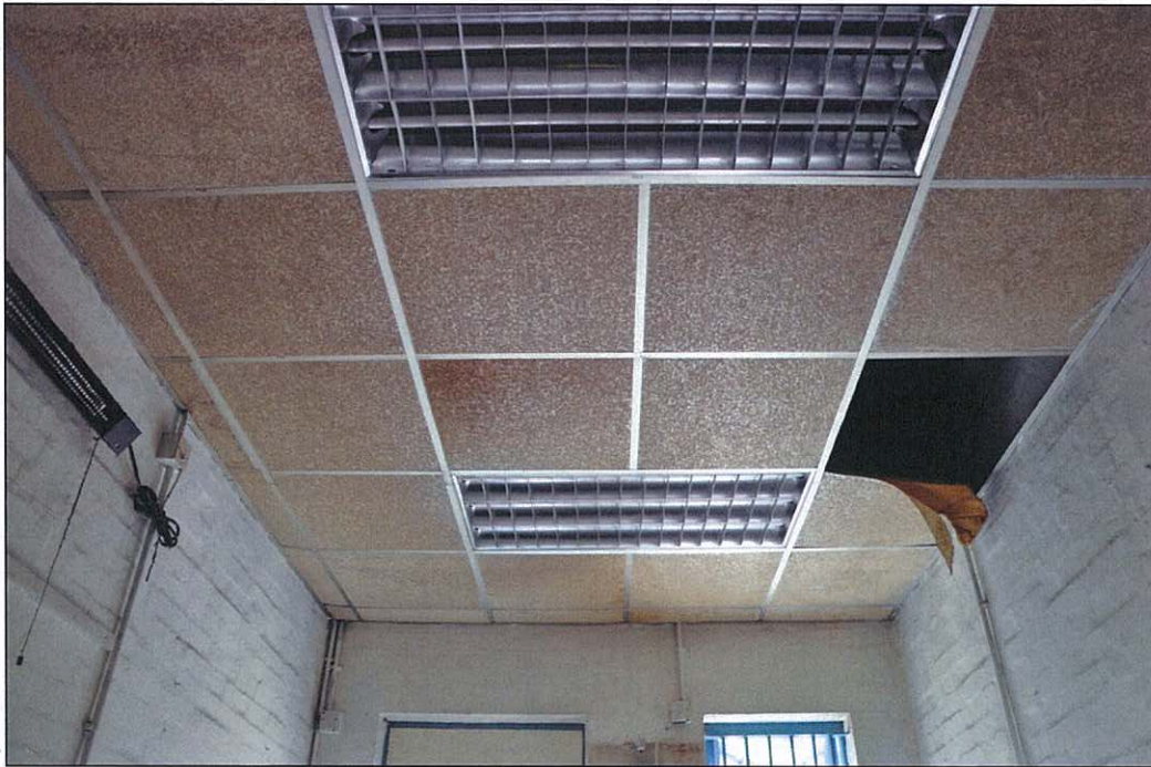
Photo 5.63 – Rear room 4, false ceiling (2011/08/13)
