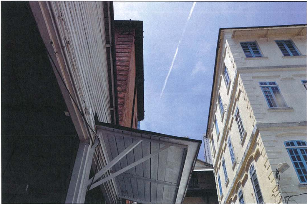
Photo 5.35 – Sun shade at south side entrance (2011/08/13)
