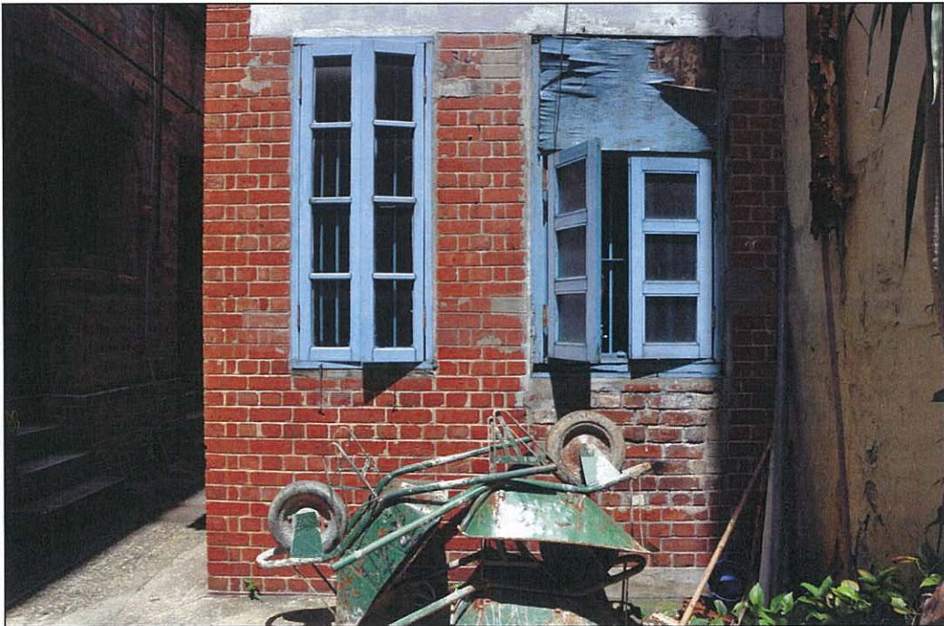
Photo 5.20 – Brick end wall, lower part (2011/08/13)
