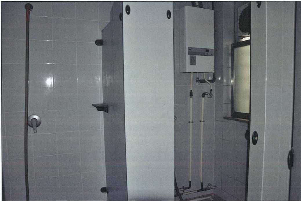
Photo 5.51 – Rear room 2, interior (2011/08/15)
