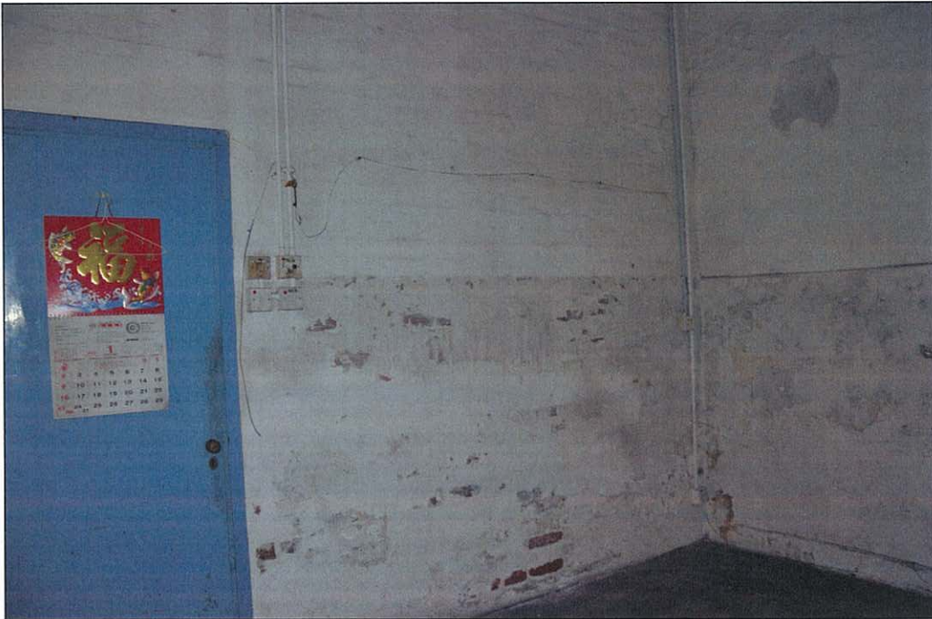
Photo 5.56 – Rear room 3, interior (2011/08/13)
