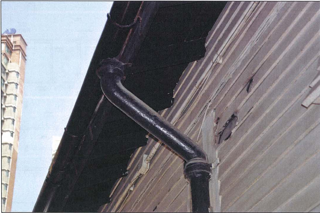
Photo 5.21 – South side external wall, eaves water gutter and swanneck (2011/08/13)
