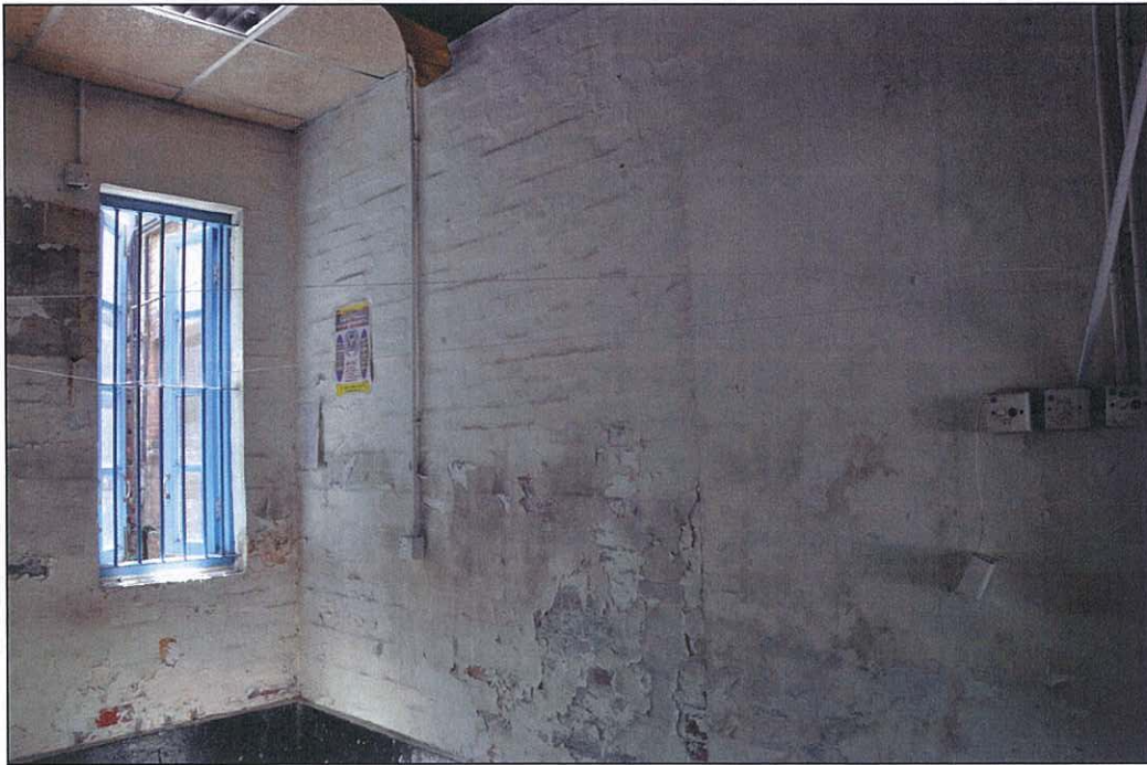
Photo 5.65 – Rear room 4, interior (2011/08/13)
