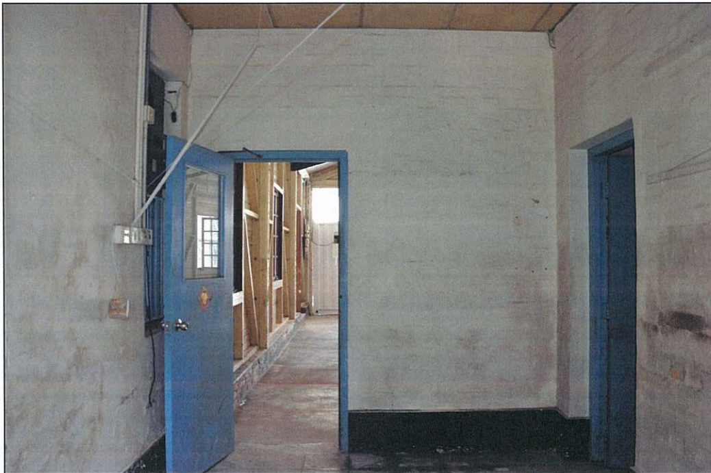
Photo 5.66 – Rear room 4, interior (2011/08/13)
