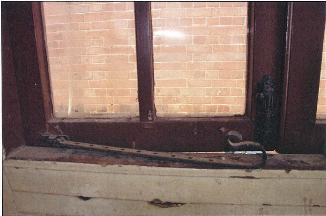
Photo 5.43 – Wrought iron lower vertical bolt and window stay (2011/08/13)
