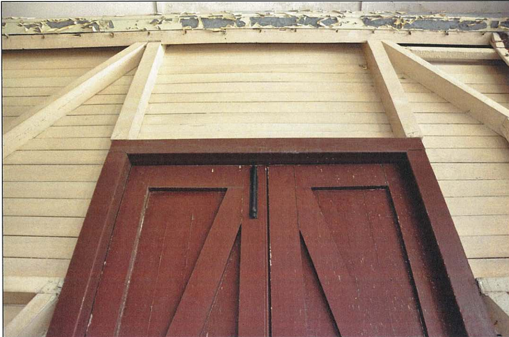
Photo 5.38 – Upper vertical bolt (2011/08/13)
