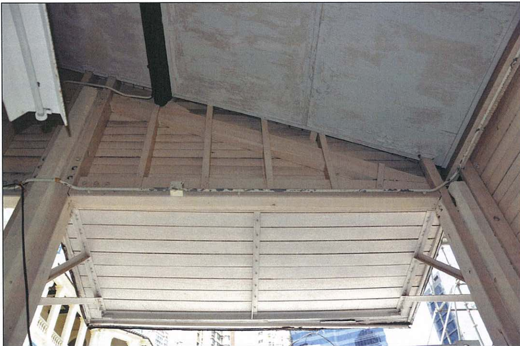
Photo 5.34 – View of timber cladding above north side entrance from internal (2011/08/13)
