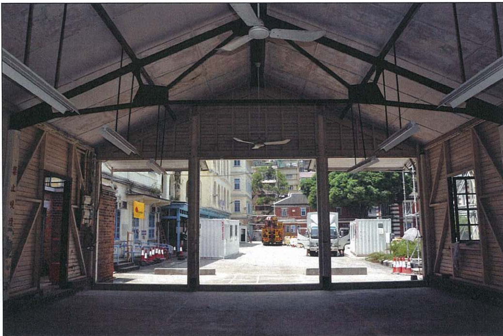
Photo 5.30 – View of entrance from internal end wall (2011/08/29)
