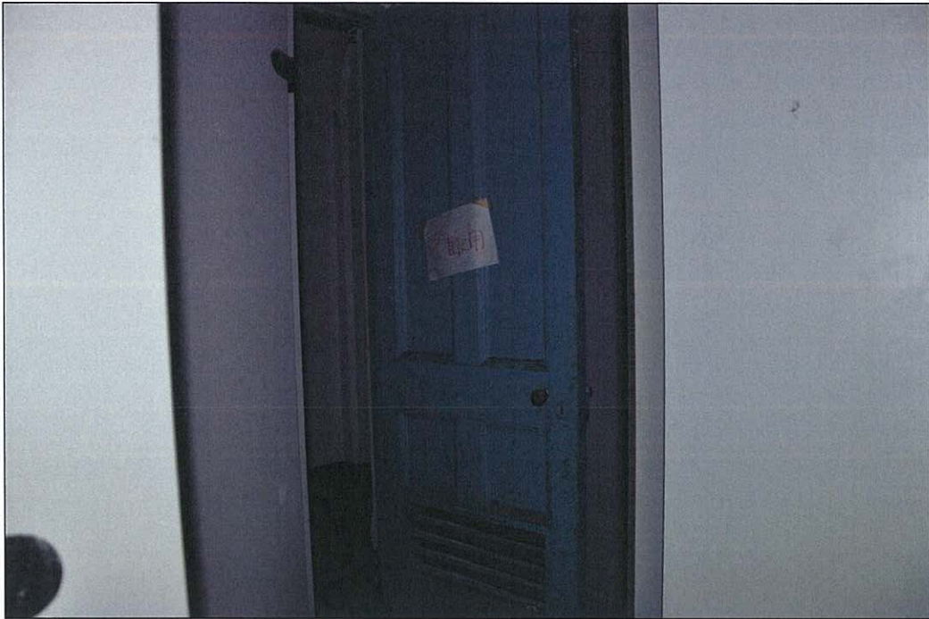
Photo 5.52 – Rear room 2, interior (2011/08/15)
