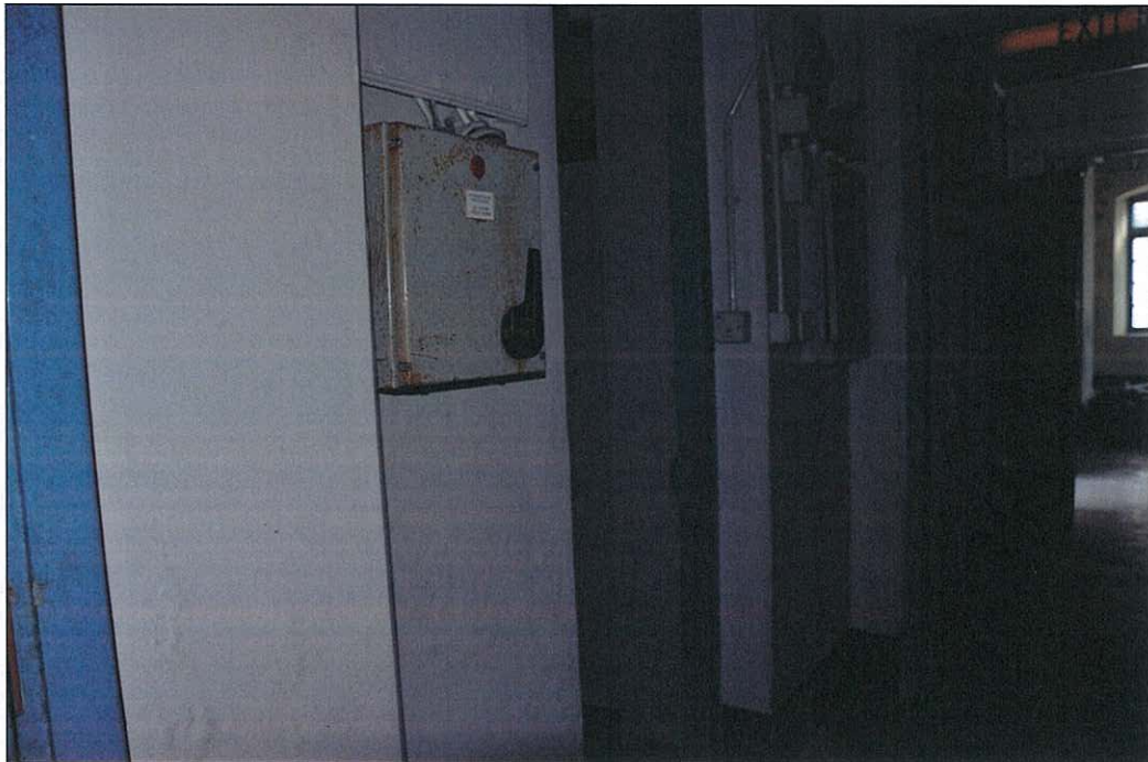
Photo 5.49 – Rear room 2, entrance from Building 4 (2011/08/15)
