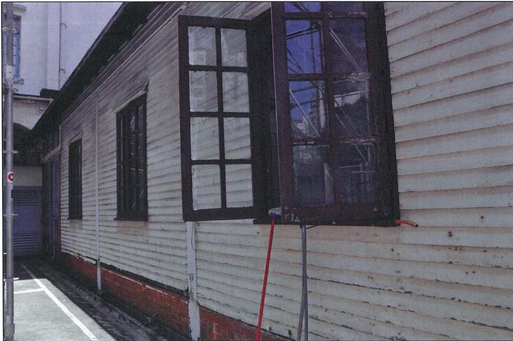
Photo 5.11 – North side external wall, front part (2011/08/13)
