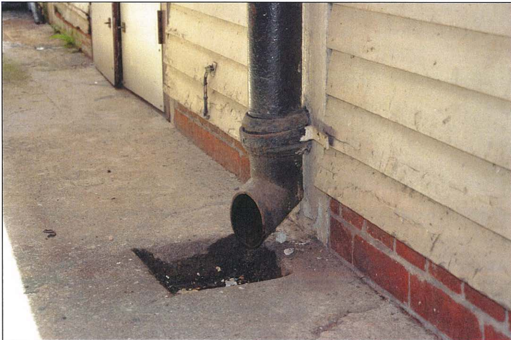
Photo 5.22 – South side external wall, rainwater downpipe and shoe (2011/08/13)
