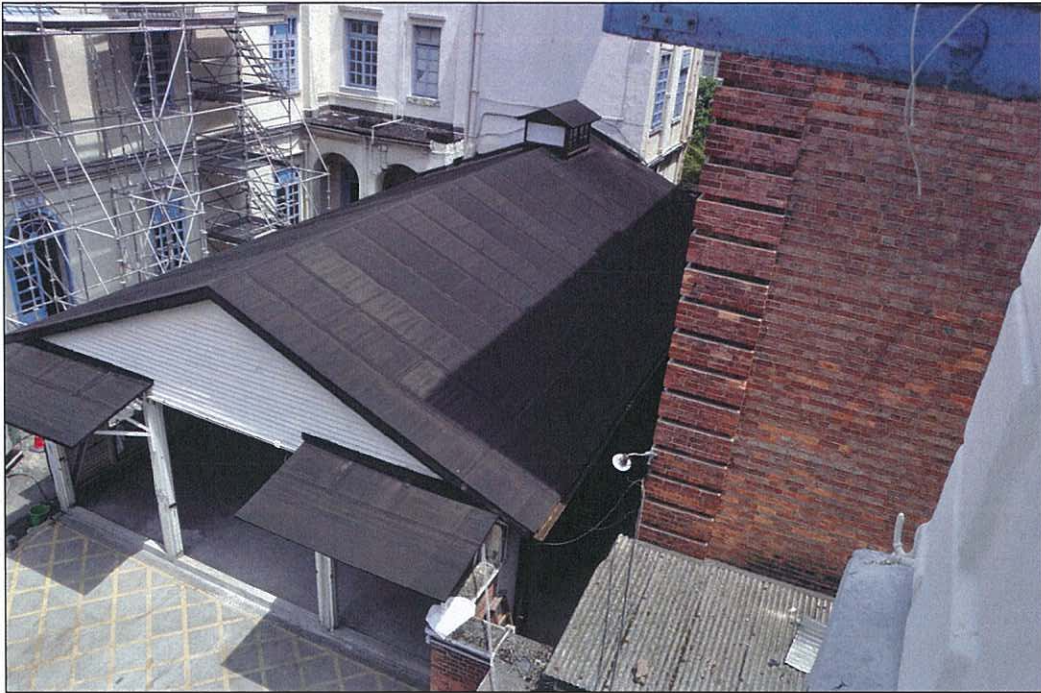
Photo 5.03 – Roof from high level (2011/08/29)
