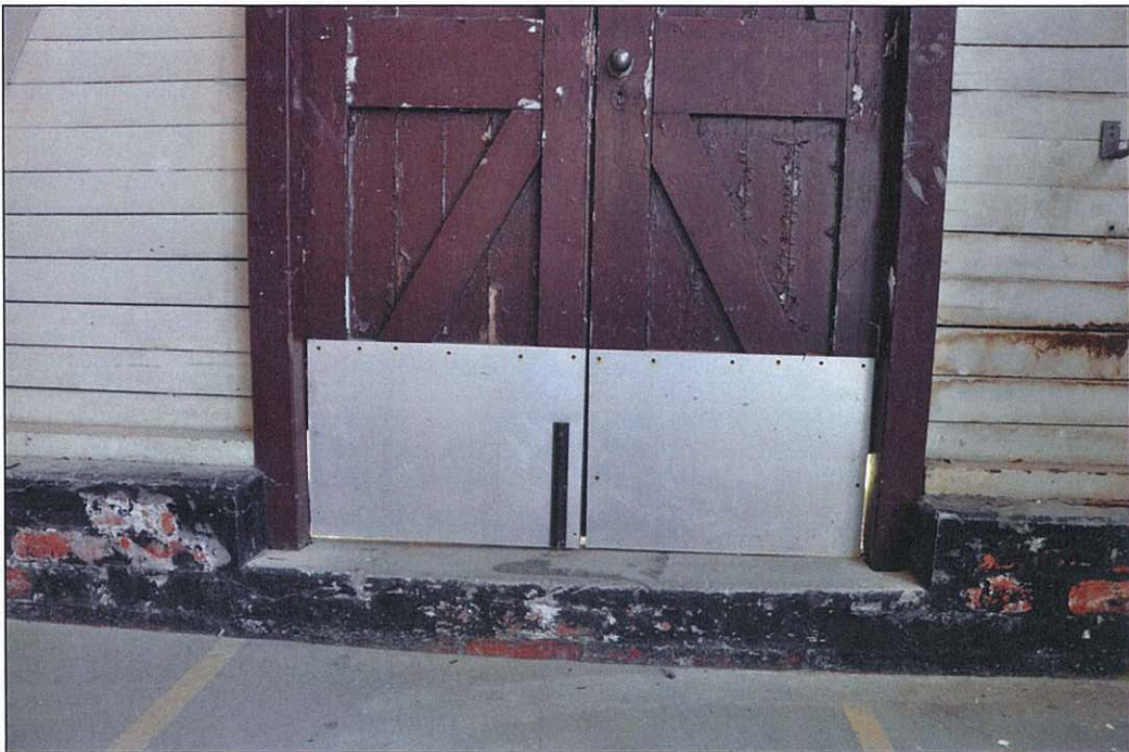
Photo 5.39 – Lower vertical bolt (2011/08/13)
