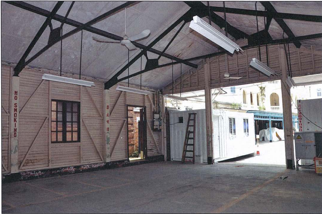
Photo 5.31 – View of entrance from internal end wall (2011/08/13)
