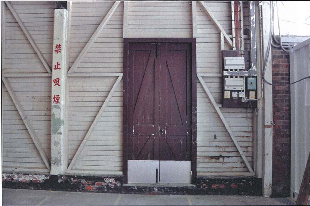
Photo 5.37 – Internal side of door at south external wall (2011/08/13)
