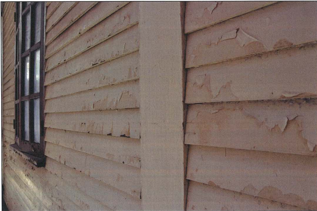
Photo 5.16 – Close up view of the external overlapping timber cladding (2011/08/13)
