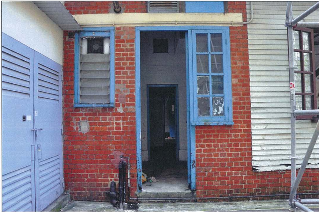
Photo 5.45 – Entrance to rear room 1 at external (2011/08/15)
