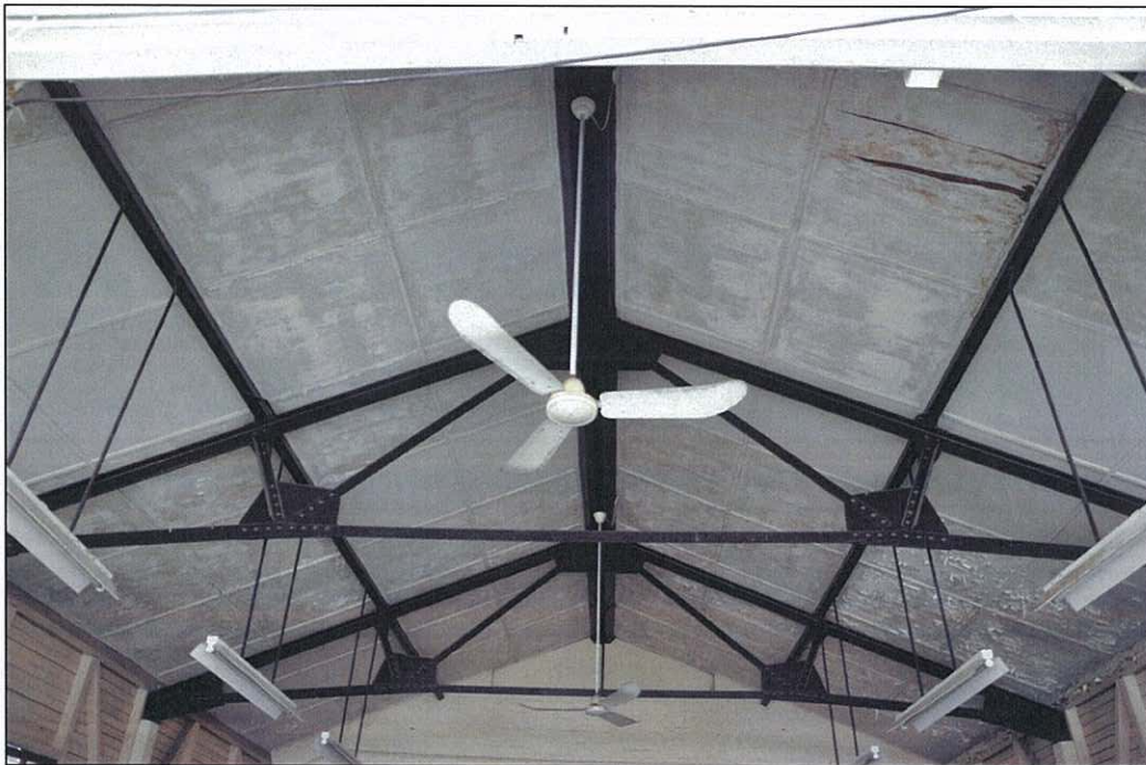
Photo 5.24 – Ceiling view from entrance (2011/08/13)
