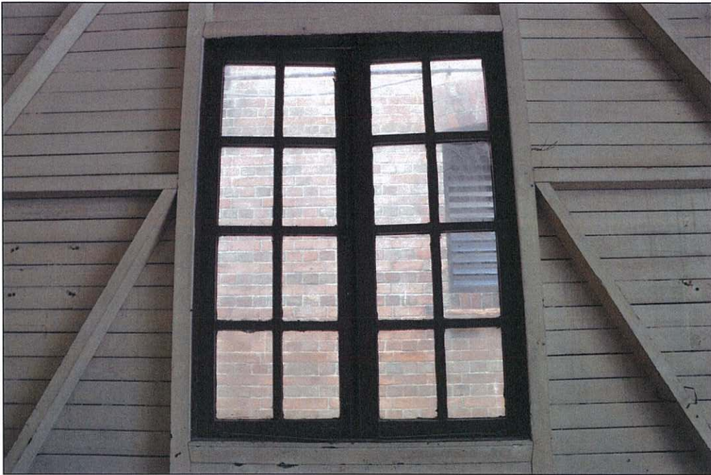
Photo 5.41 – Internal side of casement at south external wall (2011/08/13)
