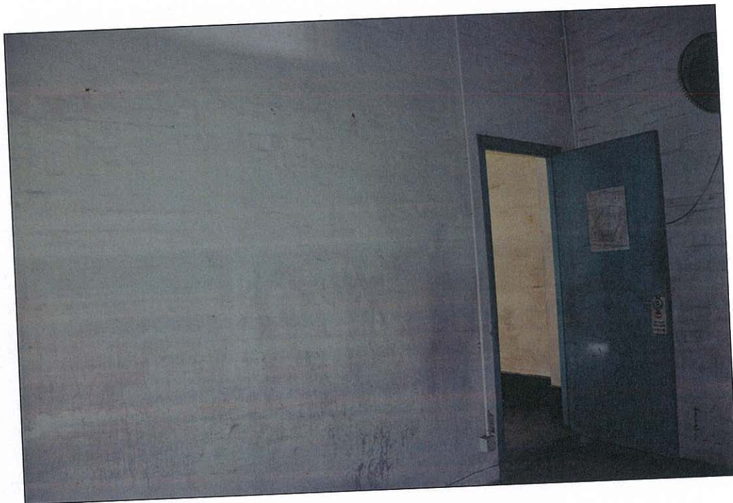
Photo 5.60 – Rear room 3, interior (2011/08/13)
