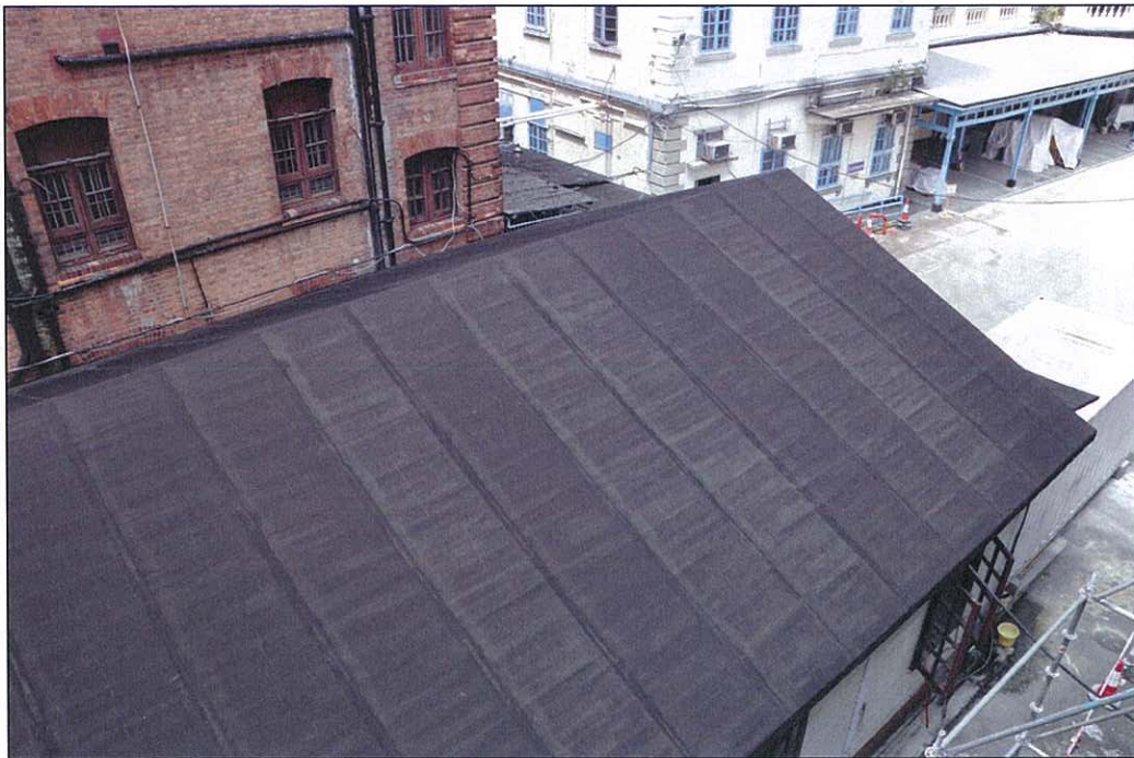
Photo 5.05 – Roof from high level (2011/08/13)
