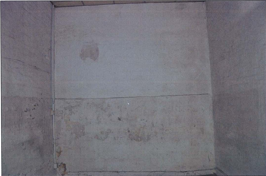
Photo 5.55 – Rear room 3, interior (2011/08/13)
