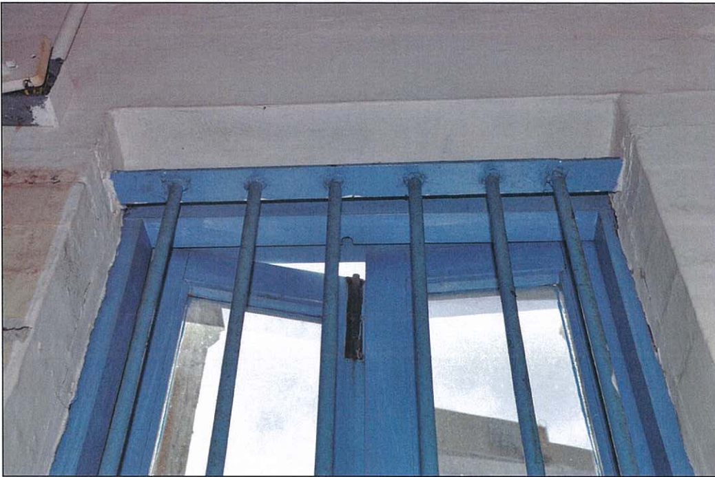
Photo 5.69 – Rear room 4, upper vertical bolt of timber casement window (2011/08/13)
