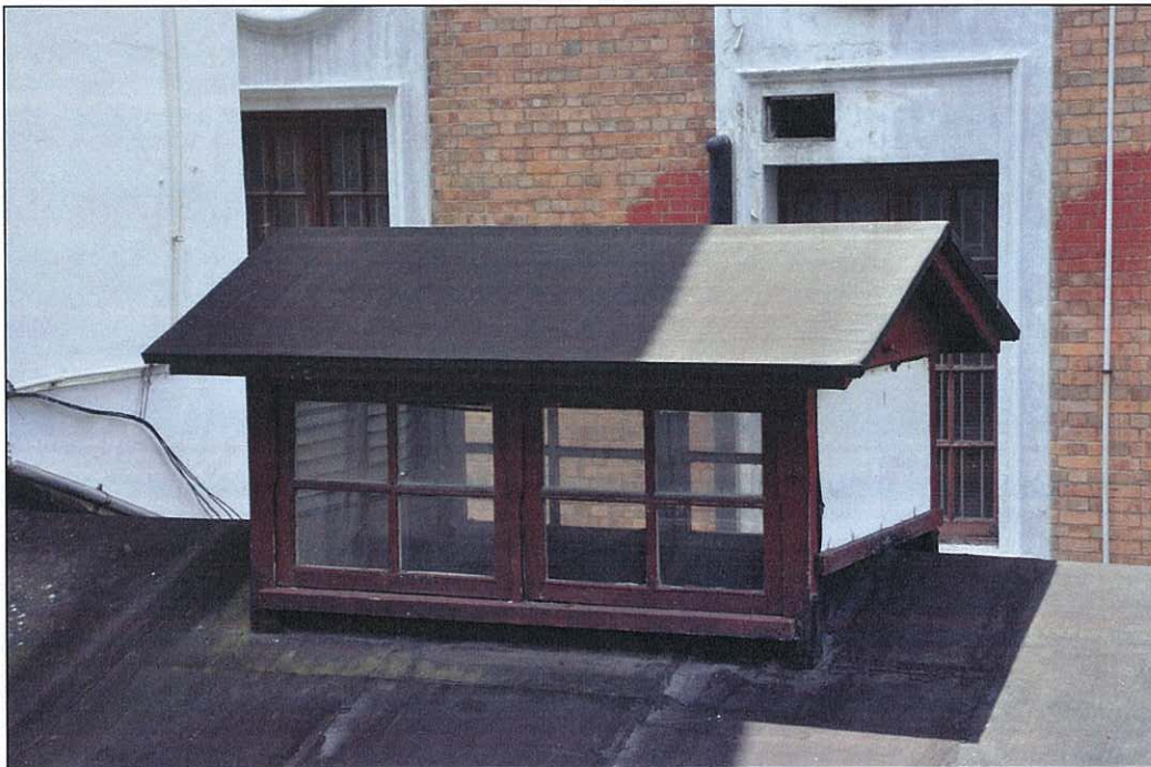
Photo 5.06 – Lantern on the roof (2011/08/13)
