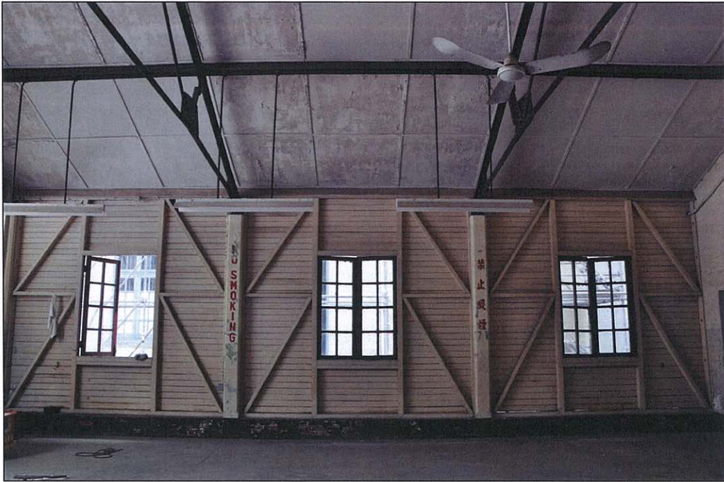
Photo 5.27 – Internal view of north external wall (2011/08/13)
