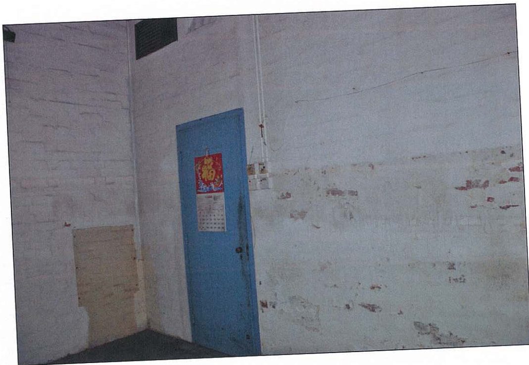
Photo 5.59 – Rear room 3, interior (2011/08/13)
