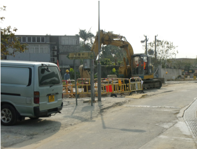
Construction works observed within close proximity of SR77 (Date: 27 December 2013)
