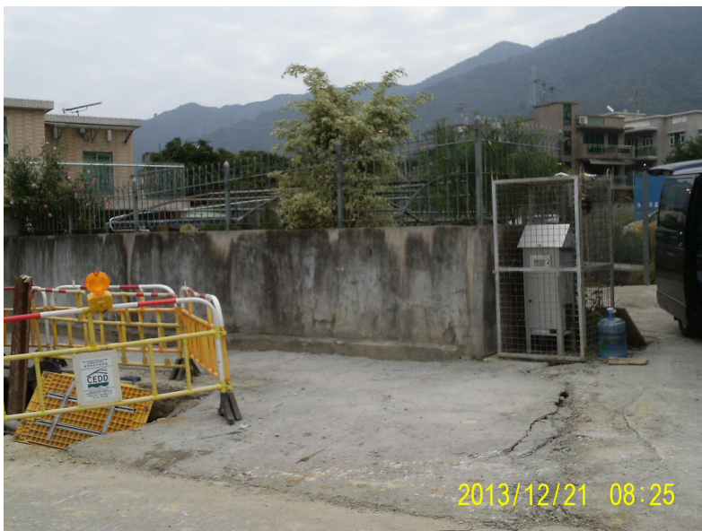
Construction works observed within close proximity of SR77 (Date: 21 December 2013)
