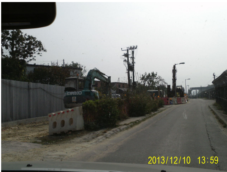
Construction works observed within close proximity of SR77 (Date: 10 December 2013)
