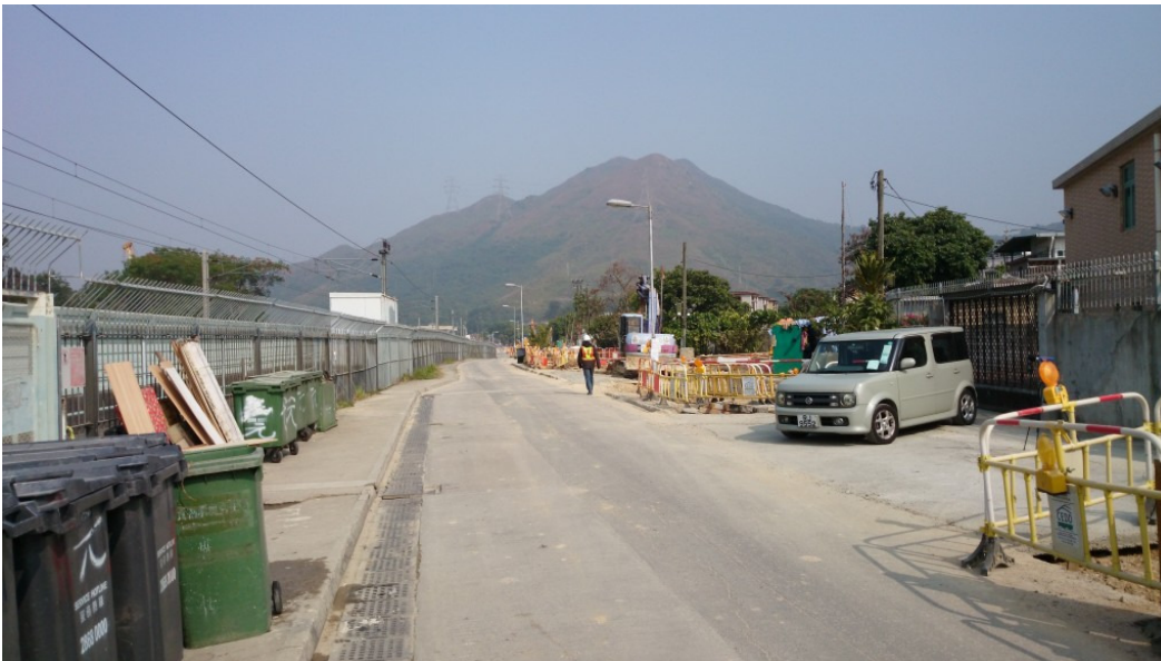
Construction works observed within close proximity of SR77 (Date: 27 December 2013)
