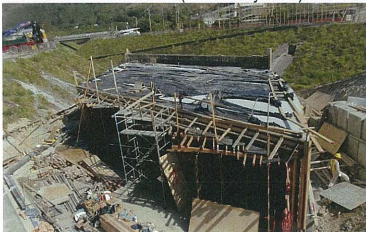
Construction works at ID4 (24 January 2014)
