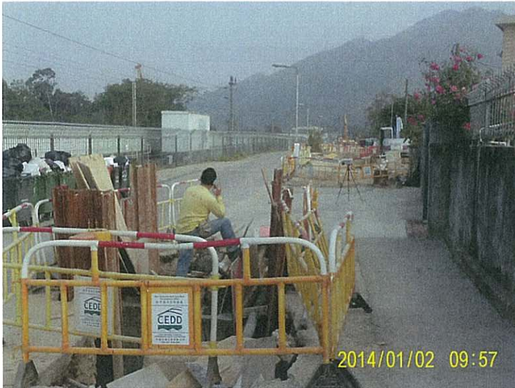
Construction works observed within close proximity of SR77 (Date: 2 January 2014)
