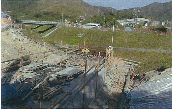
The construction works are properly protected with sand bags. (Date: 24 January 2014)
