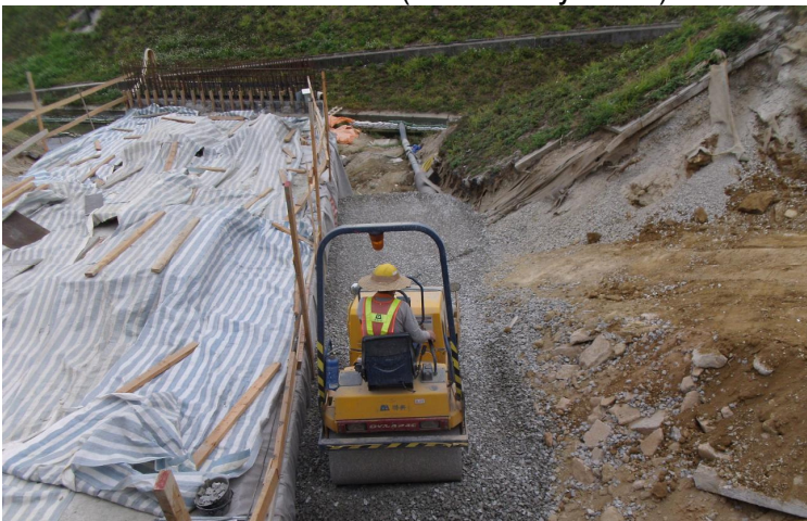
Construction works at ID5 (7 February 2014)
