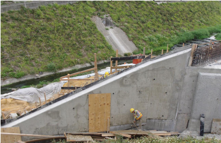
Construction works at ID4 (7 February 2014)
