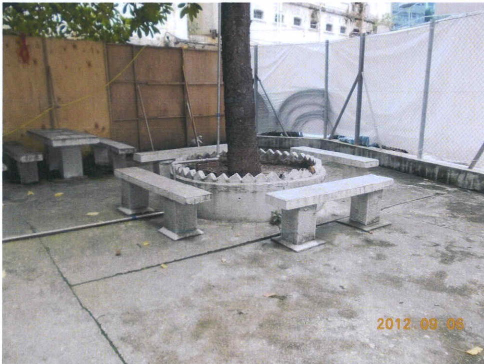
Fig. 3 The site inside the cordon zone is clean and tidy.
