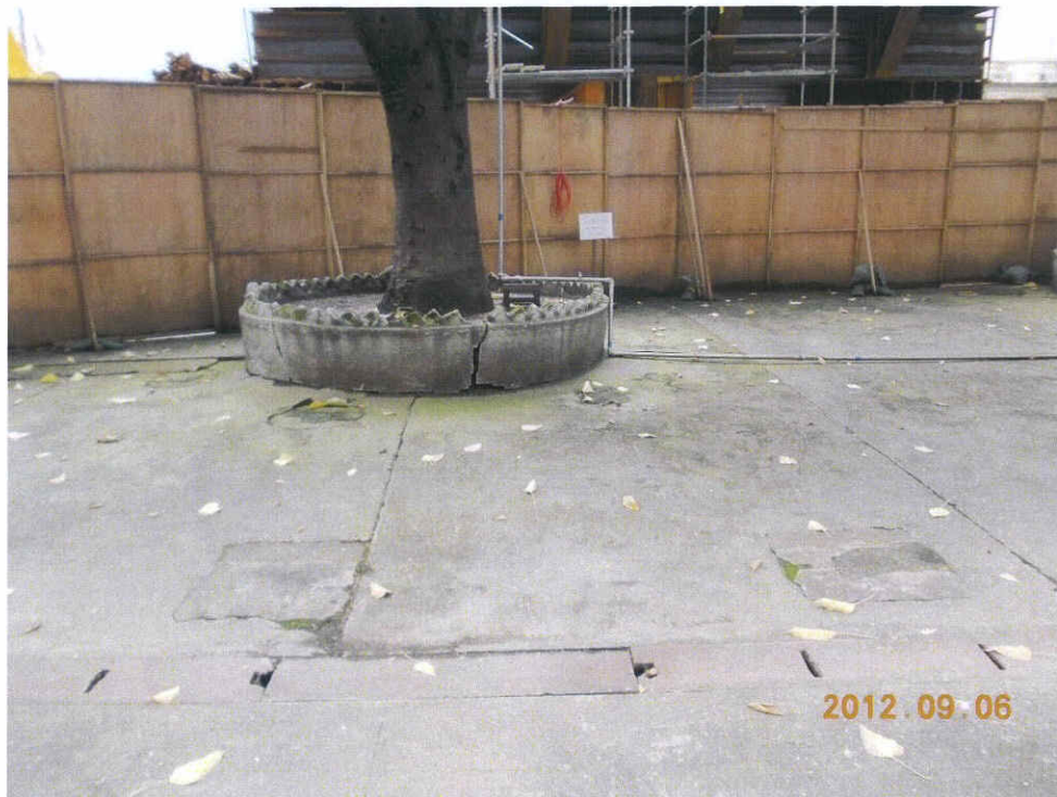
Fig. 5 Cleanliness of the site is acceptable.
