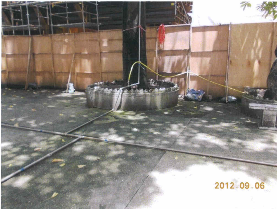
Fig. 3 The site appears clean and tidy at the time of inspection.
