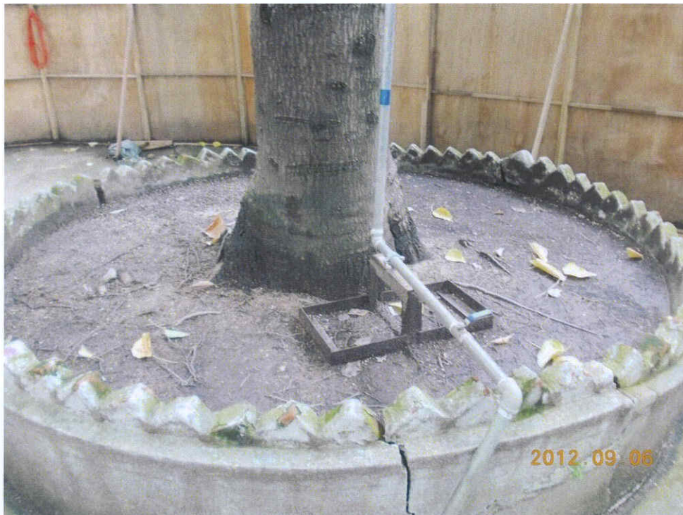
Fig 2. Cleanliness of the planter is acceptable.
