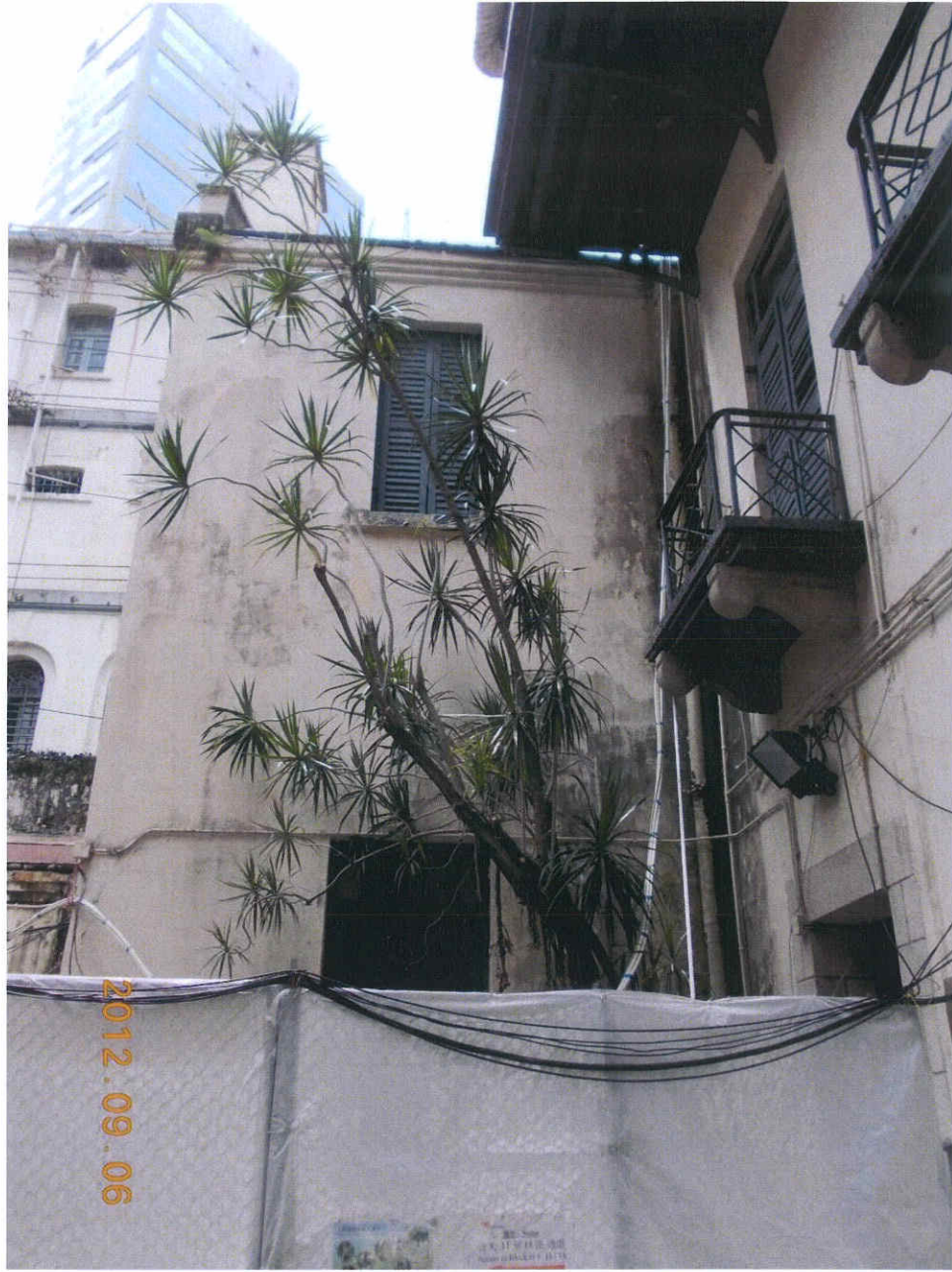
Fig. 6 Overall view of Tree-11 during inspection on 6 th September 2012.
