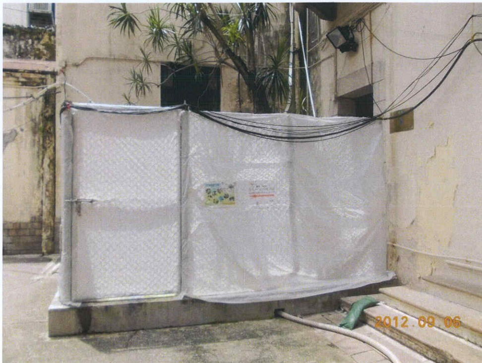
Fig. 5 The site outside the cordon zone is clean and tidy at the time of inspection.
