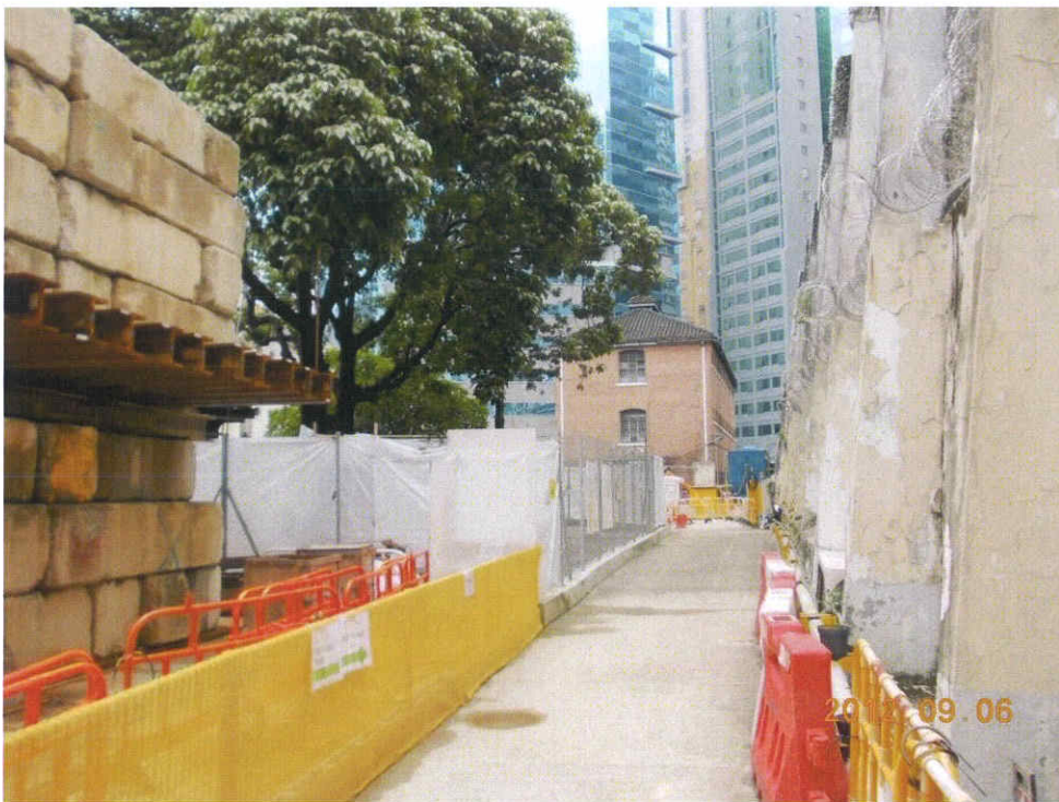
Fig. 7 The access near the cordon zone appears clean and tidy.
