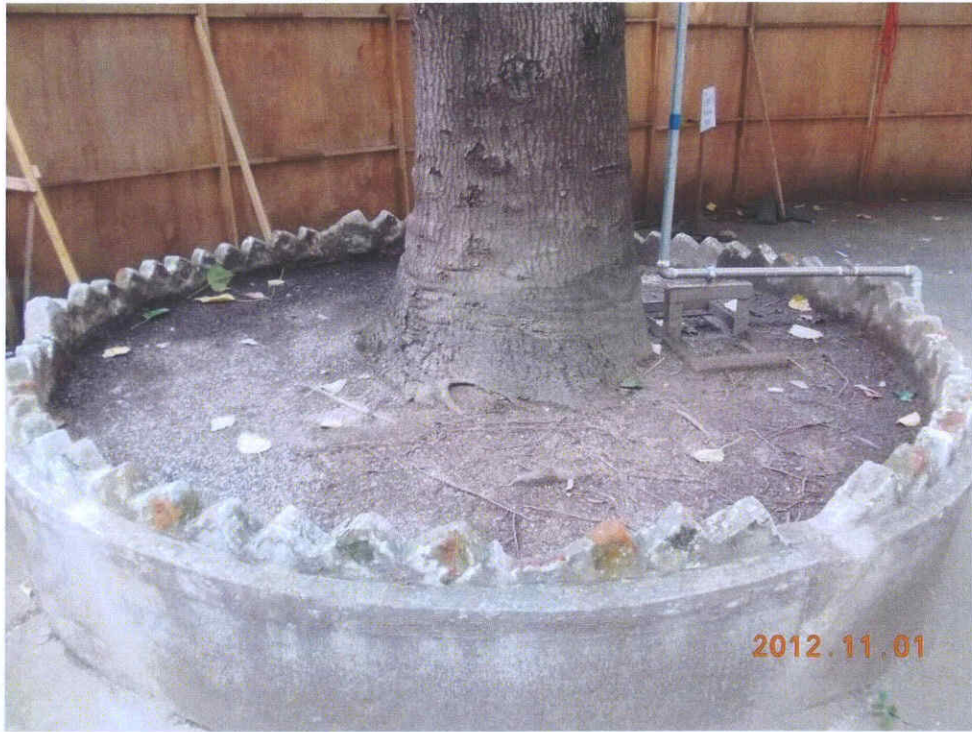
Fig 2. Cleanliness of the planter is acceptable. No new cracks have been detected on 1.11.2012.
