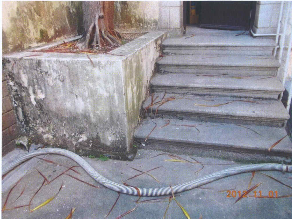
Fig. 3 Cleanliness of the site is acceptable.
