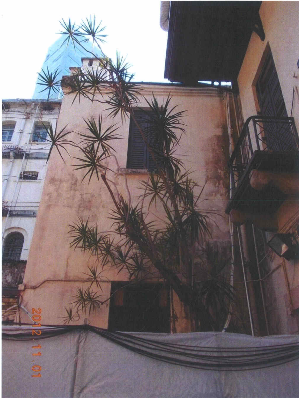
Fig. 6 Overall view of Tree-11 during inspection on 1 st November 2012.
