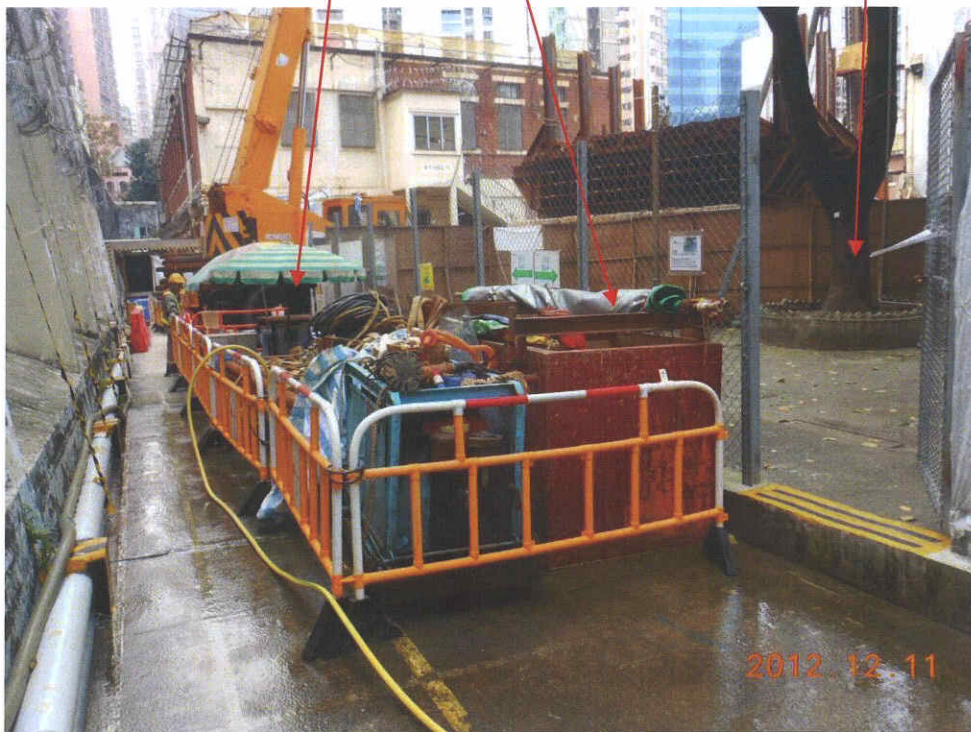
Fig. 5 Lots of construction equipment are placed outside the cordon zone. T-6
