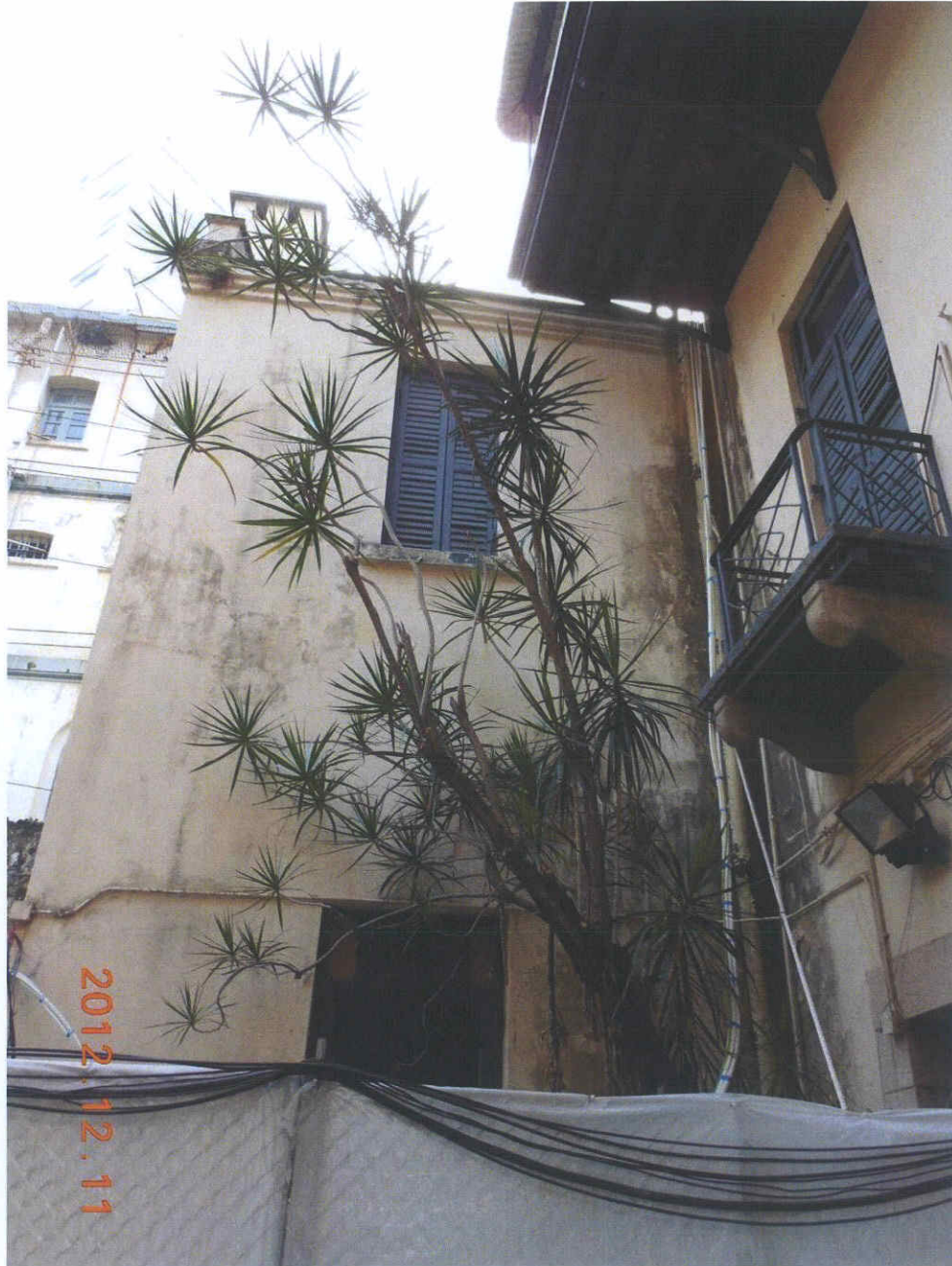
Fig. 6 Overall view of Tree-11 during inspection on 11 th December 2012.
