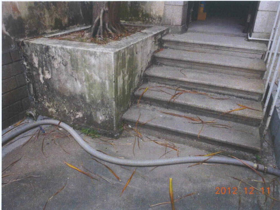
Fig. 3 Cleanliness of the site is acceptable.
