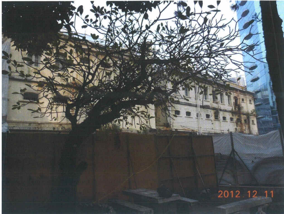
Fig. 6 Overall view of Tree-8 during inspection on 11 th December 2012.
