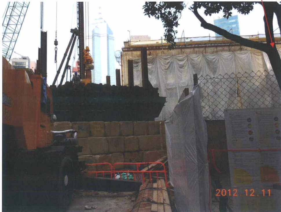
Fig. 4 Construction work in progress outside the cordon zone. T-6
