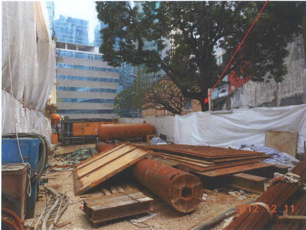
Fig. 7 Construction work in progress outside the cordon zone. T-7
