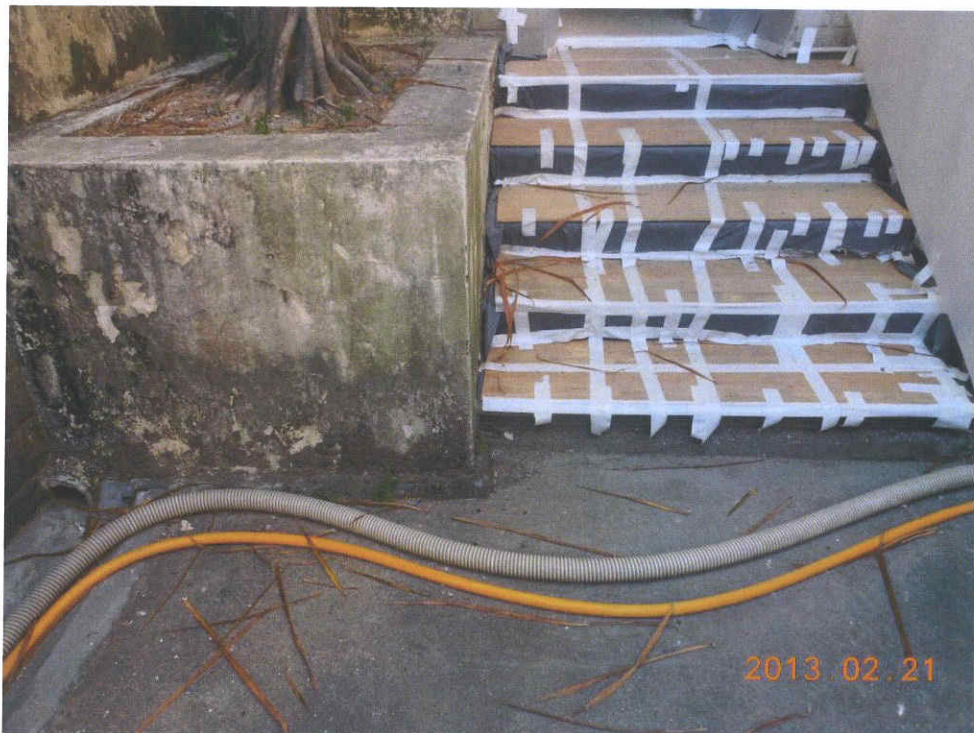
Fig. 3 Cleanliness of the site inside the cordon zone is acceptable.
