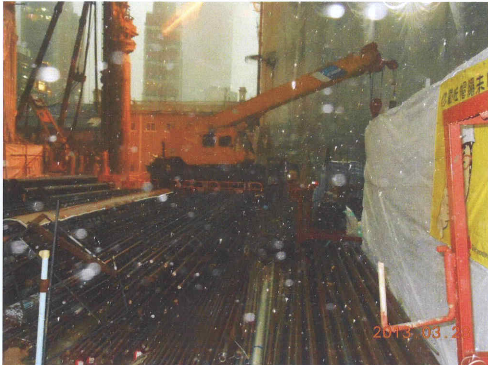
Fig. 4 Construction works in progress outside the cordon zone.
