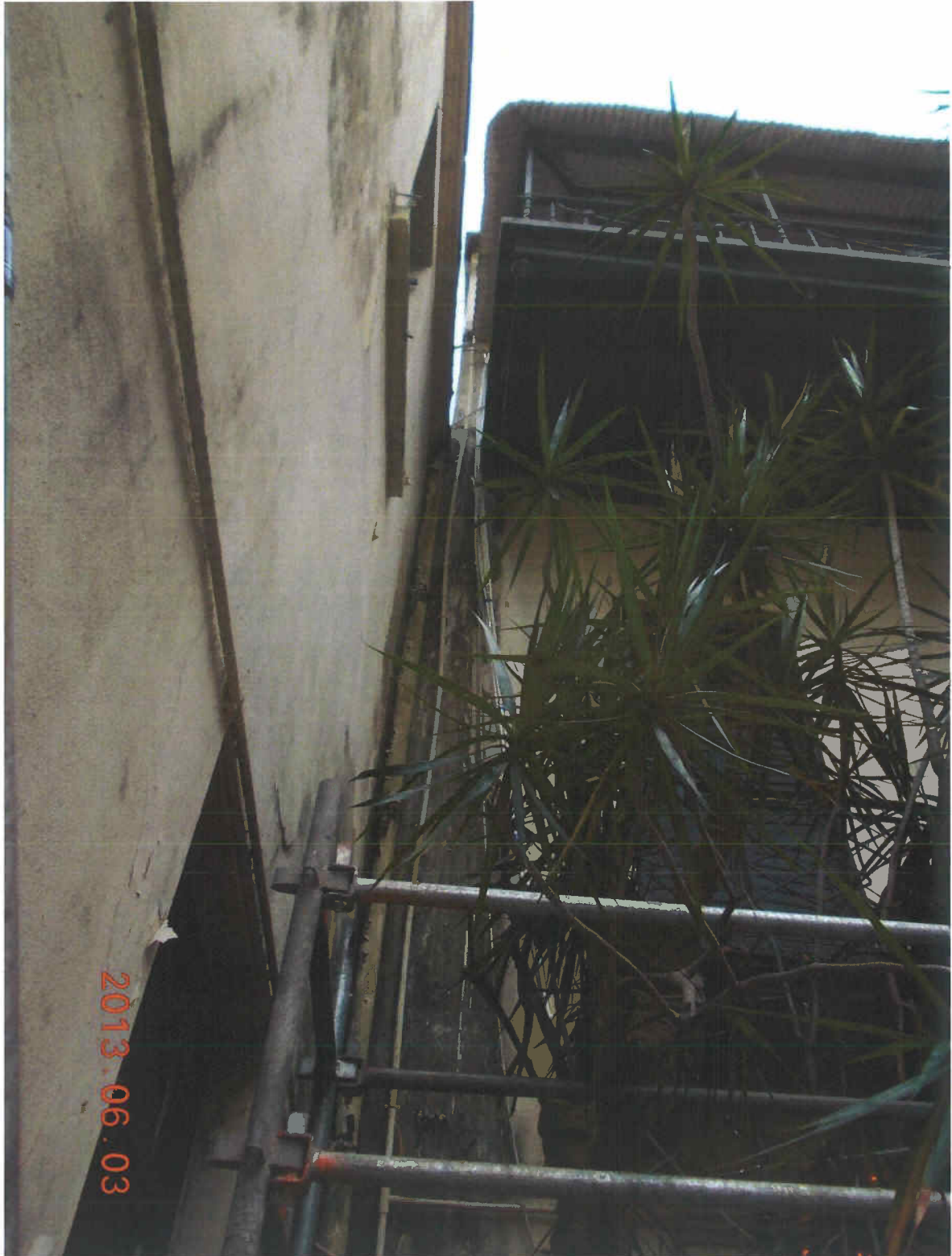
Fig. 5 Overall view of Tree-11 after provision of wrapping service.
