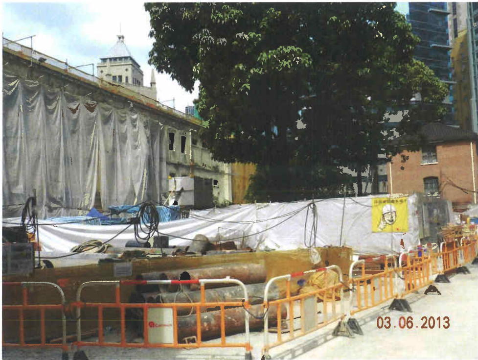
Fig. 6 Construction work in progress outside the cordon zone.
