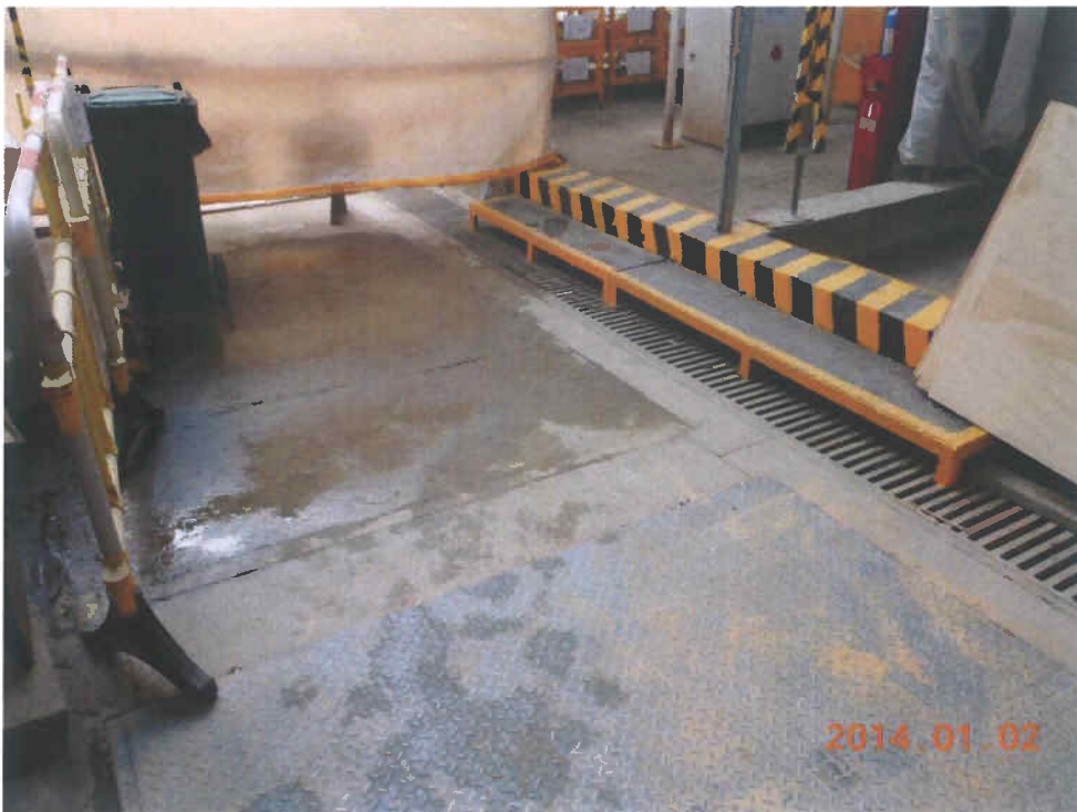
Fig. 11 The site outside the cordon zone is clean and tidy.
