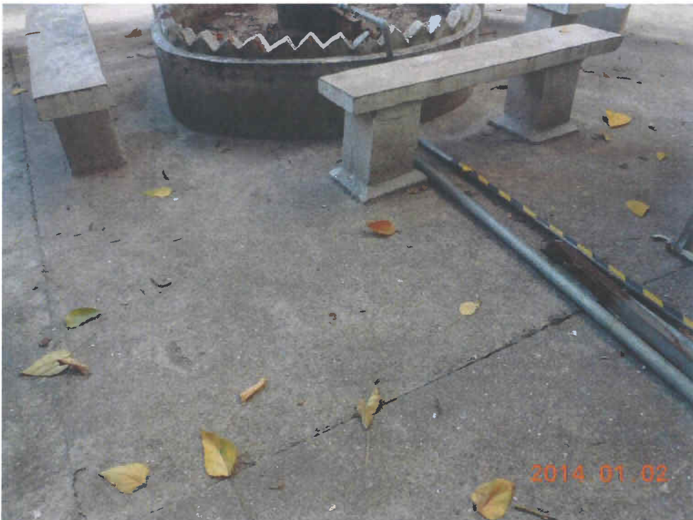
Fig. 3 Cleanliness of the site near the tree is acceptable.
