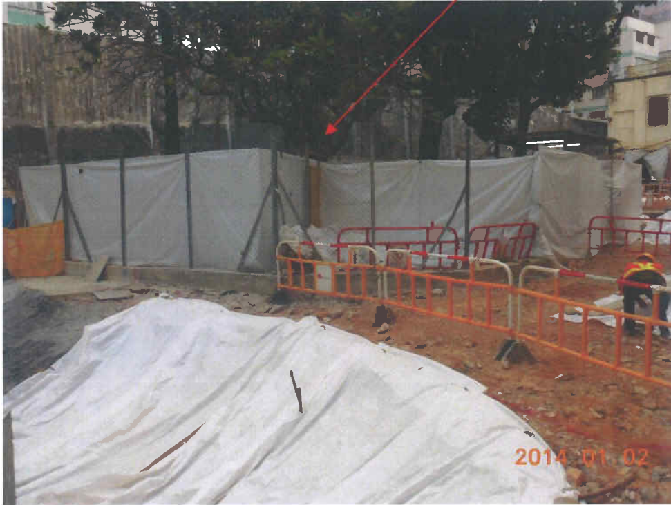
Fig. 6 Construction work has commenced near Tree-8.
