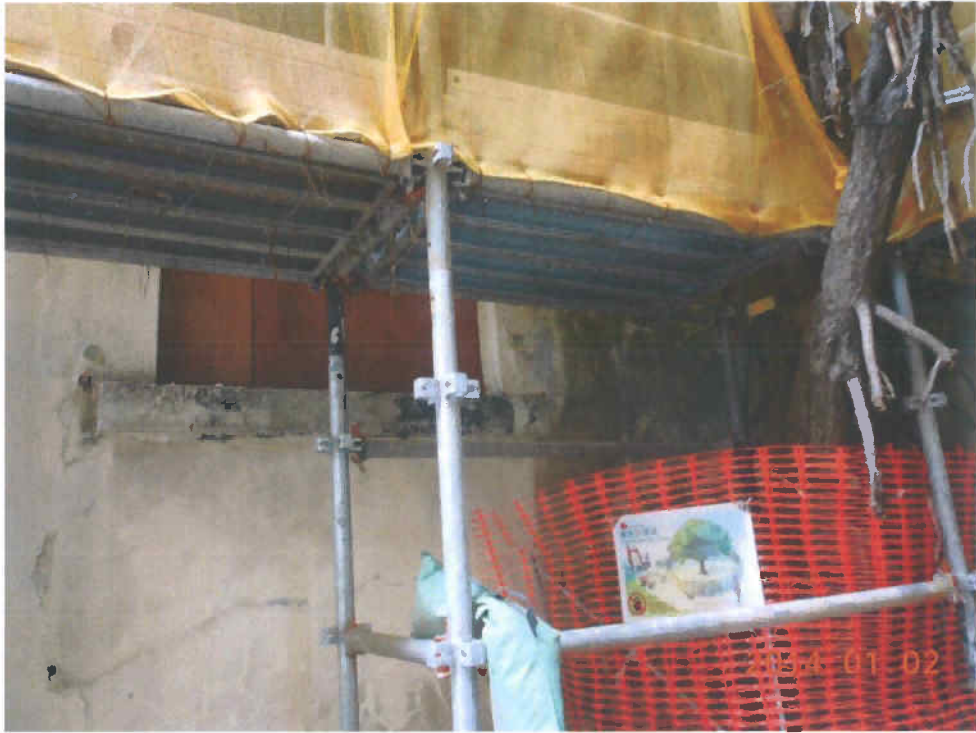
Fig. 6 The scaffold is still at site for renovation work.
