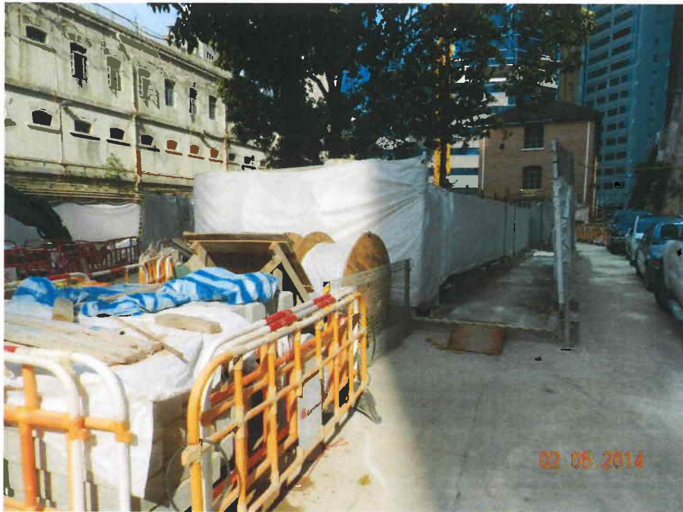
Fig. 8 The site outside the cordon zone is clean and tidy.
