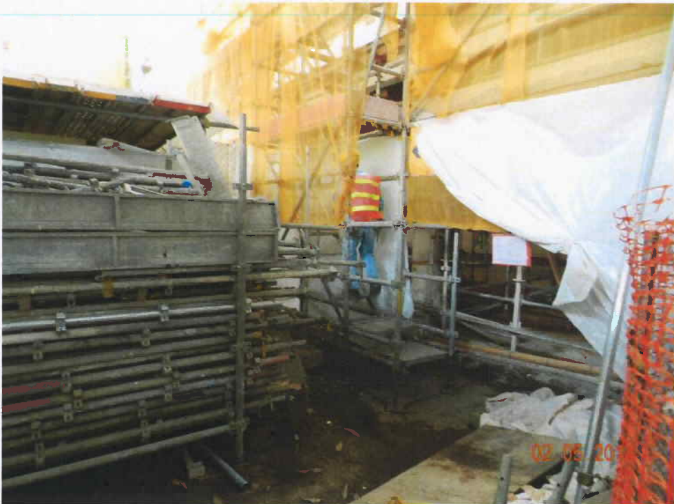
Fig. 5 Renovation works are in progress near the tree.
