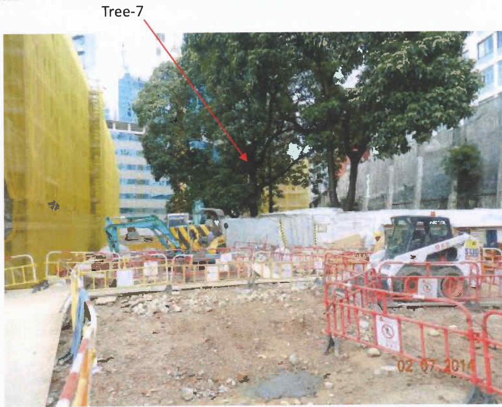
Fig. 8 Construction works are in progress outside the cordon zone.
