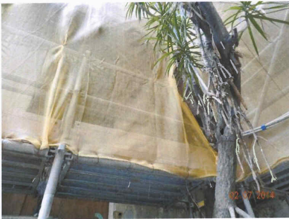
Fig. 7 Renovation works are in progress near the tree.
