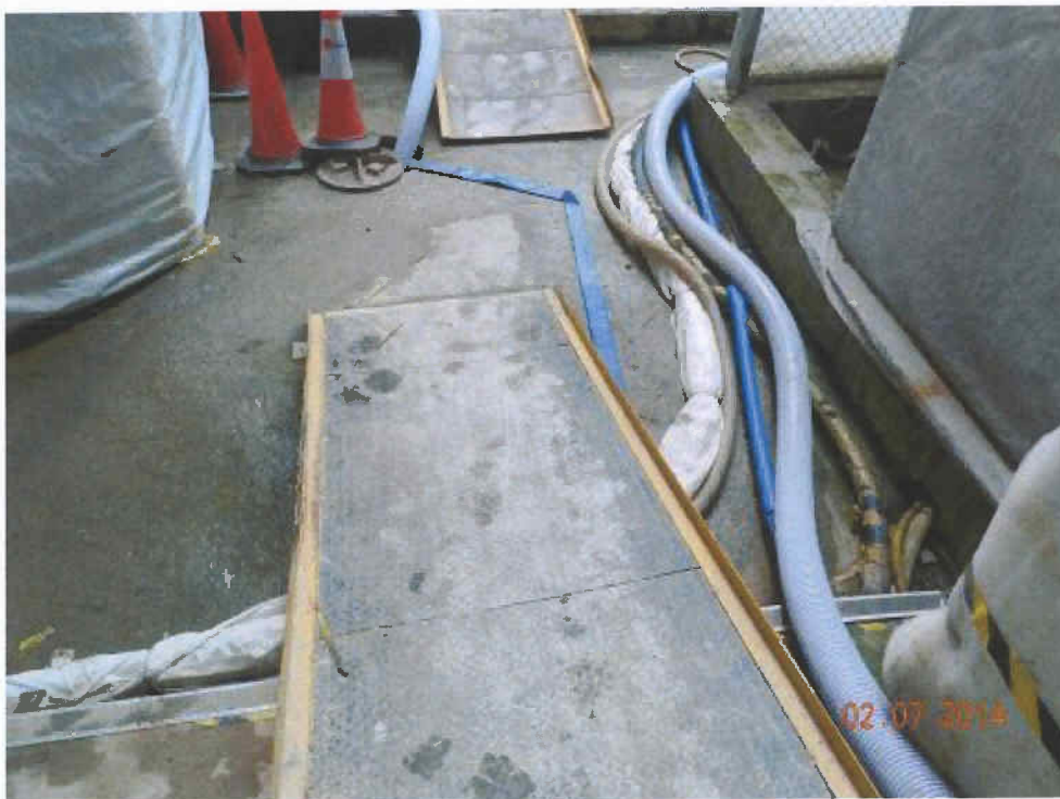
Fig. 9 The site outside the cordon zone is clean and tidy.
