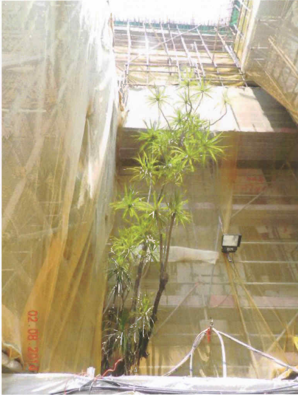
Fig. 10 Overall view of Tree-11 during inspection on 2 nd August 2014.
