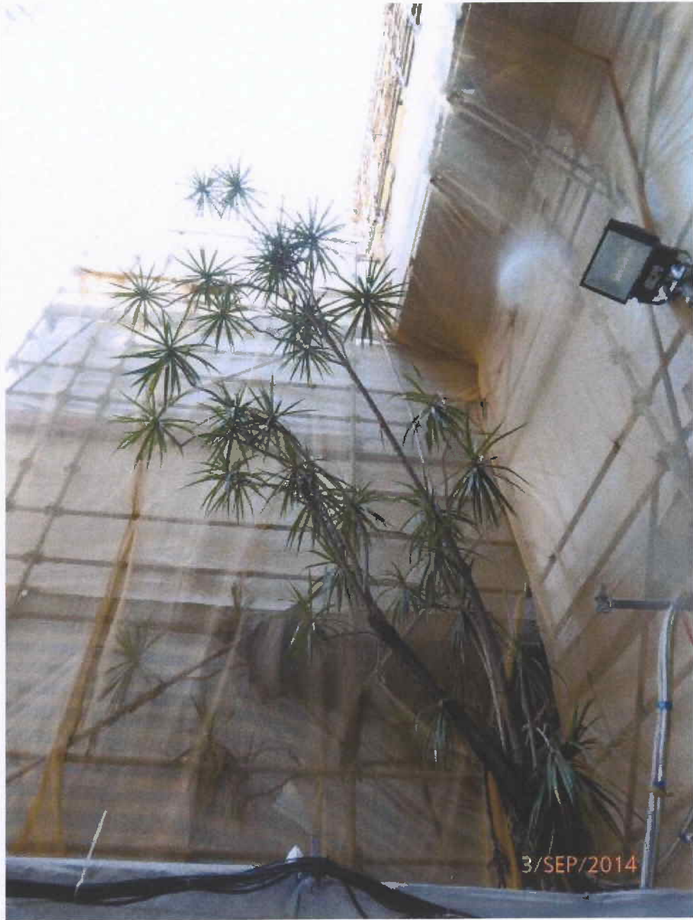
Fig. 10 Overall view of Tree-11 during inspection on 3 rd Sept. 2014.
