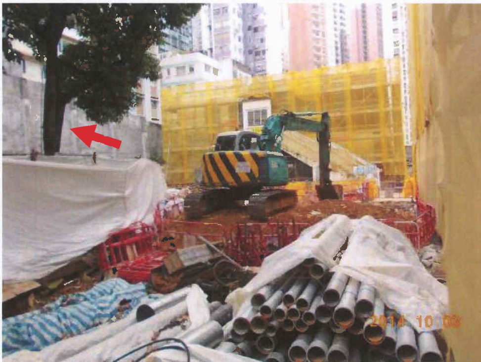
Fig. 9 Construction works are in progress outside the cordon zone.
