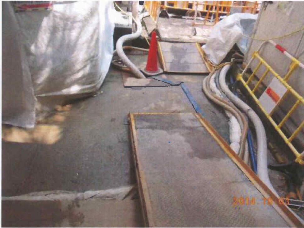
Fig. 10 Cleanliness of the site outside the cordon zone is acceptable.
