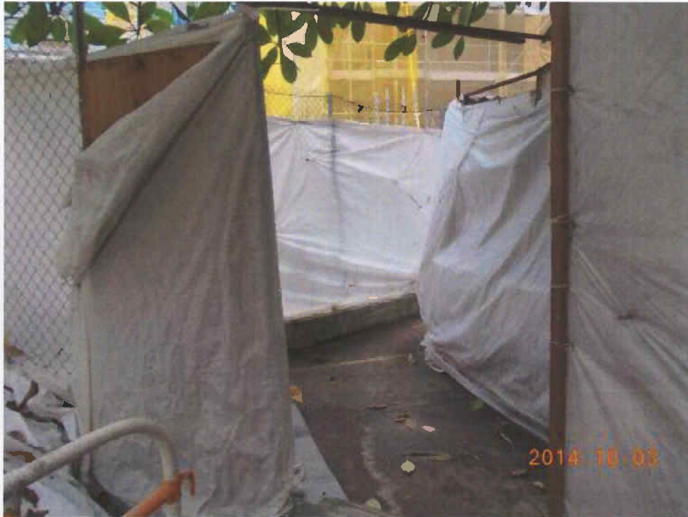
Fig. 8 Cleanliness of the access near Tree-8 is acceptable.
