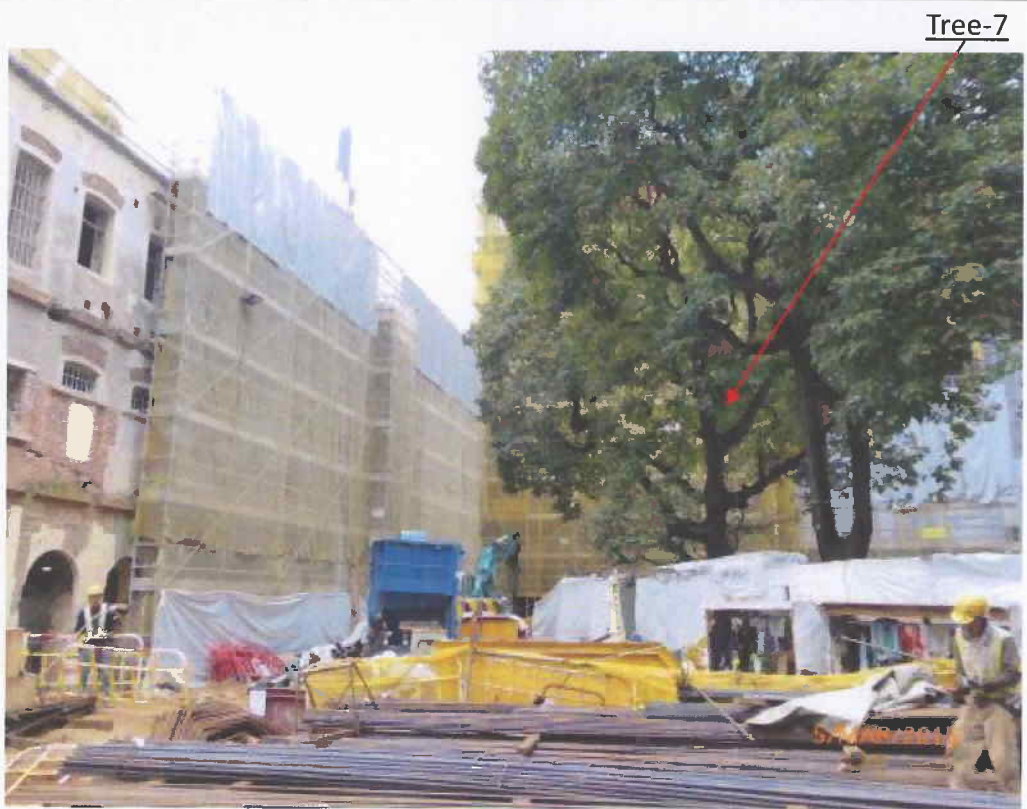
Fig. 11 Construction works are in progress outside the cordon zone.
