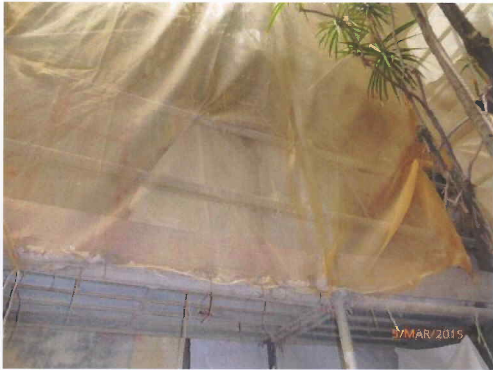
Fig. 8 Renovation work is in progress near the tree.
