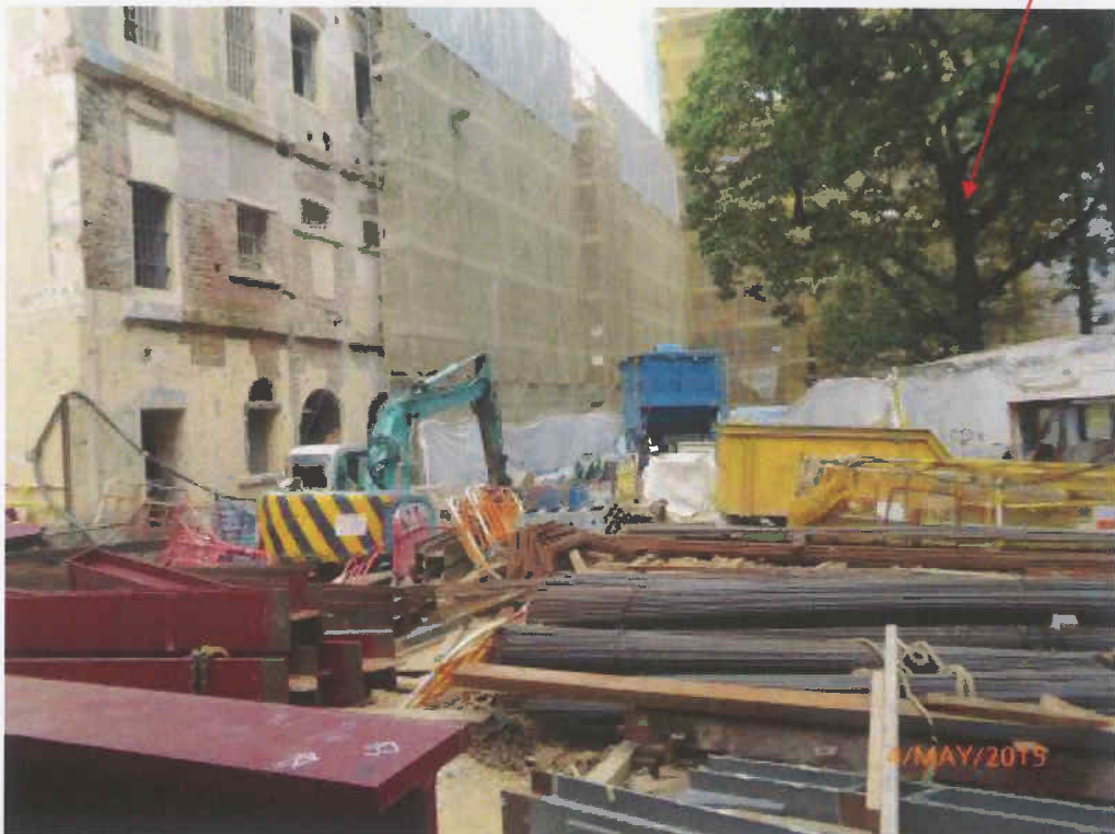
Fig. 11 Construction works are in progress outside the cordon zone. T-7
