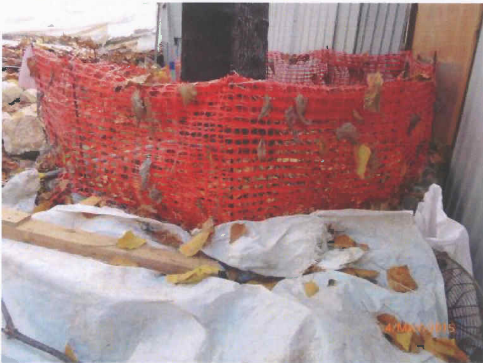
Fig. 7 The small cordon zone is in order.
