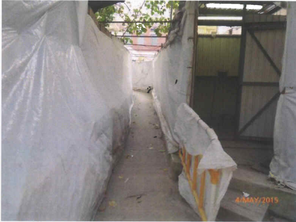
Fig. 10 Cleanliness of the access near Tree-7 is acceptable.
