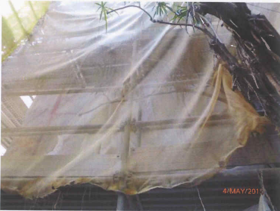
Fig. 9 Renovation work is in progress near Tree-11.
