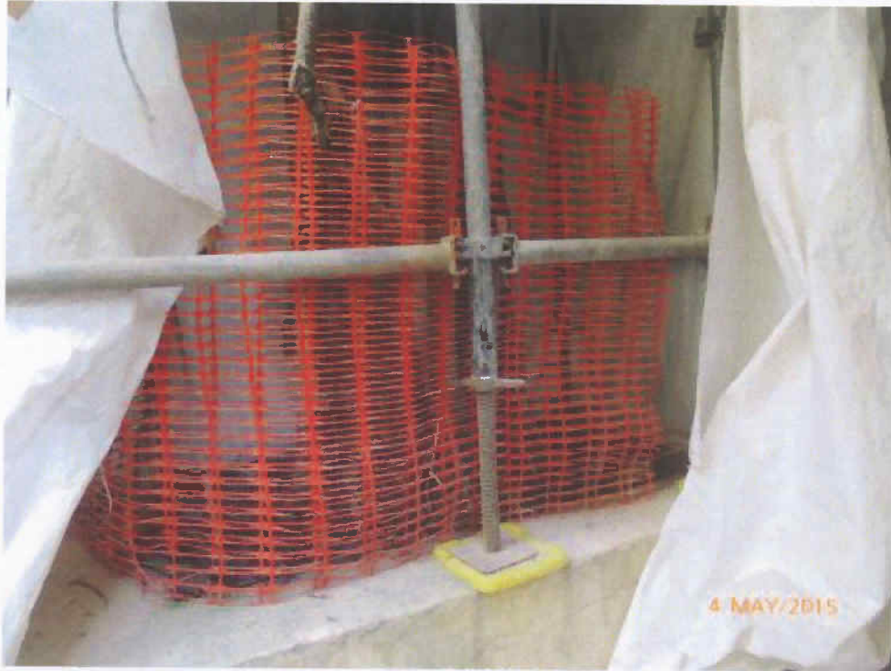
Fig. 8 The small cordon zone is in order.
