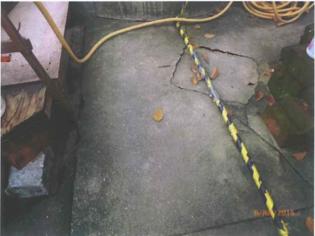
Fig. 9 The site near the planter is clean and tidy.
