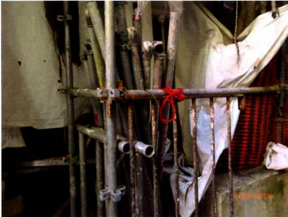
Fig. 8 Renovation works are in progress near the planter.
