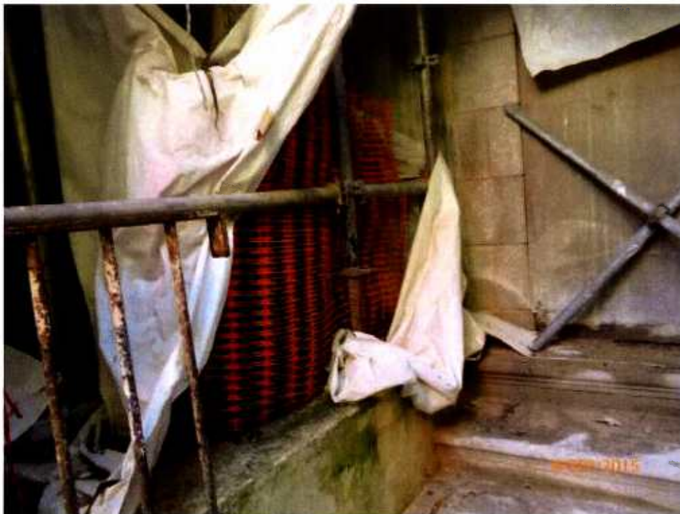
Fig. 9 The small cordon zone is in order.
