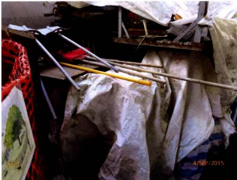
Fig. 9 Many construction items are placed near the tree.
