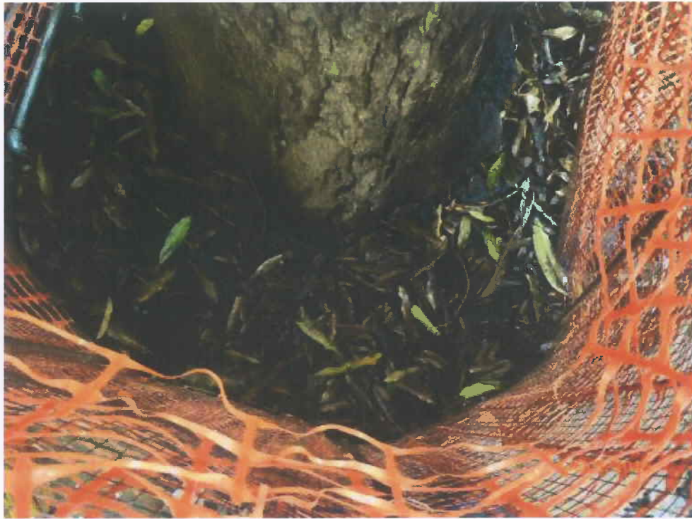
Fig 2. Root collar of Tree-5 is normal. The planter appears clean and tidy.
