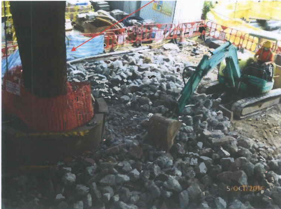
Fig. 8 Renovation work is in progress near Tree-5.
