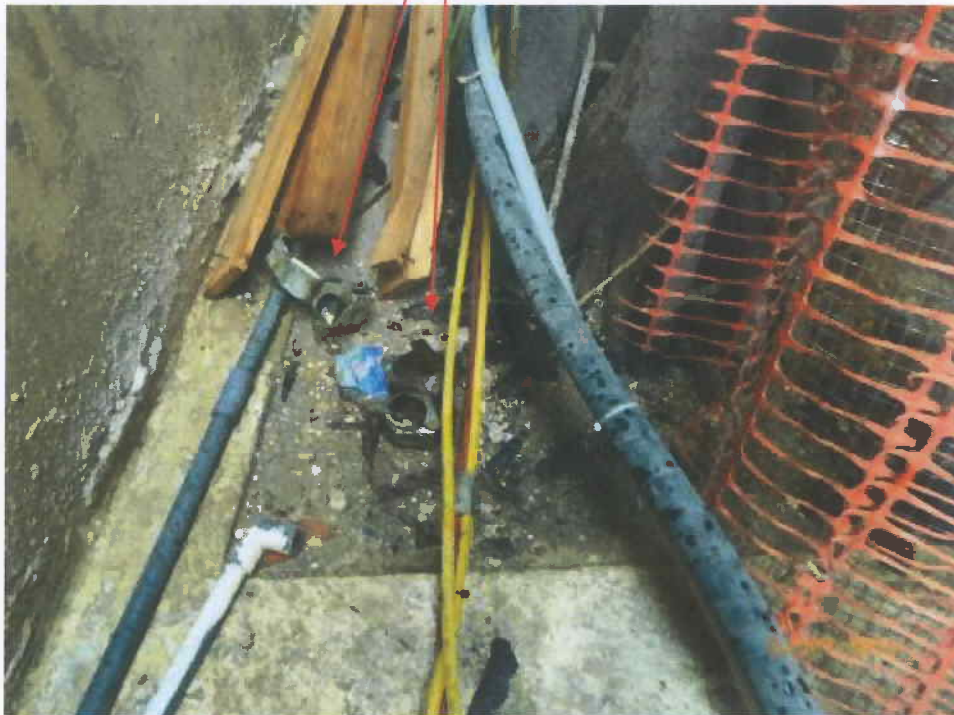
Fig. 3 Lots of construction debris are found on the bottom part of the tree.
