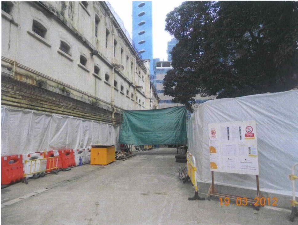
Fig. 5 Demolition works in progress outside the cordon zone.
