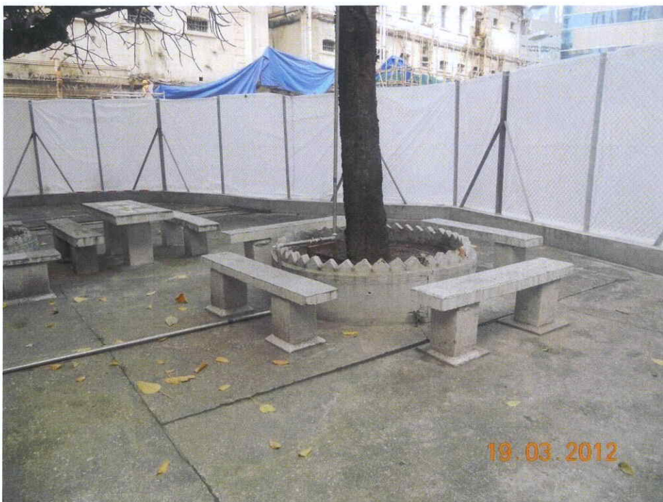
Fig. 3 The site keeps clean and tidy at the time of inspection.
