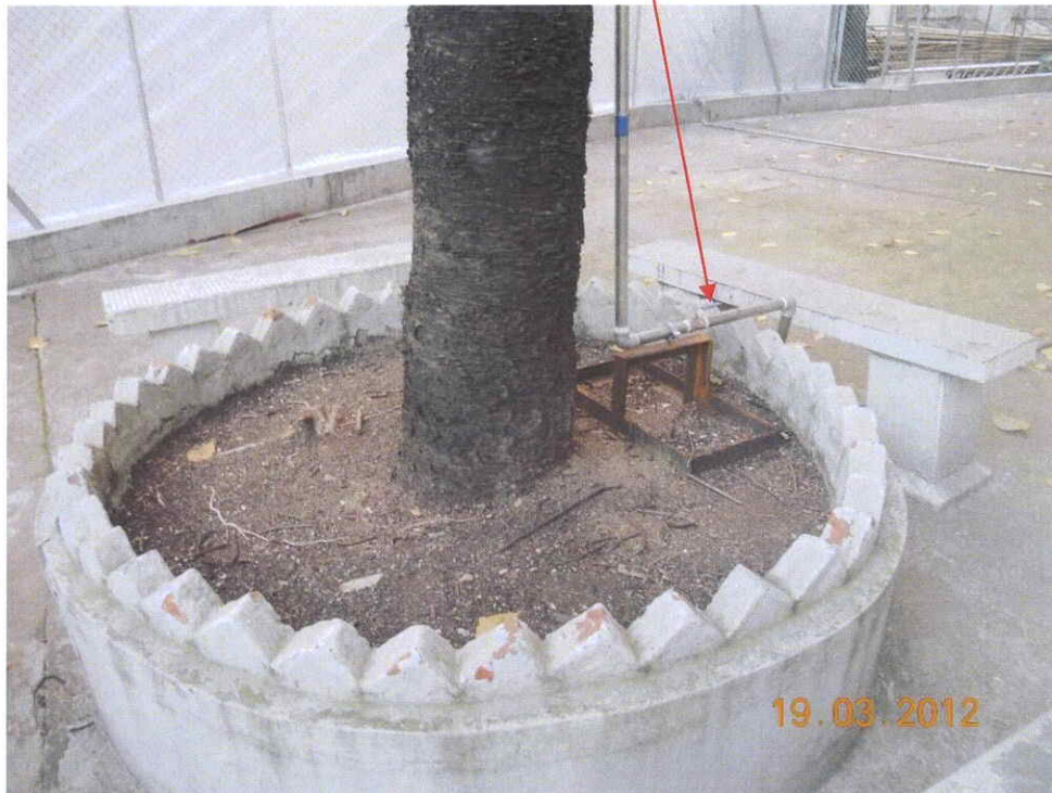
Fig 2. The planter is clean and tidy. Irrigation system has been installed for the tree.
