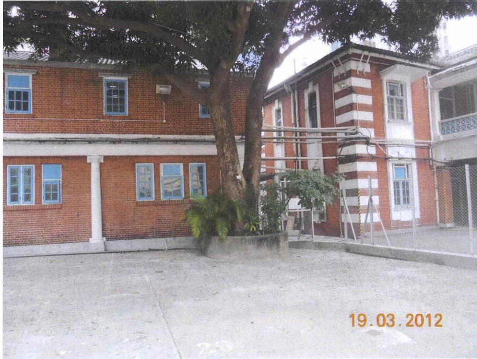
Fig. 4 Cordon zone appears clean and tidy.
