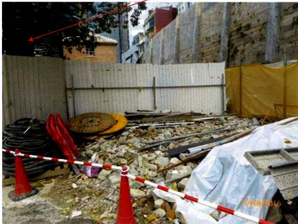
Fig. 11 Construction works are in progress near Tree-6.
