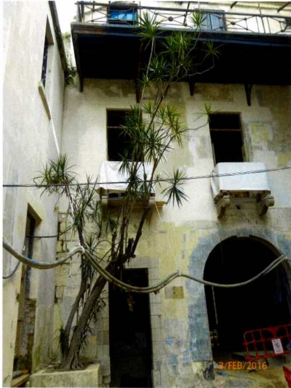
Fig. 12 Overall view of Tree 11 during inspection on 3 rd February 2016.
