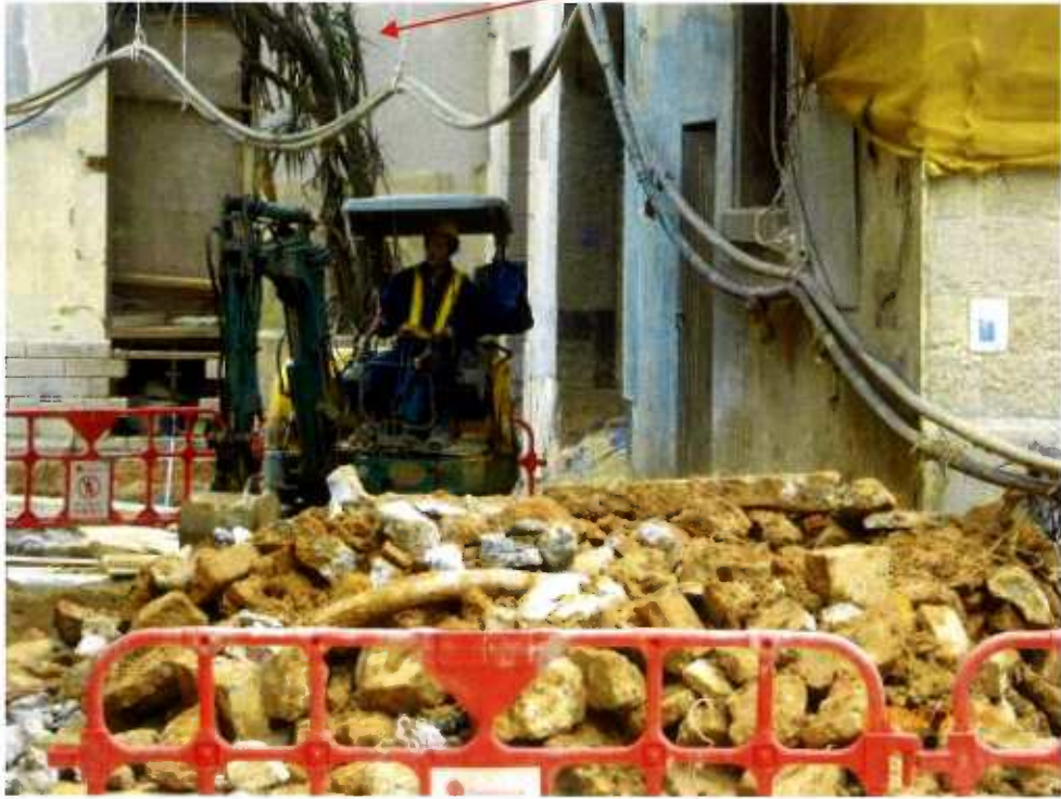
Fig. 10 Construction works are in progress in front of the tree.
