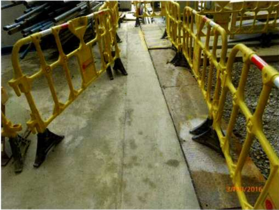
Fig. 10 The access near Tree-5 appears clean and tidy.
