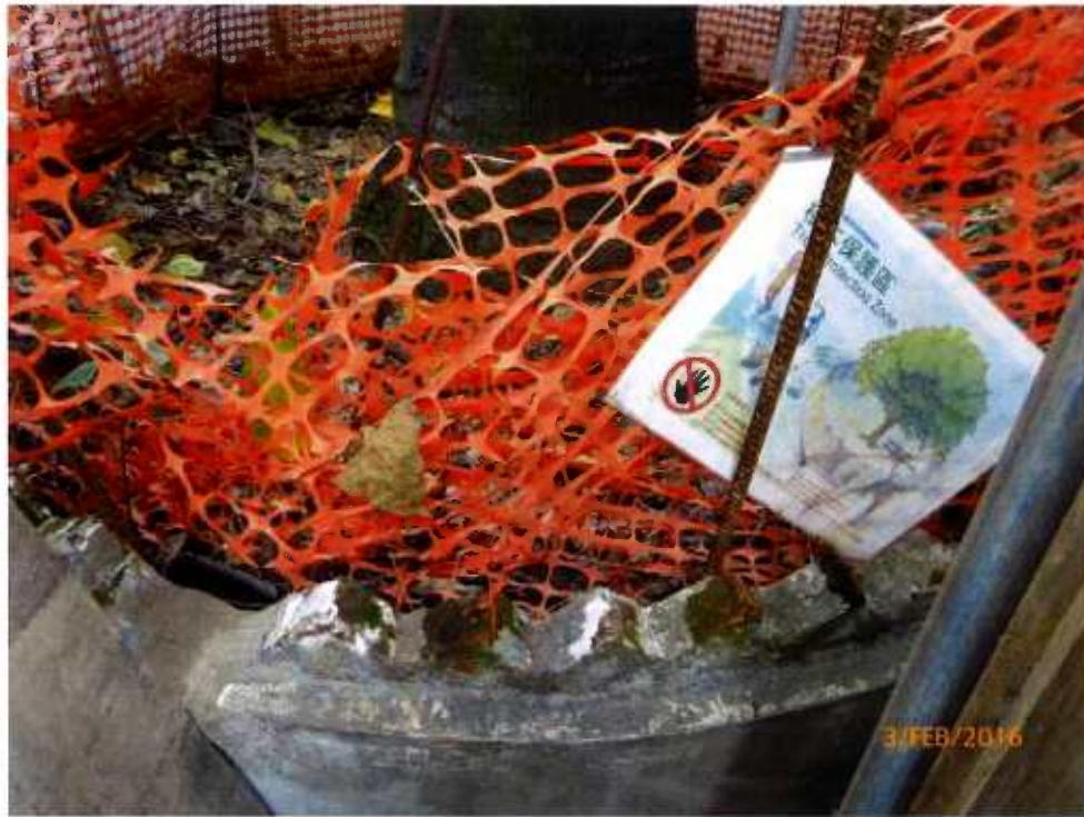
Fig. 8 The small cordon zone is in order.
