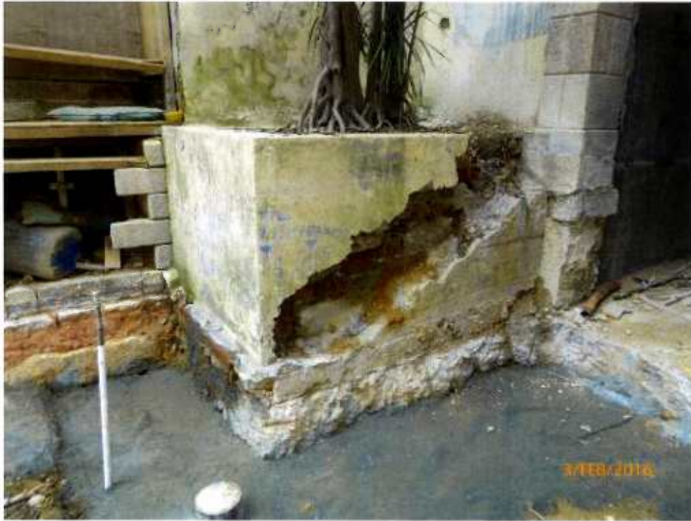
Fig. 8 The site near Tree 11 is under renovation.
