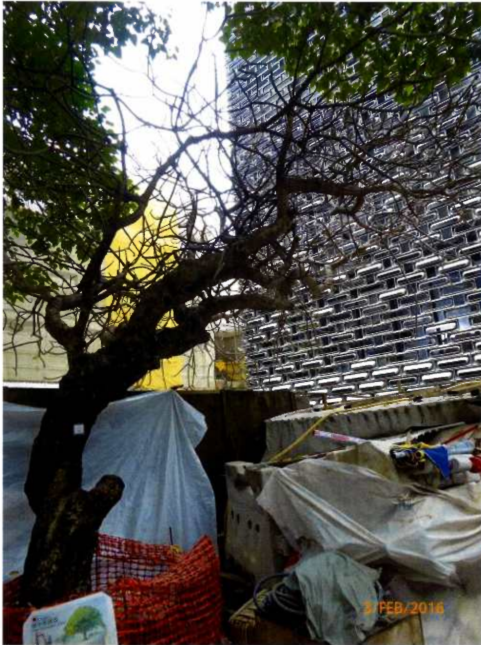
Fig. 12 Overall view of Tree-8 during inspection on 3 rd February 2016.
