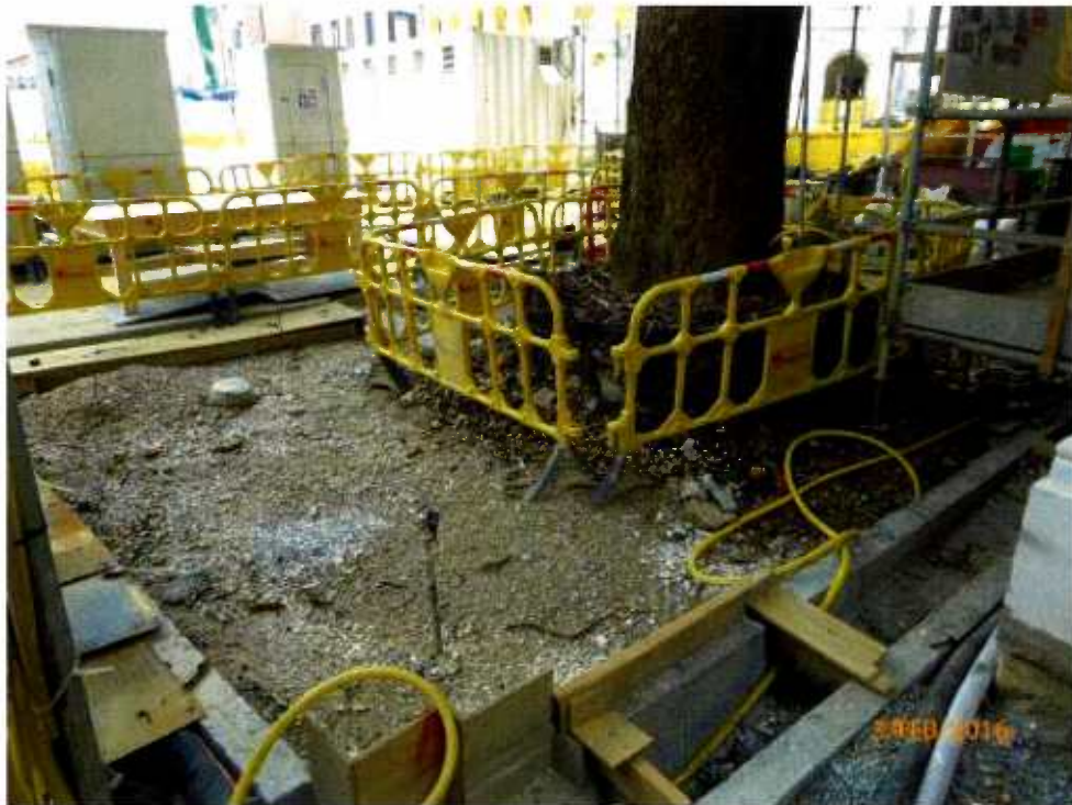
Fig. 9 The site near Tree 5 is under renovation.
