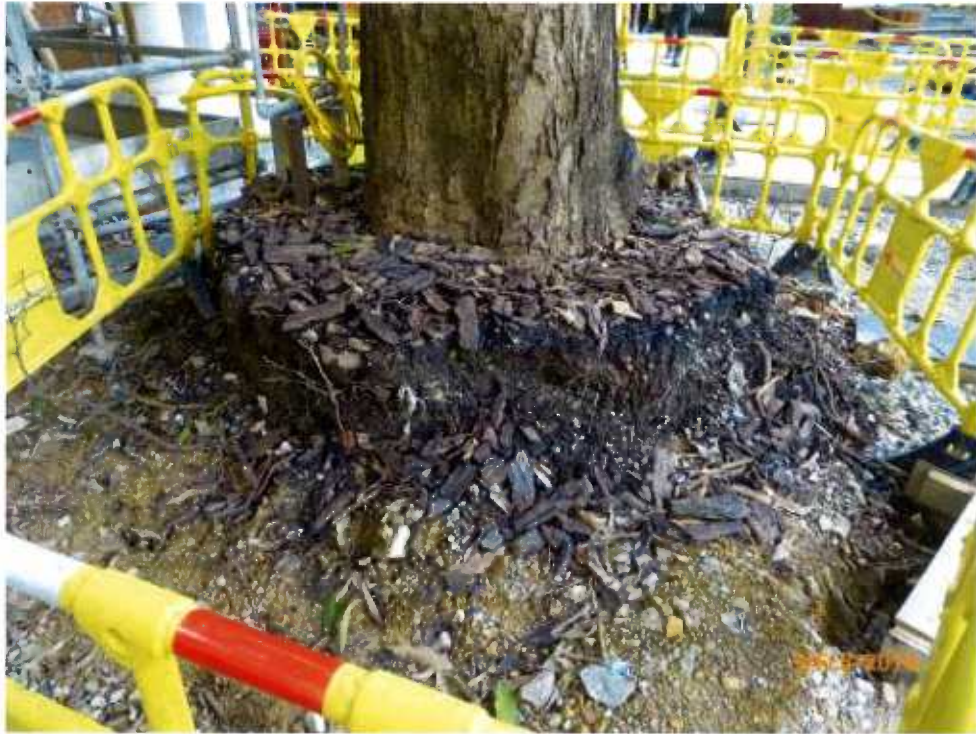
Fig 2. Root collar is normal. The planter is being re-built.
