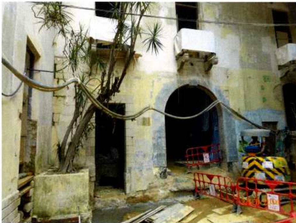
Fig. 9 The nearby buildings also are under renovation.
