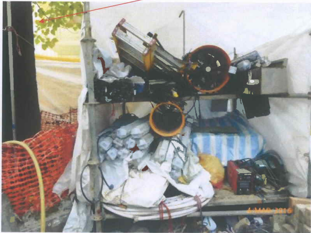
Fig. 10 Some construction tools are placed near Tree-7 .
