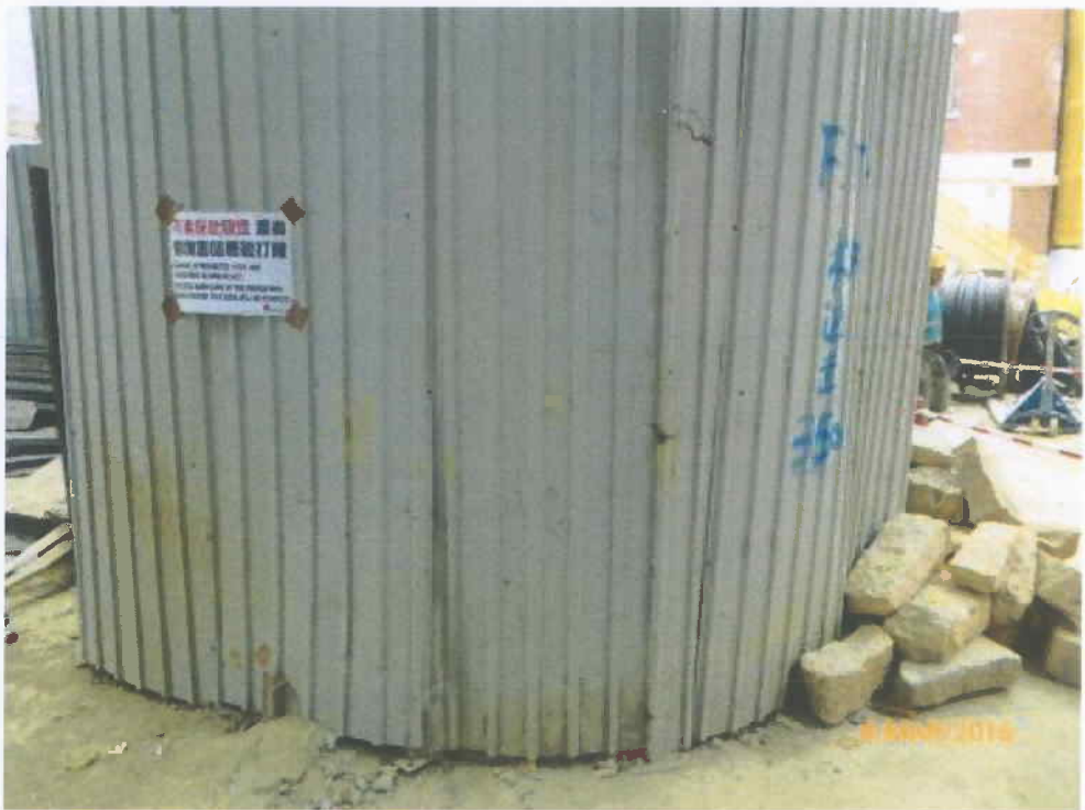
Fig. 9 Several metallic sheets surrounded the planter to act as a cordon zone.
