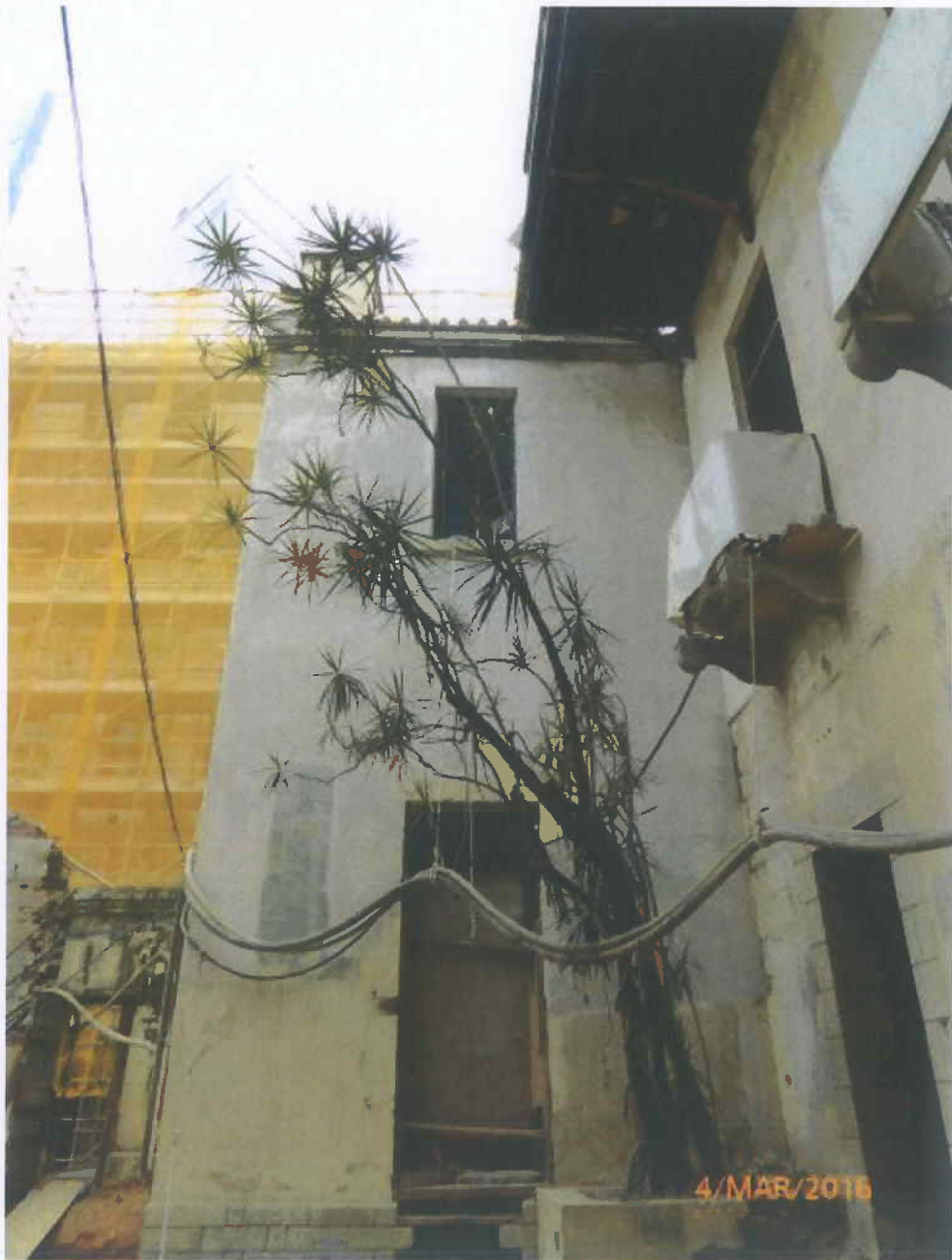
Fig. 12 Overall view of Tree 11 during inspection on 4 th March 2016.
