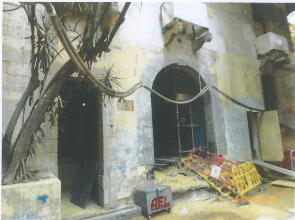
Fig. 9 The nearby buildings also are under renovation.
