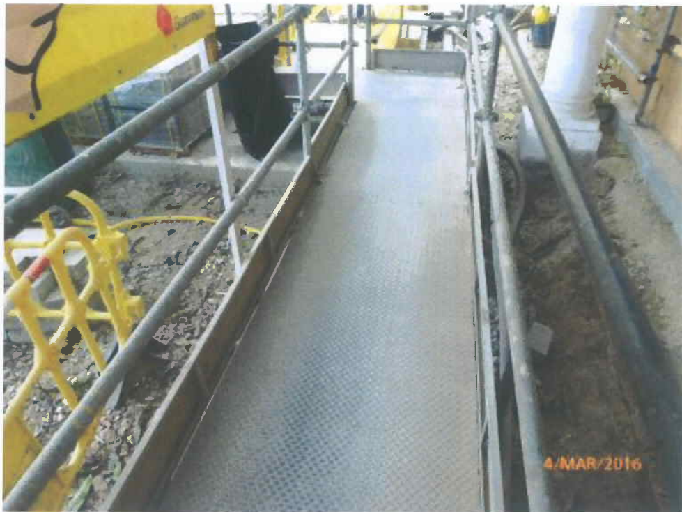
Fig. 12 The access near Tree-5 appears clean and tidy.
