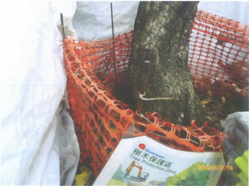
Fig. 7 The small cordon zone is in order.
