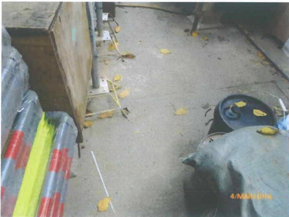
Fig. 9 Cleanliness of the site near Tree-8 is acceptable.
