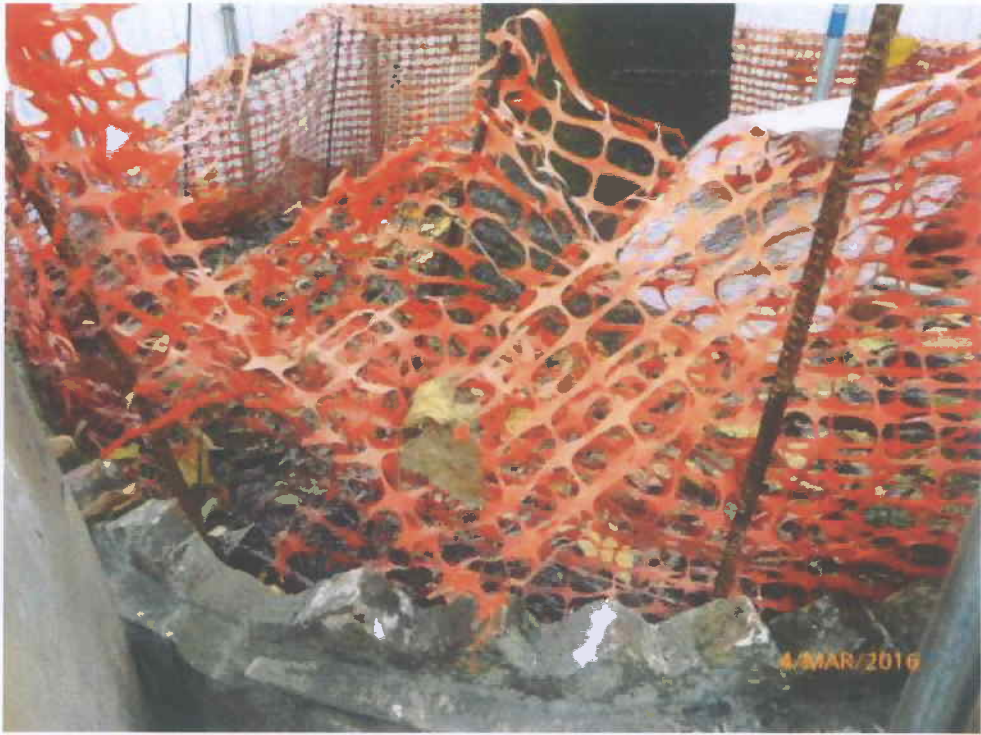
Fig. 8 The small cordon zone is in order.
