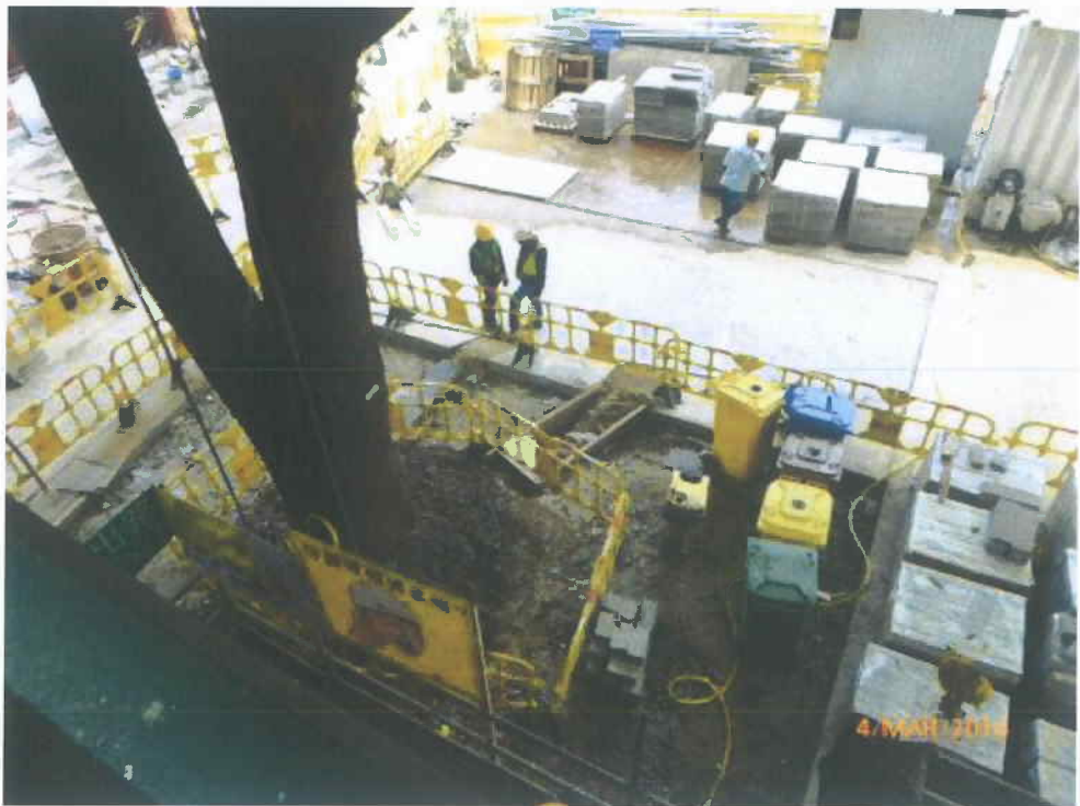
Fig. 11 Renovation work is in progress near the tree.
