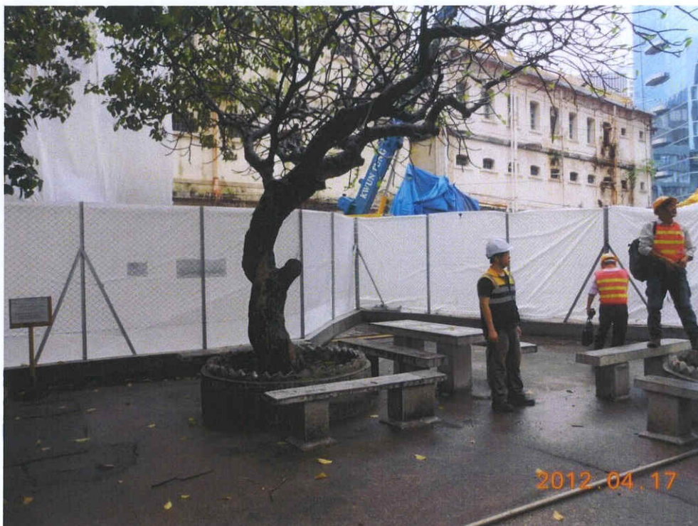
Fig. 3 Cordon zone appears clean and tidy.
