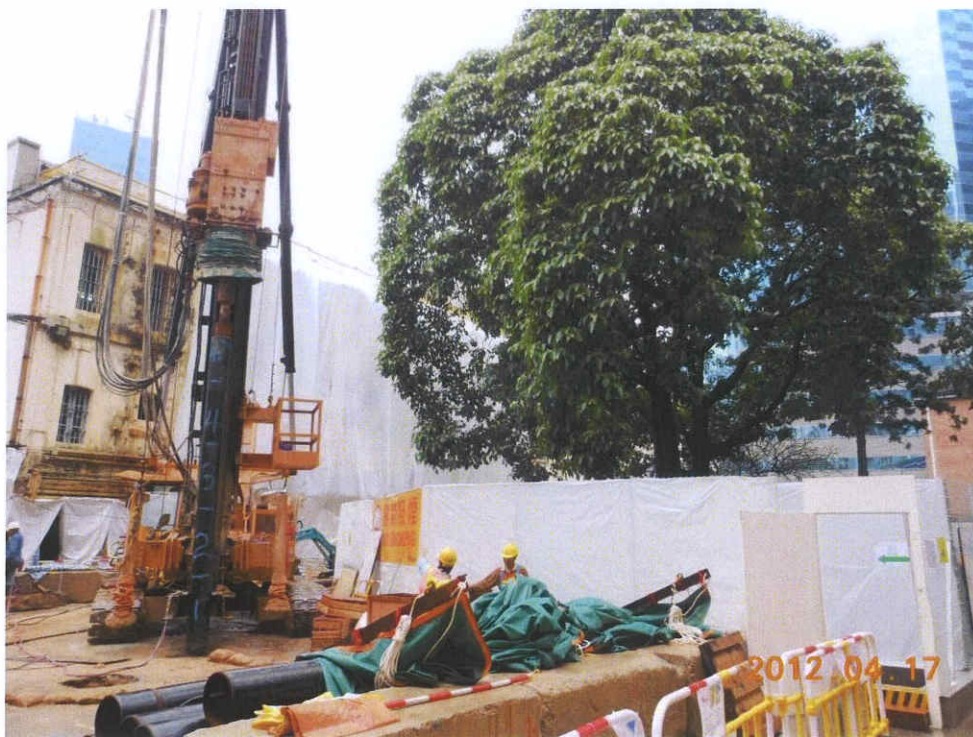
Fig. 5 Construction works commence near the cordon zone.
