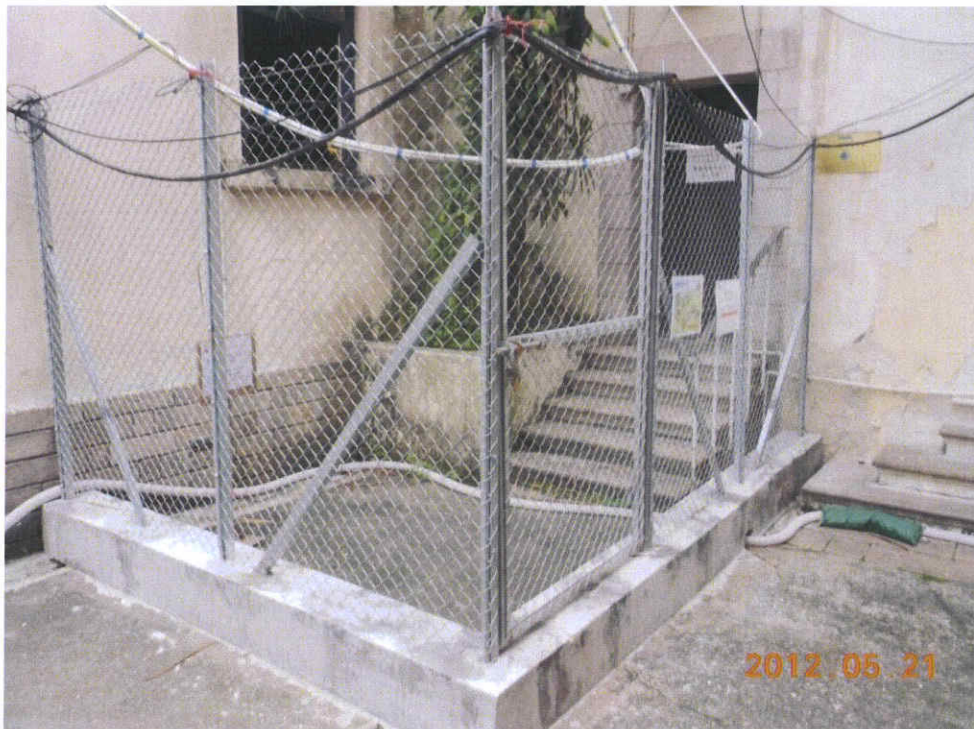
Fig. 3 Two doors are properly locked and restrict admittance to the cordon zone.
