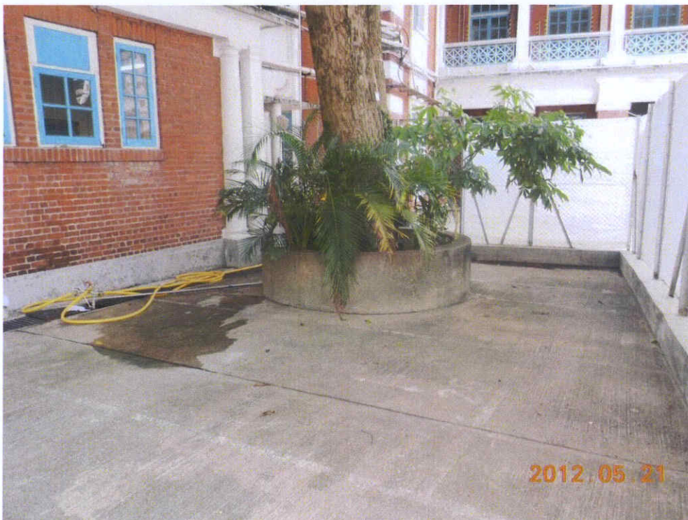
Fig. 3 The cordon zone appears clean and tidy at the time of inspection.
