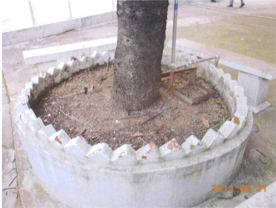
Fig 2. The planter appears clean and tidy at the time of inspection.
