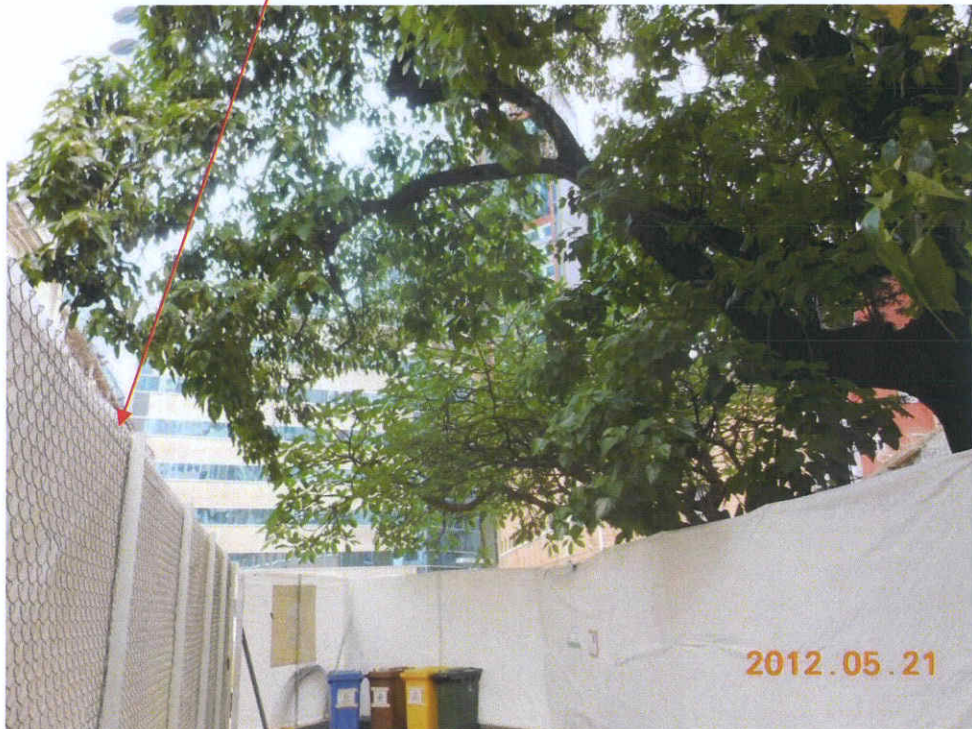
Fig. 5 One more fence has been erected to protect the passers-by.
