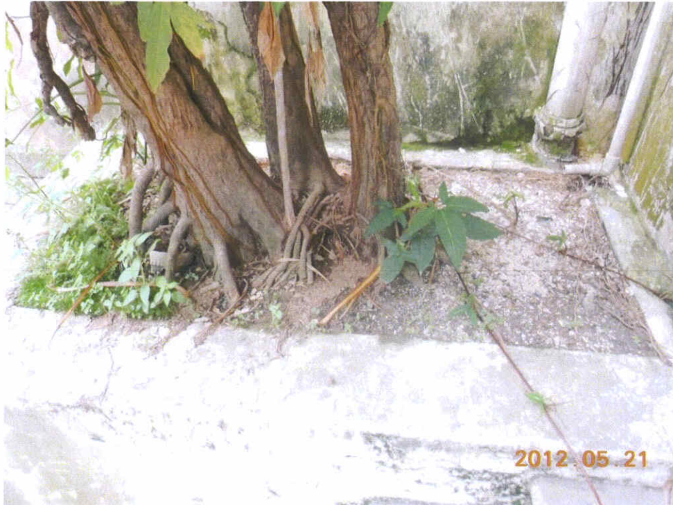
Fig. 2 Cleanliness of the planter is acceptable at the time of inspection.
