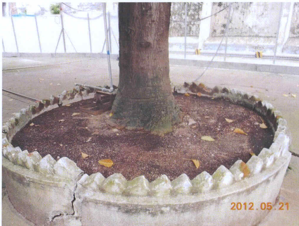
Fig. 3 The planter appears clean and tidy at the time of inspection.
