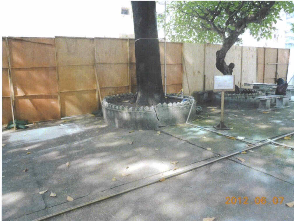
Fig. 4 The site is clean and tidy at the time of inspection.
