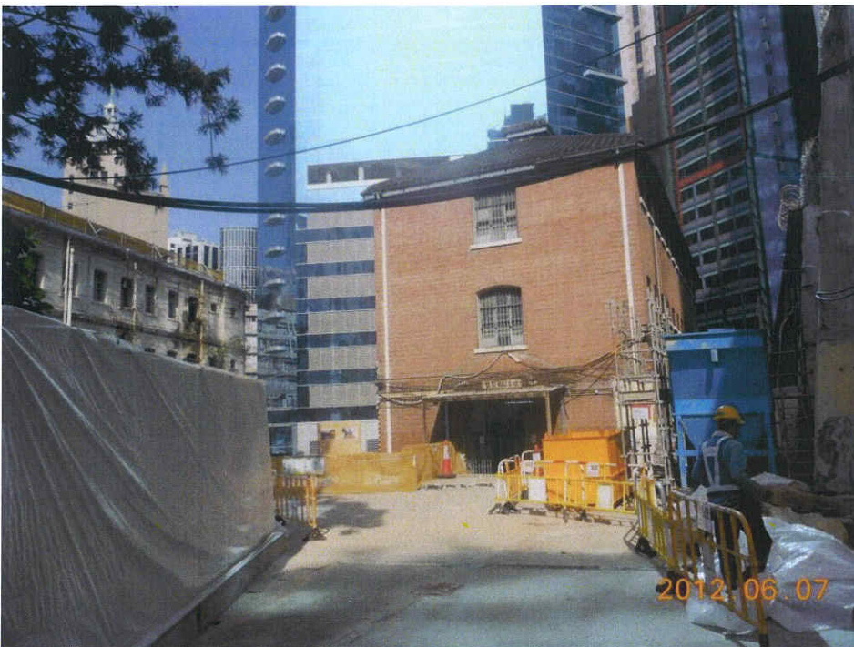
Fig. 5 Construction works are in progress outside the cordon zone.
