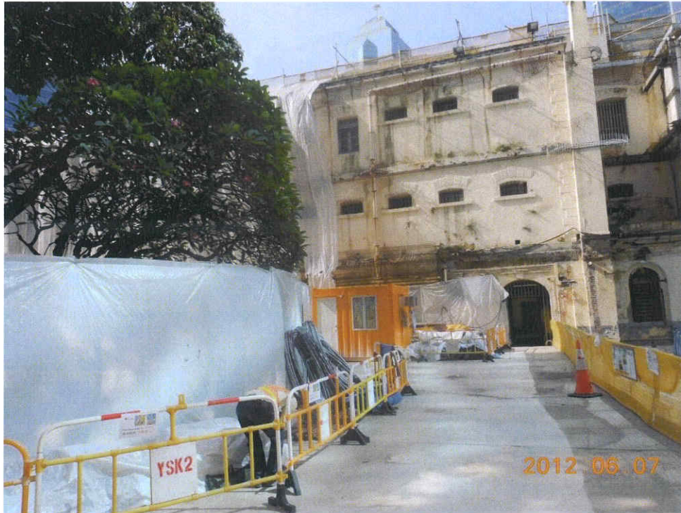
Fig. 4 Area outside the cordon zone is clean and tidy.
