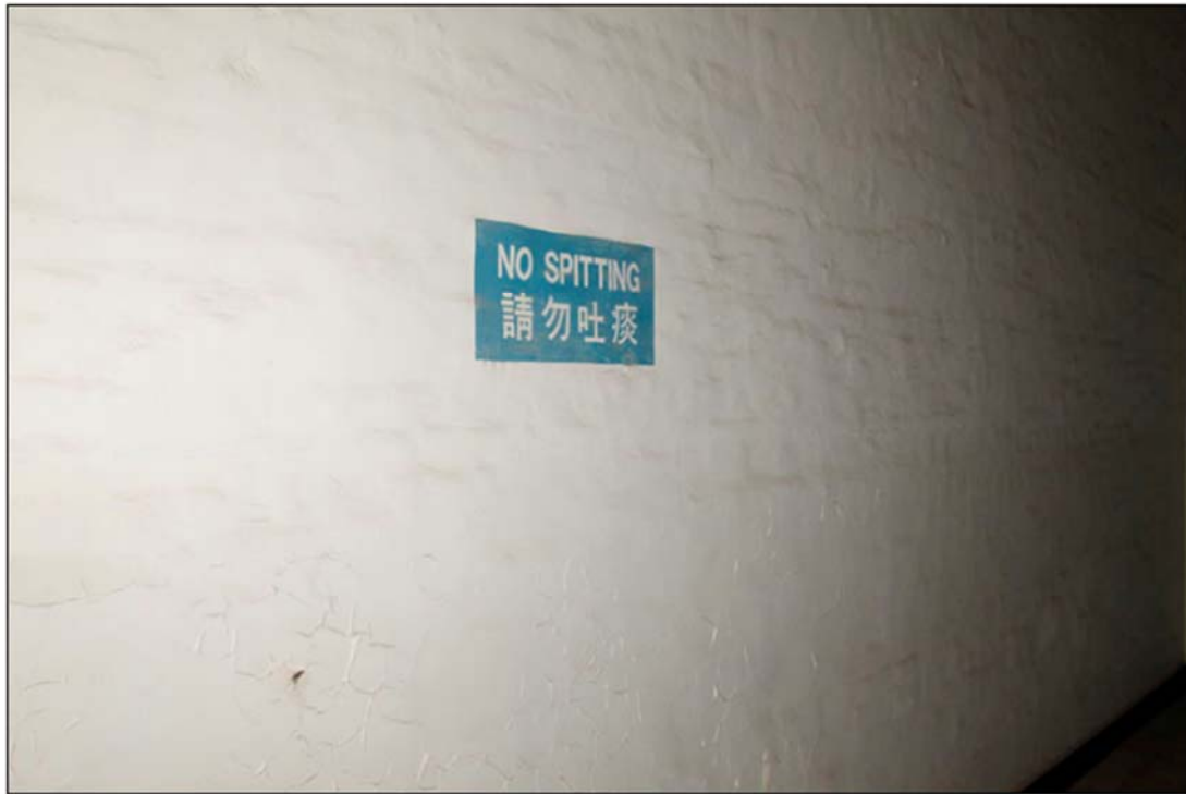
Photo 03-2F-230 General view of the wall (21-3-2012)
