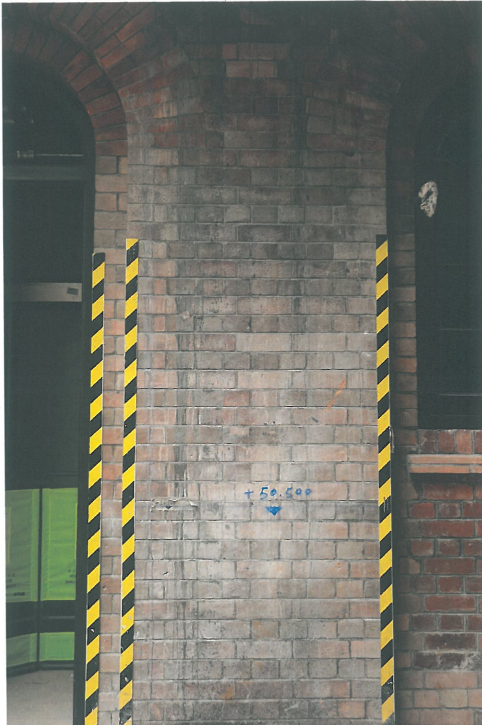
Above, photo taken on 18 th March 2016, showing spilt concrete on the Block 9 Magistracy West elevation (G/F).
