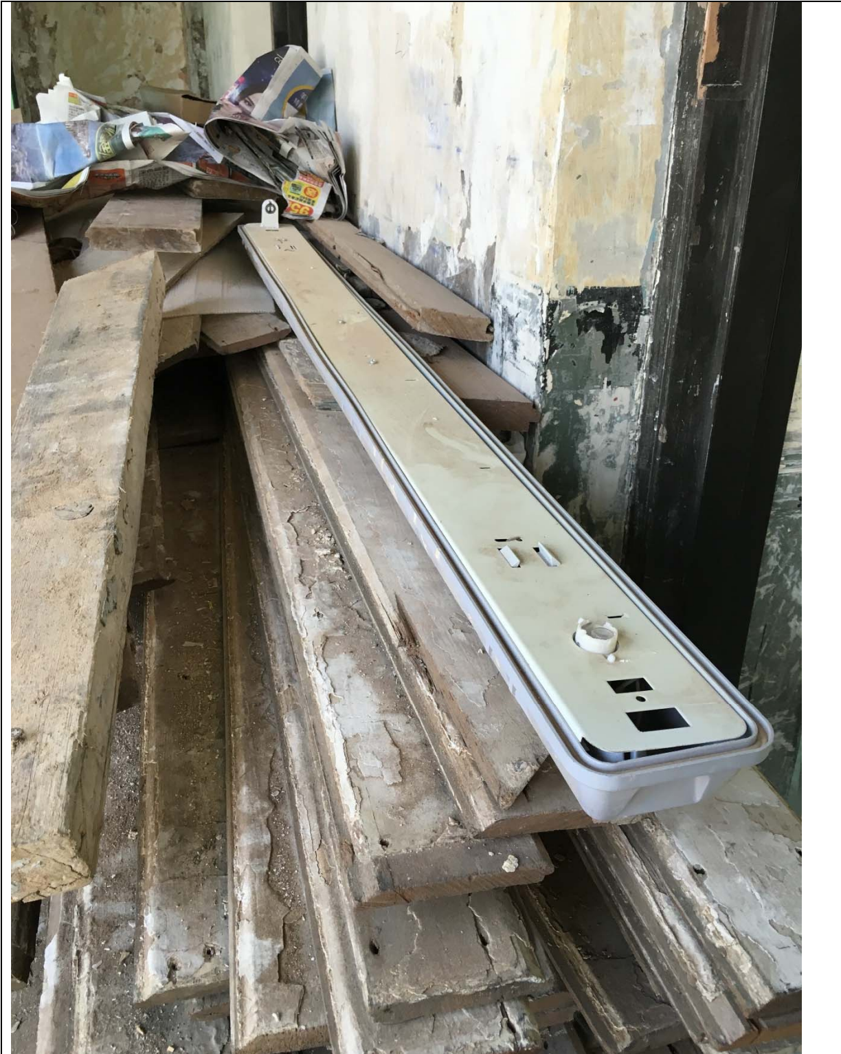
Above, photograph taken on 2 nd March, 2016, showing timber boarded ceiling was stored inappropriately with trashes.
