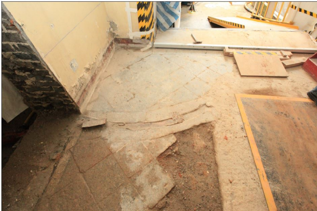
Photograph taken on 22 nd August 2013 by the Management Contractor, showing the track on the granite flagstone at the East entrance.
