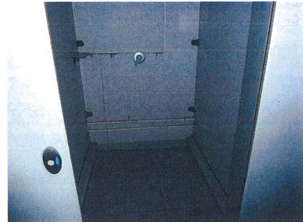
Photo 4. Hot water pipes supplying to the showers were selected for inspection
