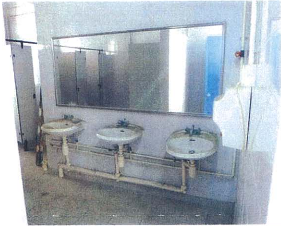
Photo 1. Hot water pipes supplying to the sinks were selected for inspection
