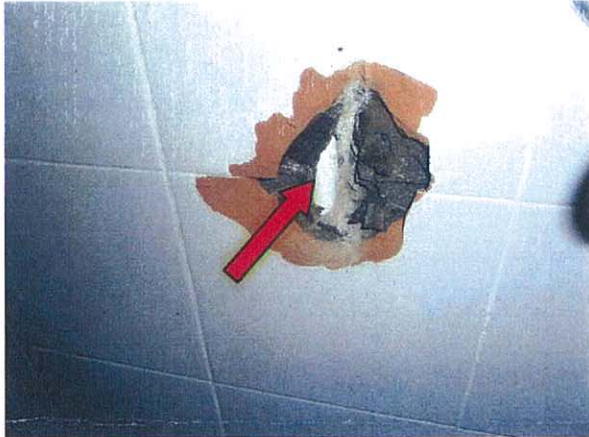
Photo 7. Embedded pipe was insulated with uPVC material
