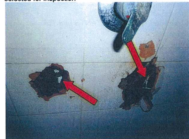
Photo 6. Embedded pipes were insulated with uPVC material
