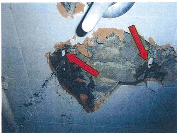
Photo 5. Embedded pipes were insulated with uPVC material
