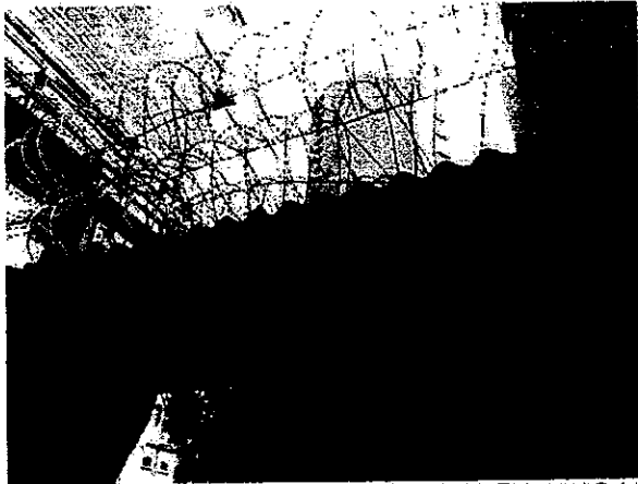
Photo 21. ACM Corrugated Sheet (Type 2) at the Entrance Gate, G/F of Block 17 (Photo taken on 20 Oct 2011).
