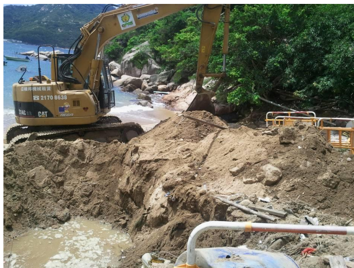
Photo 1: Excavation work was carried out on 25 June 2012 for cable laying.
