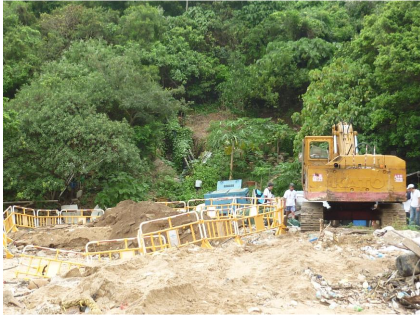
Photo 1: Excavation work was carried out on 5 July 2012 for cable laying.
