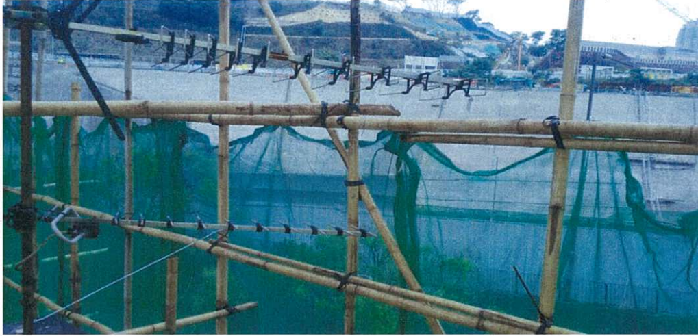
Figure 1a View from No. 21 Valley Road (to HOM work site)
