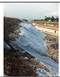
Capping of the PFA is established to prevent spreading in air.
