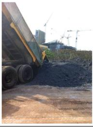
The PFA excavated has been dehydrated under sunlight, and will be buried back to its original position inside the site boundary.
