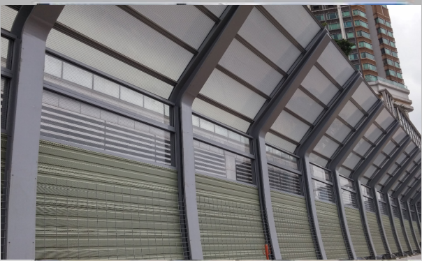
Image of Cantilever Barrier (under construction)
