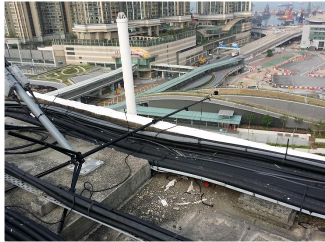
Photo 2 : Man King Building (R/F position)
