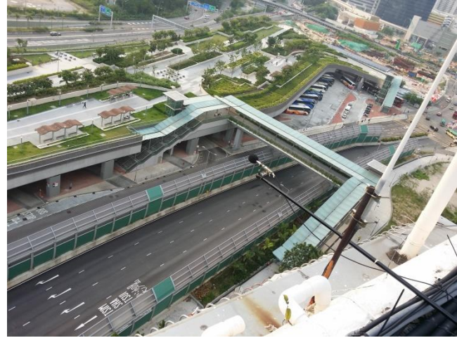
Photo 2 : Man King Building (R/F position)
