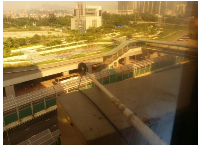
Photo 4 : Man King Building (10/F position)
