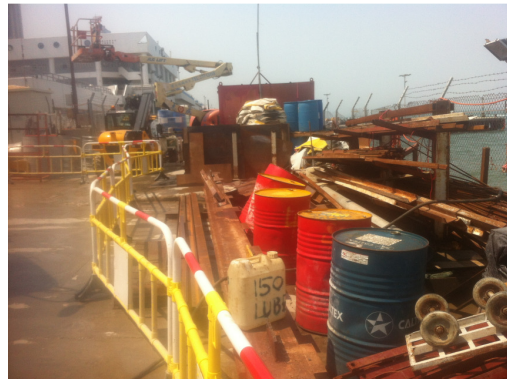
Photo 2 Chemical barrels were found to be without drip trays outside the noise enclosure area
