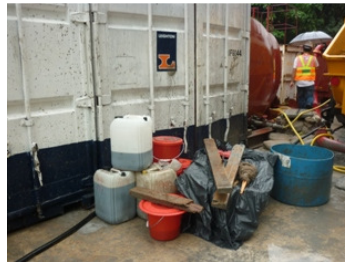
Photo 2 Some unknown chemical drums were found without labels and drip trays
