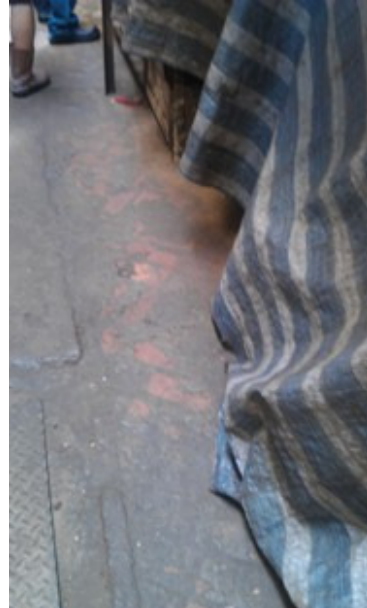
Photo 4 Waste oil near the noise enclosure of the inner entrance was cleared
