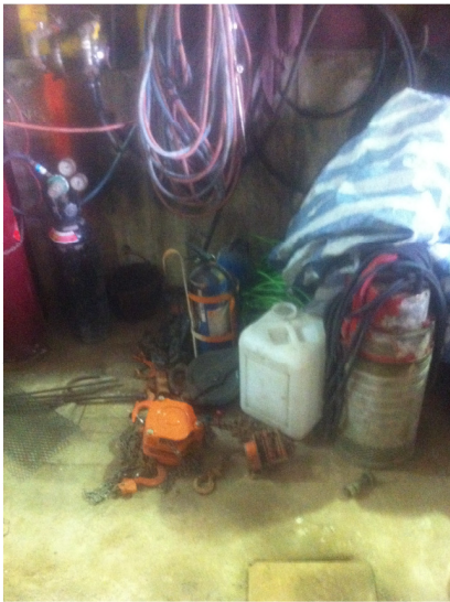
Photo 1 Oil wastes were found within the equipment area inside the noise enclosure.
