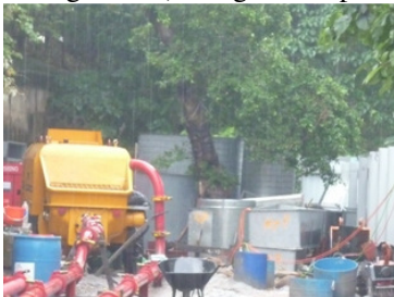
Photo 1 Construction materials were stored too close to the tree (T003 (T)) in Storage area (during last inspection)
