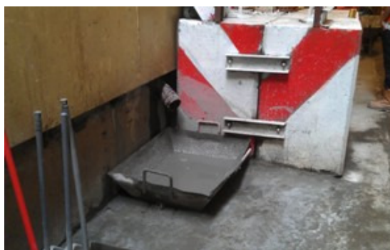
Photo 3 Wastewater from concrete sampling was stored in an unsuitable container. The waste water may overflow during the concrete sampling
