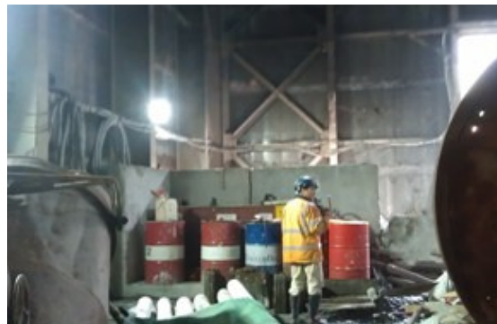
Photo 2 Chemical drums were found without chemical labels and drip trays in the noise enclosure.
