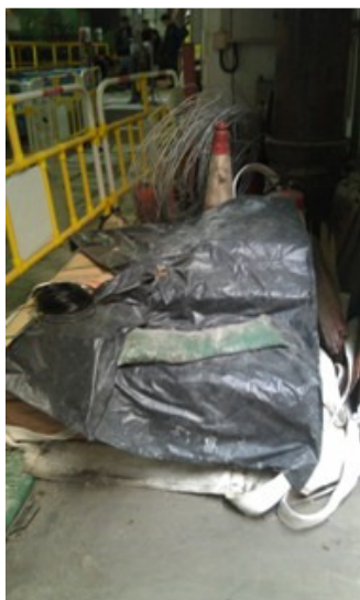
Photo F_1 Cement bags were covered properly.
