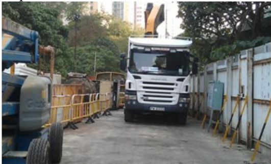
Photo 3 The access was blocked during the site inspection.
