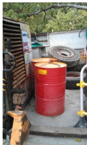
Photo 2 The chemical drums near site entrance were observed without drip trays.
