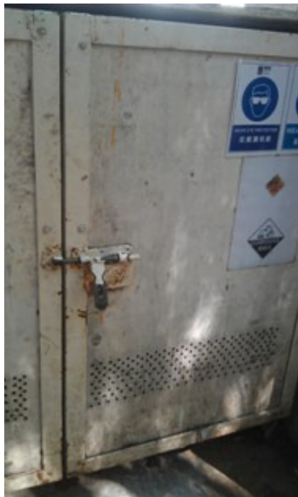
Photo 1 The storage area for rechargeable battery was not locked.
