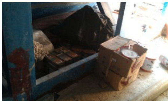
Photo 1 Some chemical drums were found without drip trays under the Aqua. Sedimentation tank
