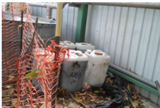
Photo 3 Wastewater from concrete sampling was stored in an unsuitable container. The waste water may overflow during the concrete sampling
