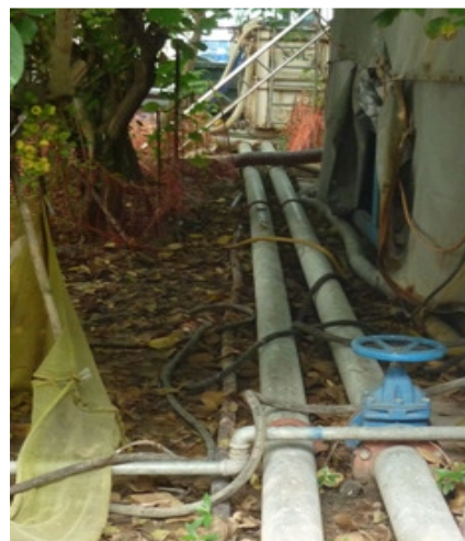
Photo 6 No potential stagnant pools were found behind the sedimentation tank
