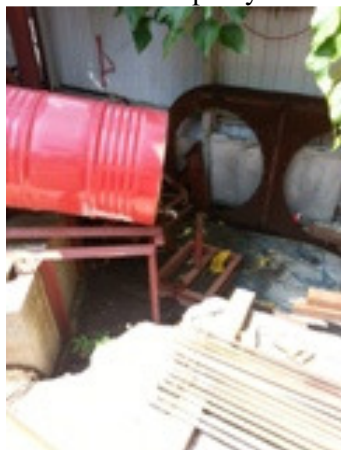
Photo 1 Chemical near the welding zone was found without drip tray
