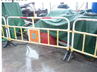
Photo 1 Some chemical containers were found without labels and drip tray near stockpiles
