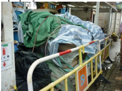
Photo 1 Cement bags were found without properly cover
