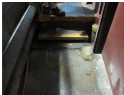
Photo 4 Stagnant pool was found in the noise enclosure
