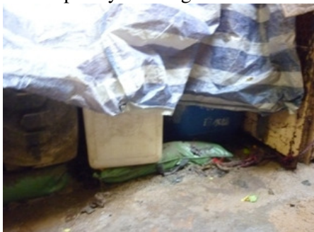
Photo 3 The contractor provided some sand bags for temporary bunding
