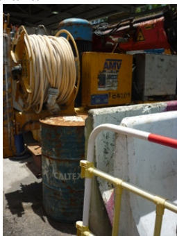
Photo 3 Chemical barrel was found without near the AMV plant.
