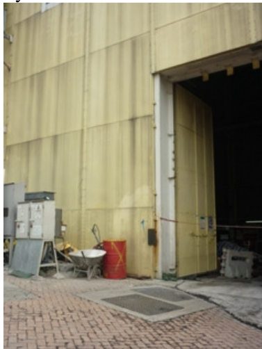
Photo 1 Chemical barrel was found without drip tray near the door of noise enclosure
