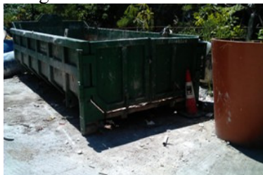
Photos 1 and 2 Trashes were found next to the skip near the gate
