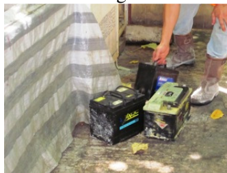
Photo 2 Liquid state battery was stored improperly near the fuel storage area.
