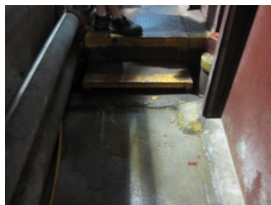
Photo 4 Stagnant pool was found in the noise enclosure
