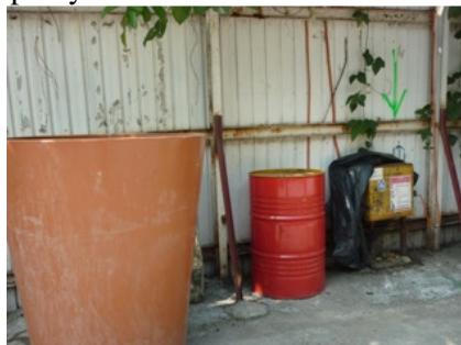
Photo 3 Some chemical barrels were found in workshop without suitable labels and drip tray
