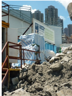
Photo 3 Cement bags were covered properly
