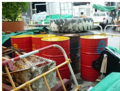
Photo 2 Oil barrels were found without drip trays
