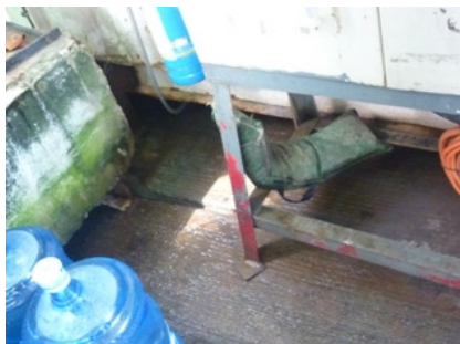
Photos 1 and 2 Dripping from air conditioner was found near material container
