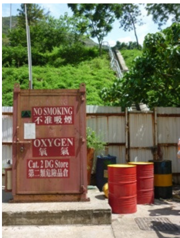
Photo 3 workshop without suitable labels and drip tray
