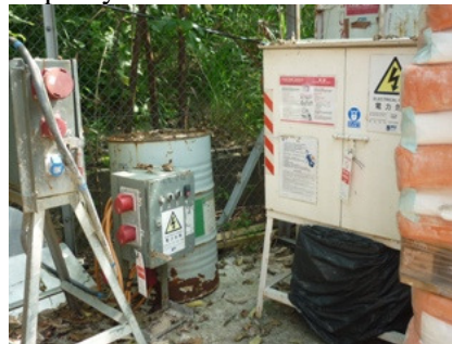
Photo 2 Some chemical barrels were found in the workshop without suitable labels and drip tray
