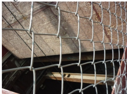
Photo 3 Stagnant water l-beam was cleared
