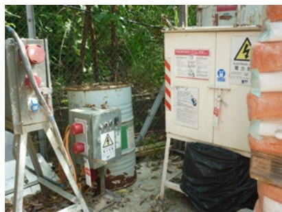
Photo 2 Some chemical barrels were found in workshop without suitable labels and drip tray
