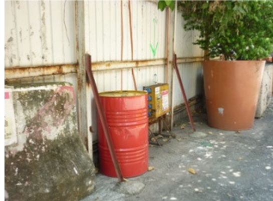
Photo 2 Chemical barrel without drip tray in workshop near electric box on last inspection.
