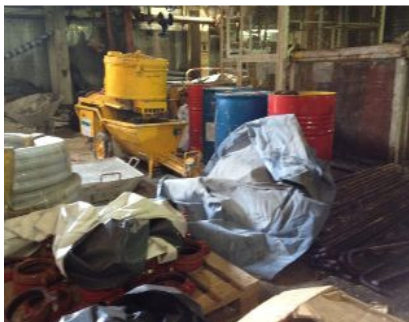
Photo 3 Cement bags had been covered by tarpaulin
