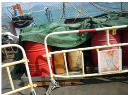
Photo 3 Chemical without suitable labels were found
