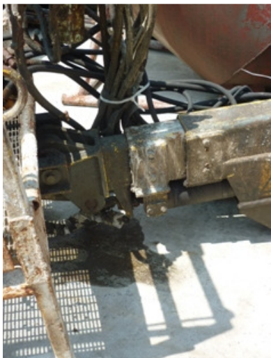
Photo 1 Oil droplets were found near the plants stockpile since last inspection
