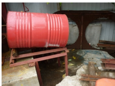
Photo 1 Chemical near welding zone was found without drip tray
