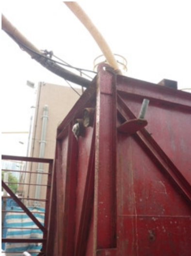
Photo 3 No more leaking was found near the sedimentation tank
