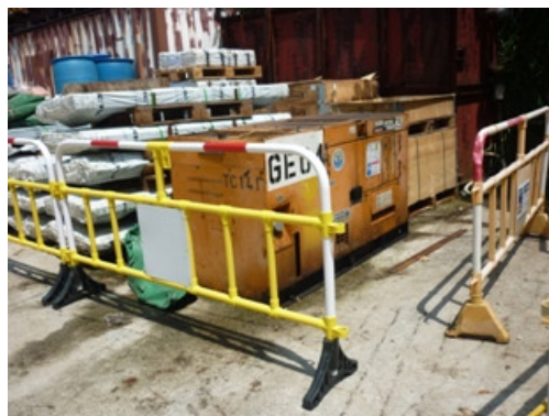
Photo 6 Oil stains were found under the air compressor near stockpiles in workshop
