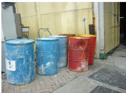
Photo 1 Some chemical barrels were found without drip tray near the door of noise enclosure
