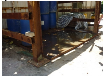
Photo 5 Stagnant water pools were found in the drip tray
