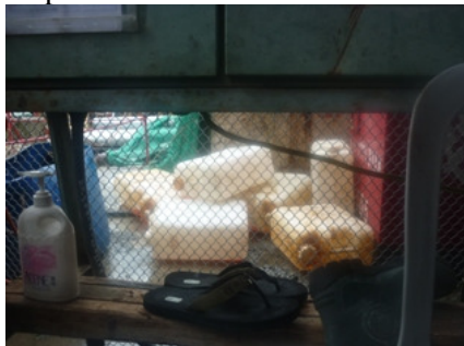
Photo 1 Come chemical drums were found without suitable labels and drip tray next to the air compressor near the mobile crane
