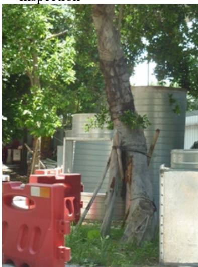
Photo 1 The transplant tree (T003) was found without protective fence since last inspection
