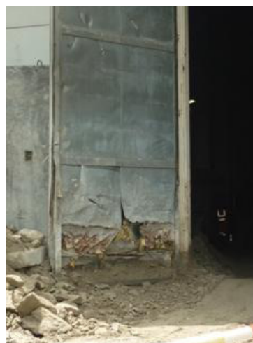
Photo 2 Chemical without suitable labels were found
