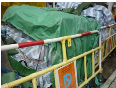
Photo 1 Cement bags were covered properly
