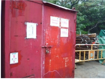
Photos 3 The chemical storage was found without chemical contain list
