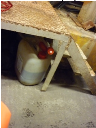
Photo 1 A chemical drum was found without chemical label and drip tray
