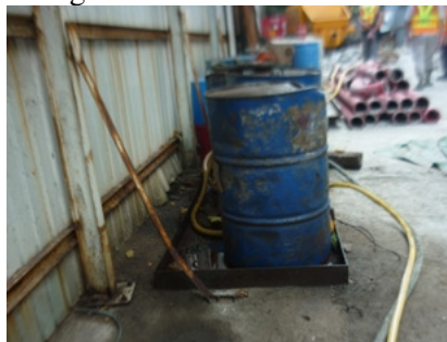
Photo 10 Accumulated of water was found in drip tray of oil barrels near the stockpiles in storage area
