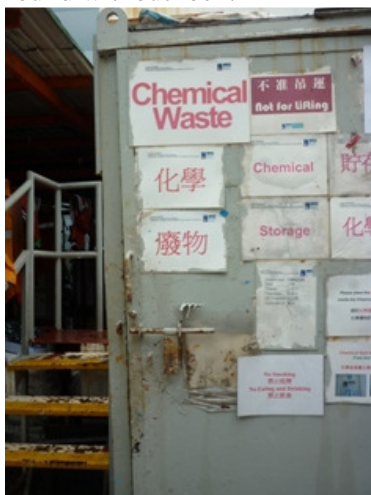
Photo 3 The Chemical Storage container was found without lock.
