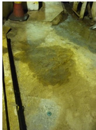
Photo 2 Some sand mix with oil was found in noise enclosure
