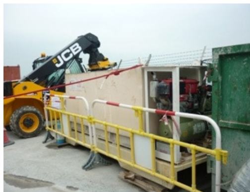
The chemical drum was behind the fuel tank.
