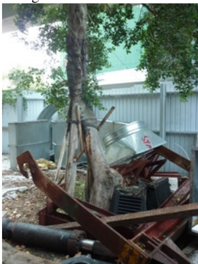
Photo 1 Construction materials were stored too close the tree (T003(T)) in storage area
