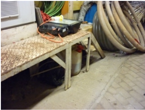
Photo 2 Water accumulation was found near the noise enclosure
