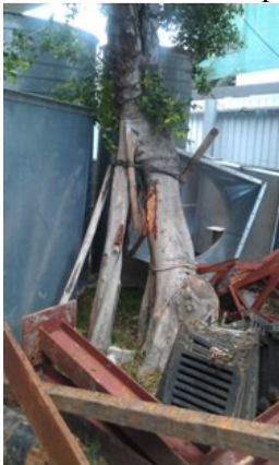
Photos 2 and 3 The items of “Construction materials were stored too close to the tree (T003 (T)) in Storage area” will be follow up in next inspection due to assess road was blocked.
