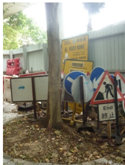
Photo 8 Construction materials were stored too close to the tree (T005 (T)) in storage area.
