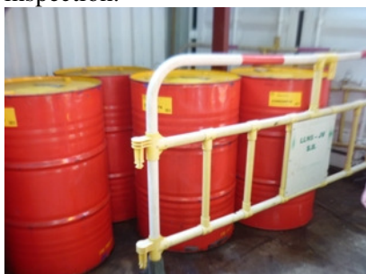
Photo 3 Some chemical barrels were found without drip tray next to chemical storage since last inspection.
