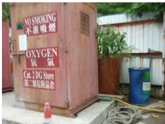
Photo 5 A waste oil barrel was found near the Oxygen container in storage area
