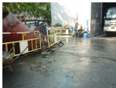
Photo 4 Some oil stains were found next to the stockpiles
