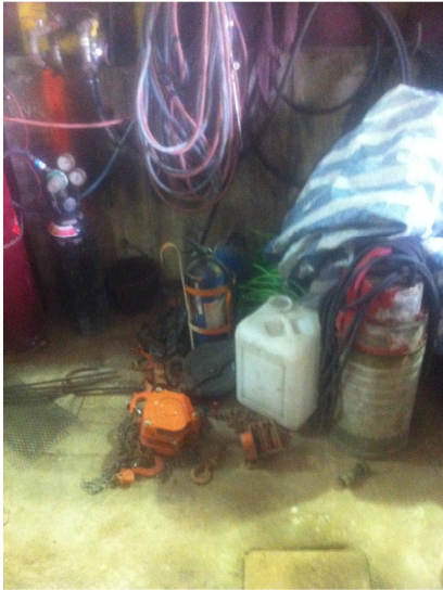
Photo 1 Oil wastes were found within the equipment area inside the noise enclosure.
