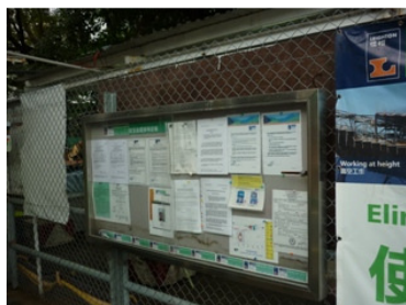
Photo 1 No valid EP was found at entrance.
