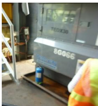
Photo 5 Waste oil was accumulated in drip tray of generator at 1 st platform.
