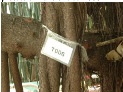
Photo 7 A metal bar was found inside the tree protection zone of tree T006
