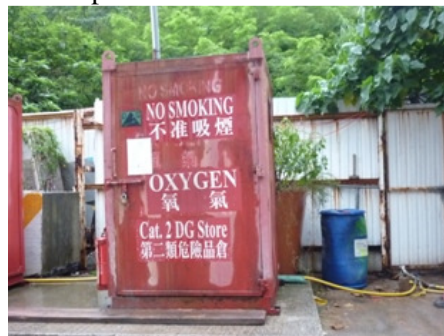
Photo 6 A waste oil barrel was found near the Oxygen Container in storage area since last inspection
