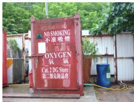
Photo 4 A waste oil barrel was found near the Oxygen Container in storage area since the site inspection undertaken on 13 th November 2012
