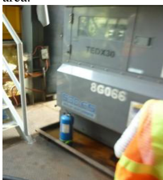
Photos 11 and 12 Waste oil was accumulated in drip tray of generator at 1 st platform and drip tray of generator in storage area.
