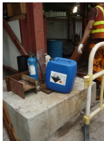
Photos 3 and 4 Some chemical barrels were found without drip tray next to Plants zone and near the site hoarding behind the chemical storage container
