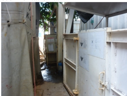
Photo 1 Some water accumulated next to sedimentation tank
