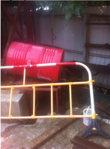
Photo 1 Chemical barrel was found to be without a drip tray.
