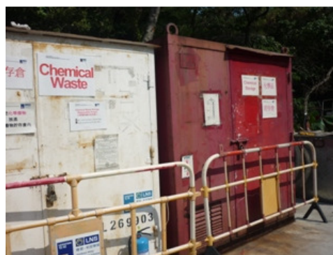
Photo 2 The chemical storage was found without chemical storage list.
