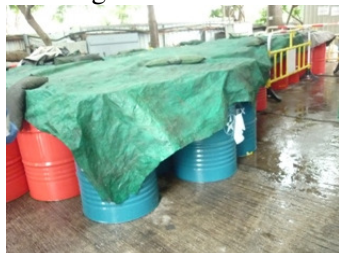
Photo 1 Some chemical barrels were found without drip tray next to chemical storage area and near the site hoarding behind the chemical storage container.
