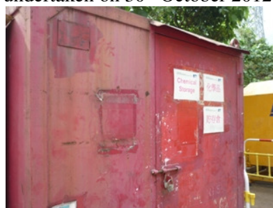
Photo 2 The chemical storage was found without chemical storage list since the site inspection undertaken on 30 th October 2012
