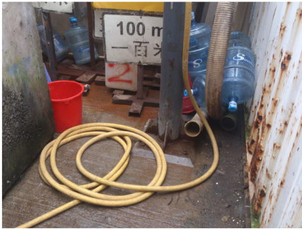
Photo 3 Water accumulation was found in the drip tray next to noise enclosure.
