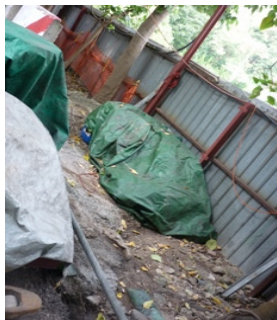
Photo 1 Some chemical barrels were found without drip tray next to chemical storage area and near the site hoarding behind the chemical storage container.
