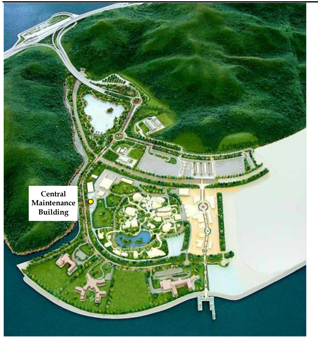
Figure 2.4 NM4 – Rooftop of Central Maintenance Building
