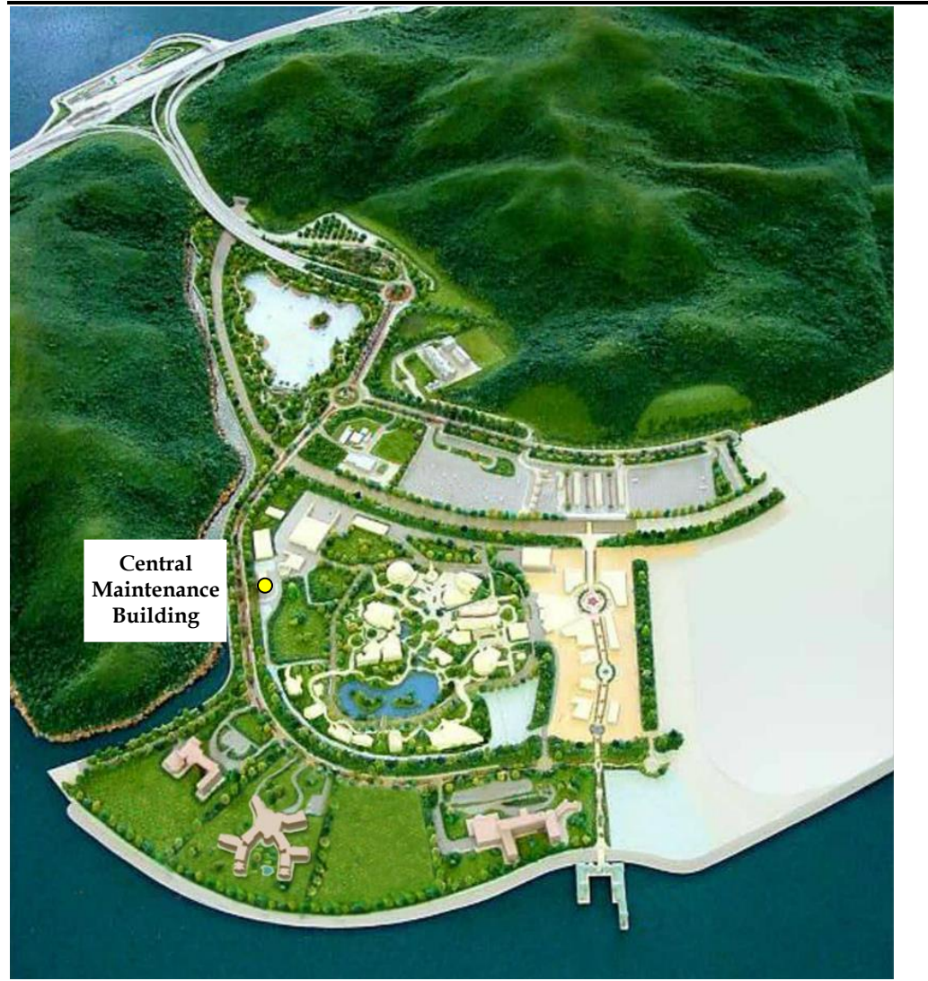
Figure 2.4 NM4 – Rooftop of Central Maintenance Building
