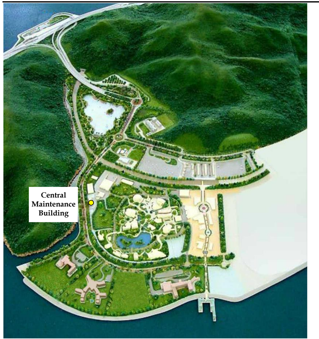
Figure 2.4 NM4 – Rooftop of Central Maintenance Building
