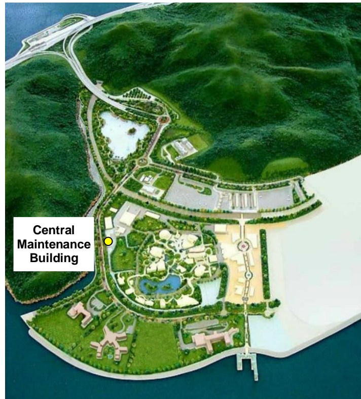
Figure 2-4 NM4 – Rooftop of Central Maintenance Building
