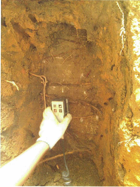
Cover-meter scanning for checking of reinforcement
