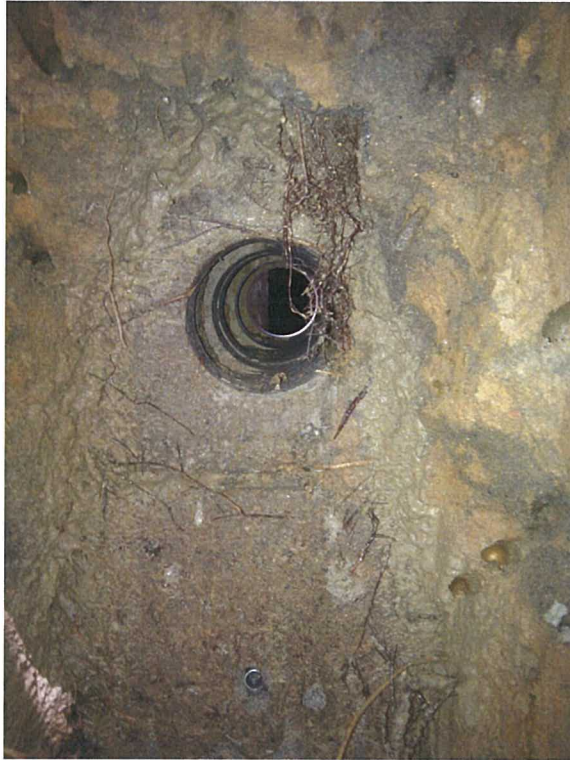
Thickness of wing wall measured through the core-hole is 665mm
