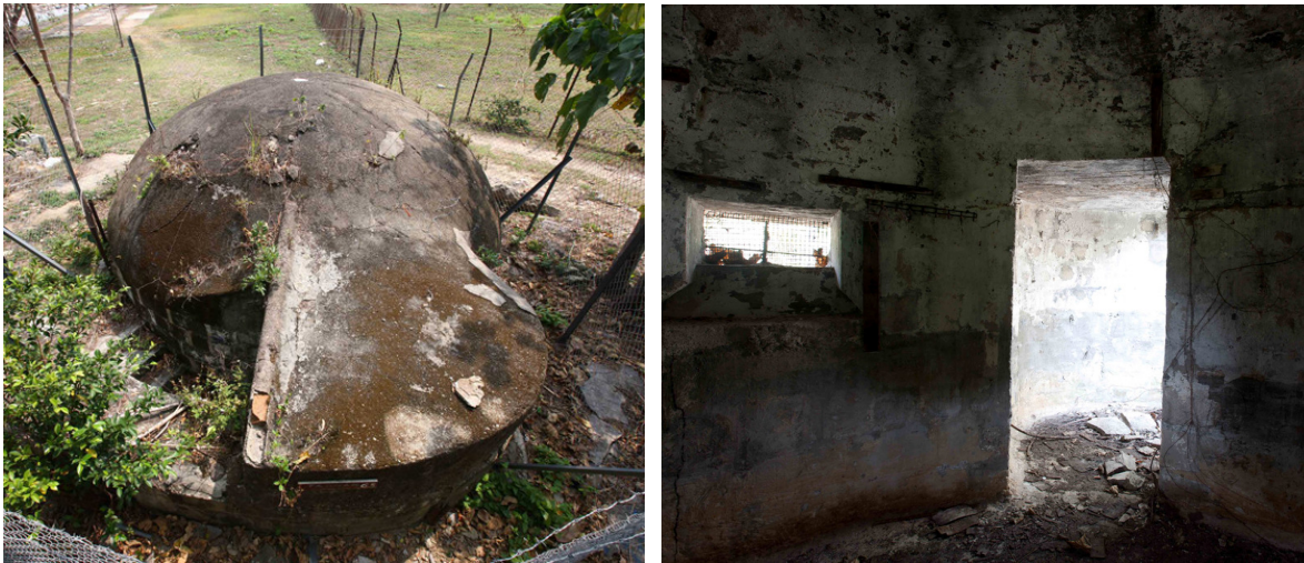
Photo 3.1 & 3.2 The above photos show the outlook and entrance of the pillbox.
