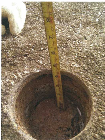
Rebar was encountered at 110mm
