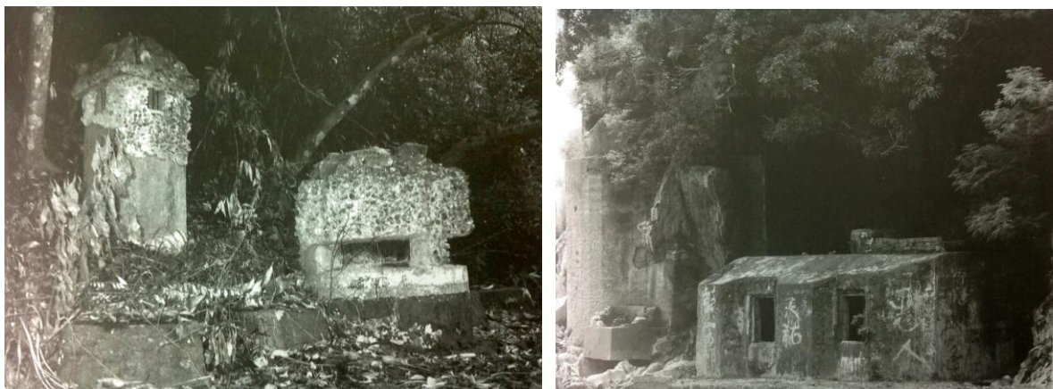
The common rectangular shape Pillboxes built by British Army before WWII in Tai Tam Gap (left) and Waterfall Bay (right).
