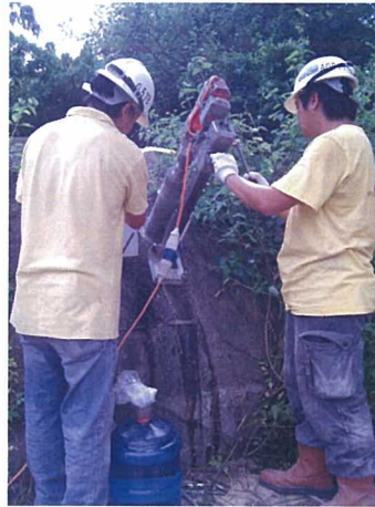
Core drilling
