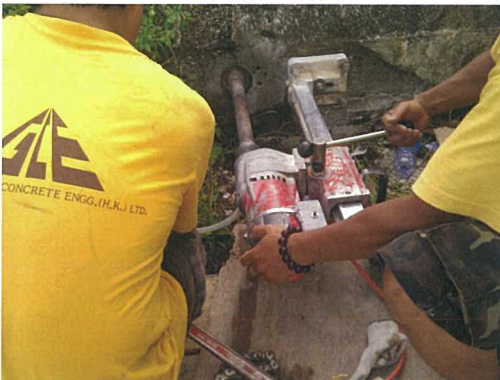
Core Drilling
