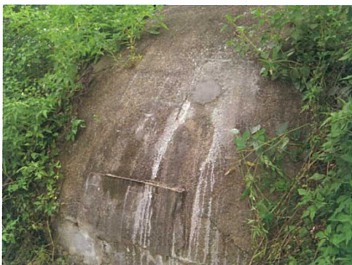
Core-hole and bolt hole were reinstated
