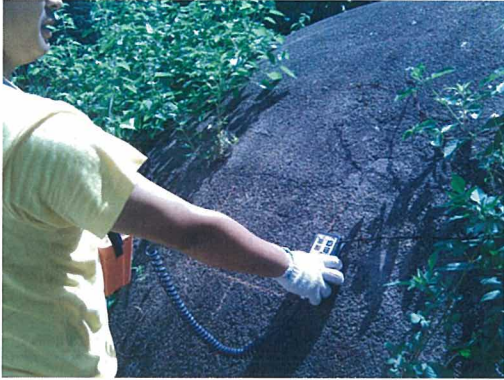
Cover-meter scanning at roof dome, R1
