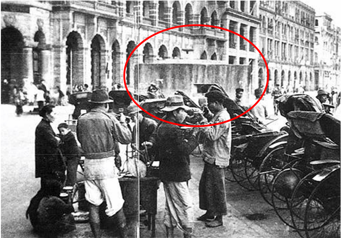
Photo 4.1 (top) & 4.2 (bottom) Photos from after 1941 show other pillboxes located at Hennessy Road Wan Chai and Central.
