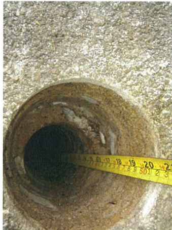
Thickness of roof dome is 515mm
