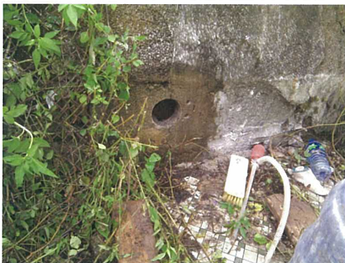
Thickness of wing wall measured through the core-hole is 730mm
