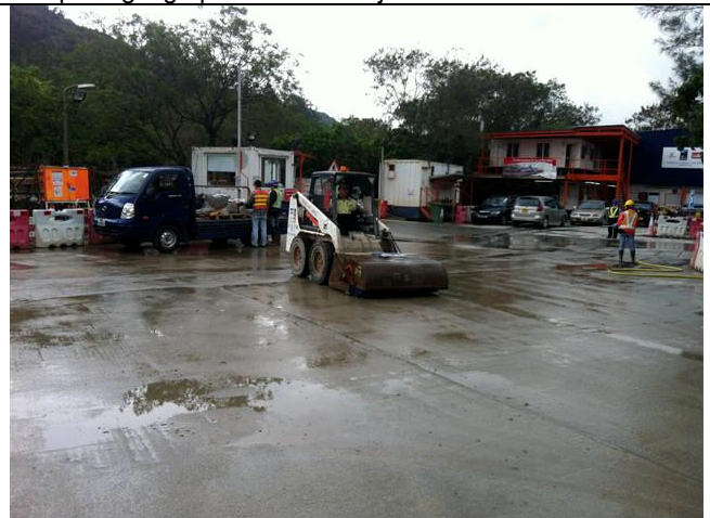
Photo 6. The floor area of the site exit point had been paved.
